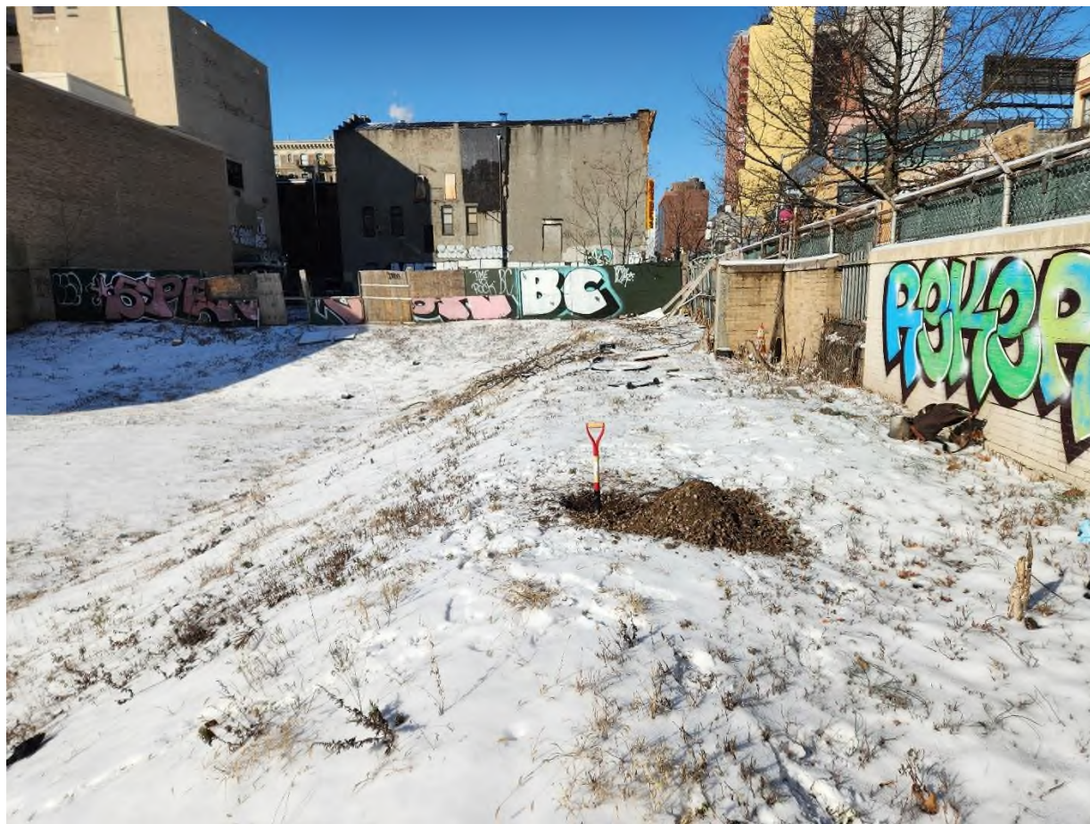
Photo 13: Temporary cover system with Test Pit to confirm RCA depth, facing west toward Madison Avenue (January 17, 2024)
