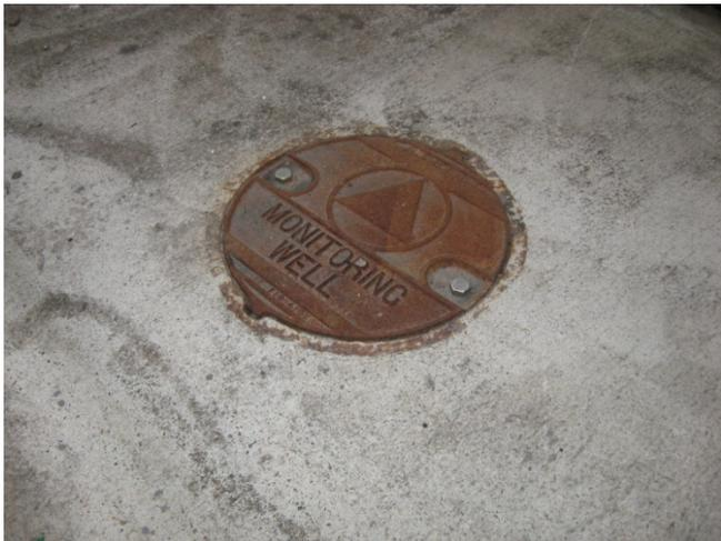
Photo #3 – View of well M-8 (representative of other site monitoring wells)..
