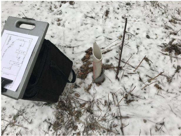
Photo #5 – View of damaged well M-10C.
