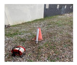
Photo 4: View of well M-10C showing repaired casing.
