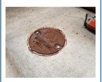
Photo 3: Typical monitoring well in active area of the Site.
