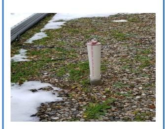
Photo 4: Well M-10C remains intact with repaired casing.
