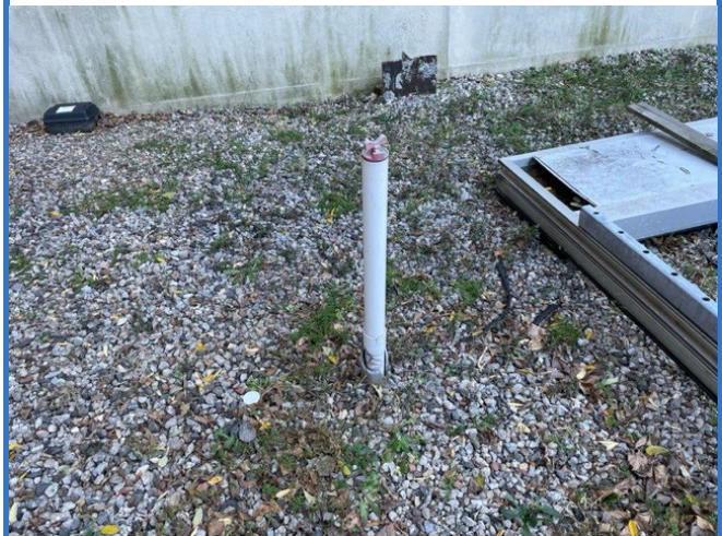
Photo 4: Well M-10C remains intact with repaired casing.
