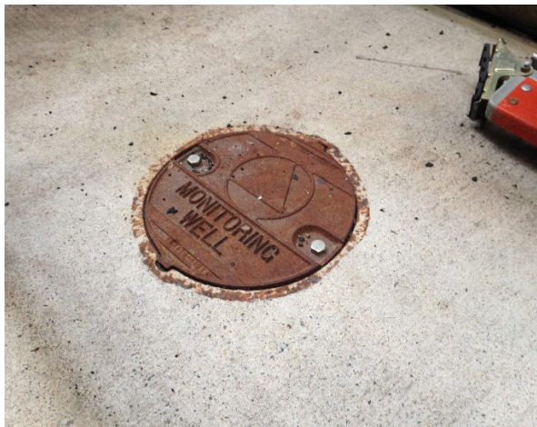
Photo 3: Typical monitoring well in active area of the Site.
