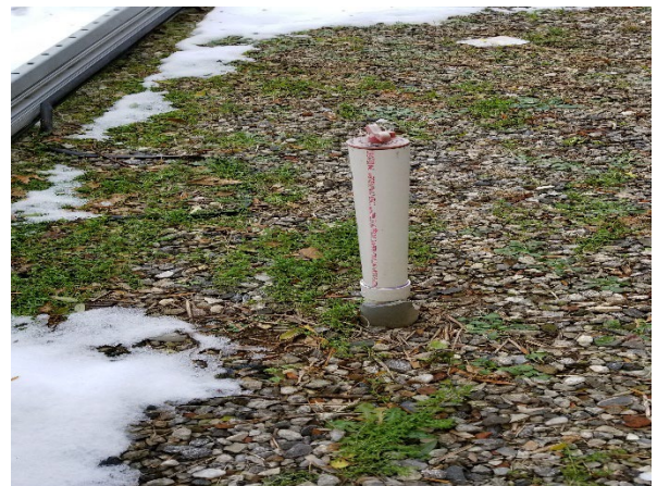
Photo 4: Well M-10C remains intact with repaired casing.
