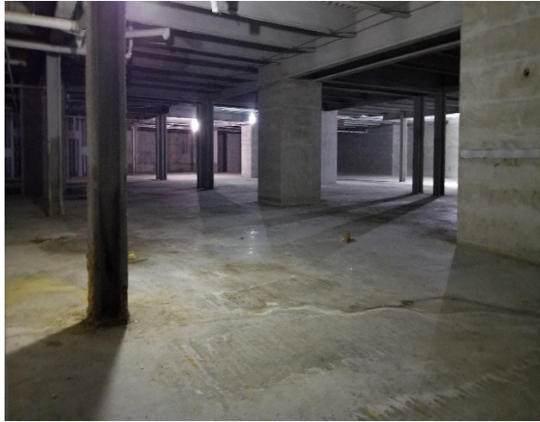
Photo 1: View of basement-level building interior (vacant at this time) showing cover system in place.
