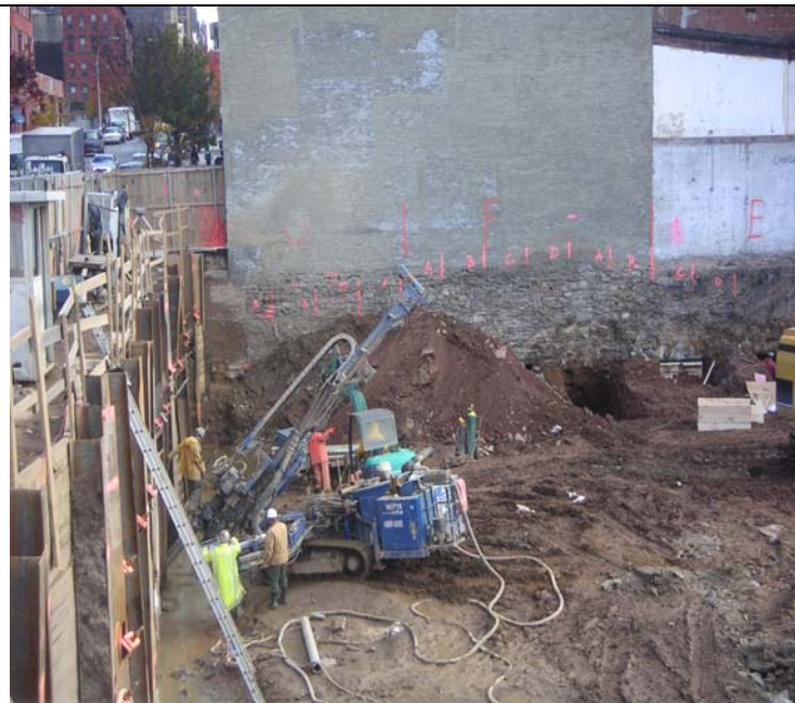
Photo 20: Installation of second row of tie-backs along northern border (35 th Street).
