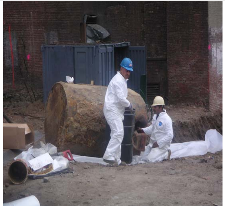
Photo 6: Decommissioning of USTs uncovered near southern gate
