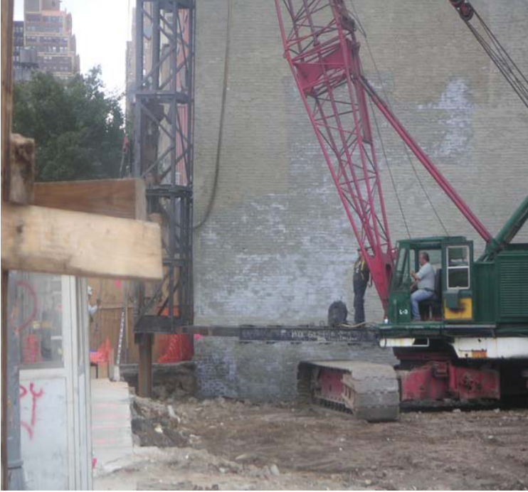
Photo 1: Installation of soldier beam in northeast.
