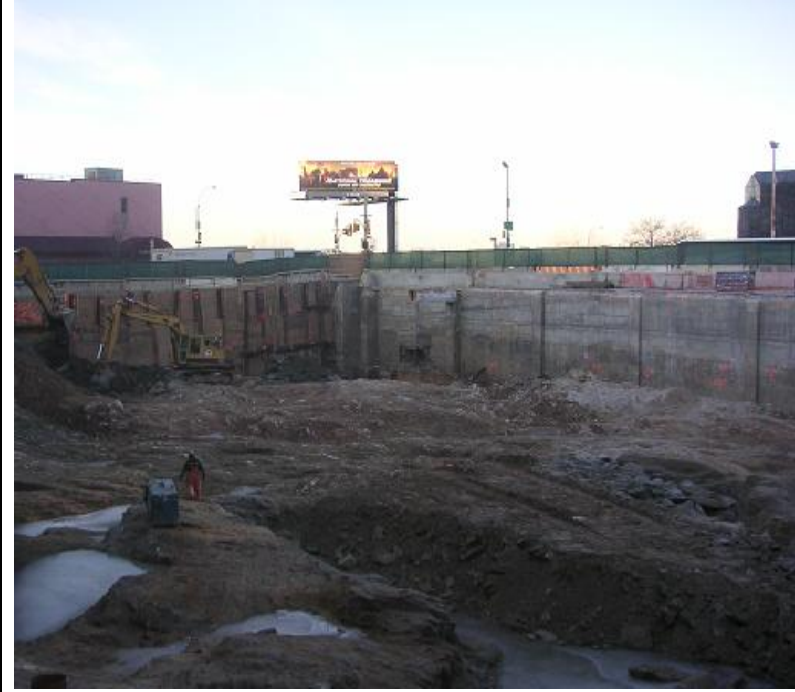
Summary photo of site from northeast to southwest
