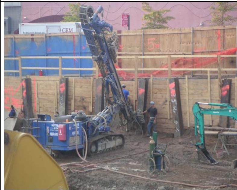
Photo 15: Replacement drill rig continuing drilling tie-backs along southern border (34 th Street).
