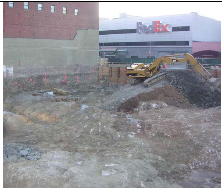
Summary photo overlooking site from northwest to southeast
