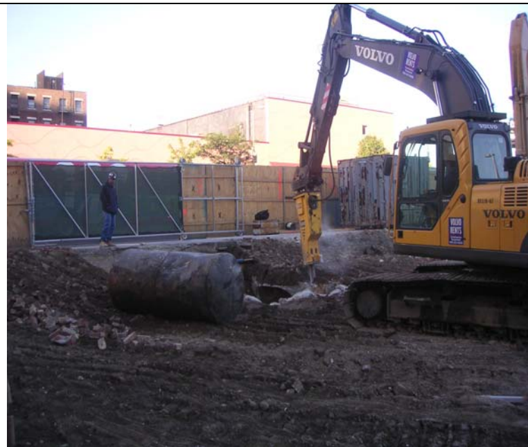
Photo 4: Removal of USTs near southern gate.
