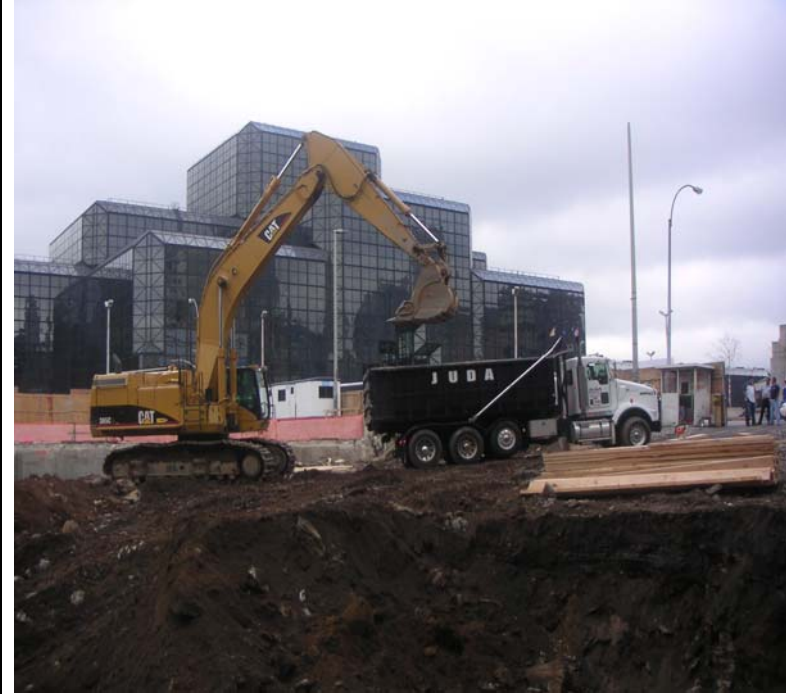
Photo 13: Trucking out of excavated materials.
