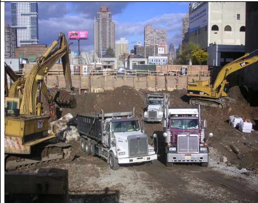
Photo 19: Excavation of material. Photo taken facing down the secondary ramp.
