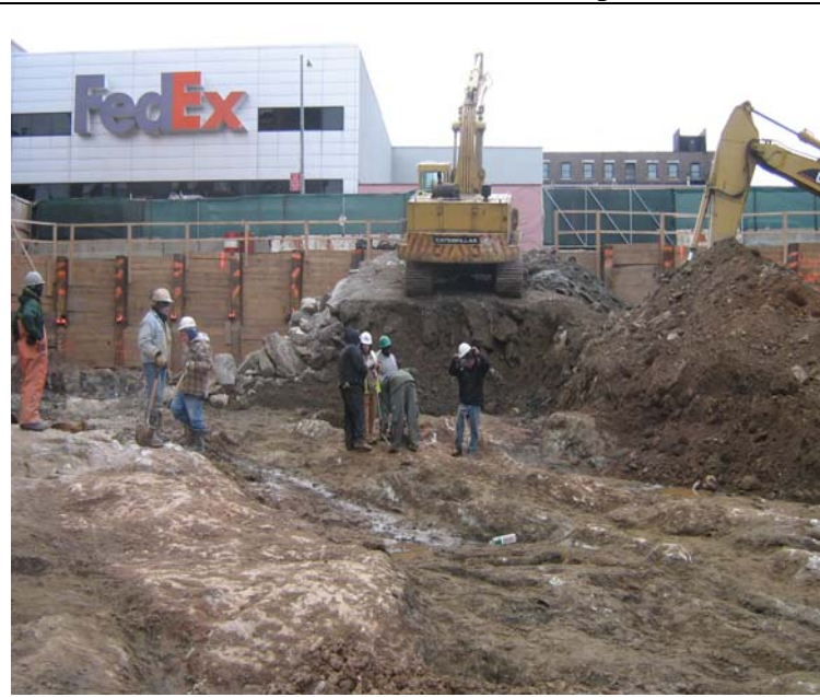
Photo 24: Excavation of area at base of the secondary ramp.
