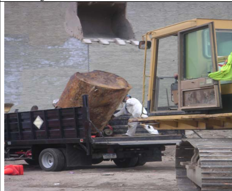
Photo 5: Broken concrete vault that housed three USTs near southern gate.
