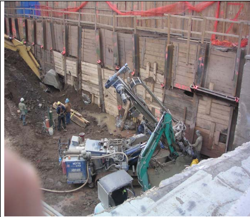
Photo 17: Installation of timber lagging and drilling of tie-backs in southwest corner.
