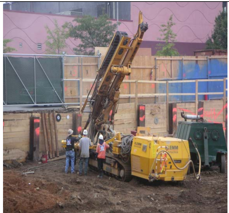
Photo 12: Begin drilling first row of tiebacks along southern border (34 th Street).
