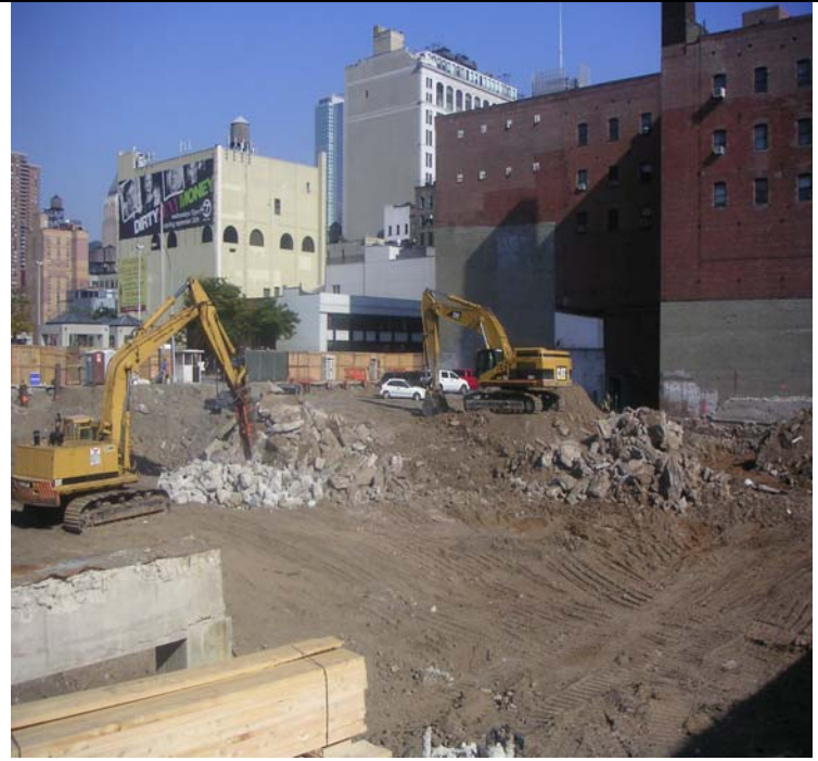
Photo 10: Excavation facing northeast.
