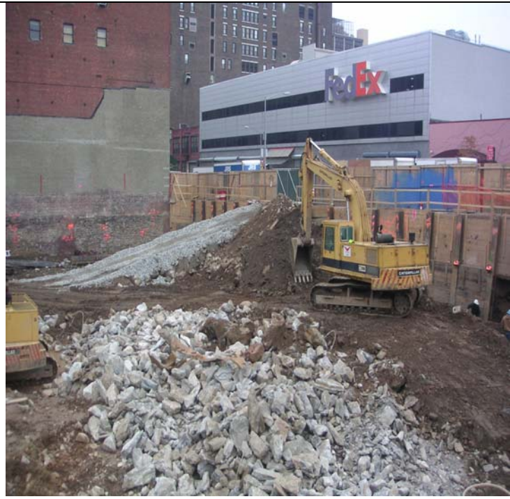
Photo 18: Secondary Ramp on 34 th Street.
