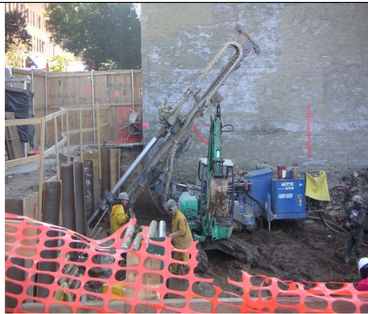
Photo 16: Begin drilling tie-backs in northeast corner.
