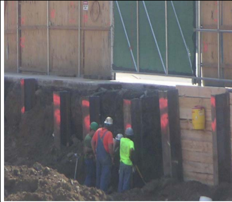
Photo 9: Installation of soldier beams and lagging along southern border (34 th Street).
