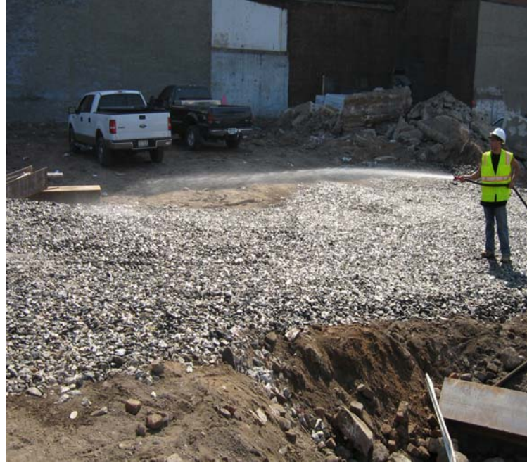
Photo 2: Truck wash ramp at the 35 th Street exit.
