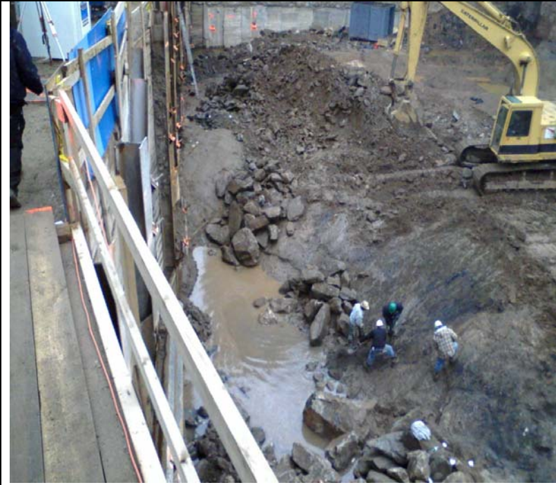
G-1 through G-5 (some bedrock fill)
