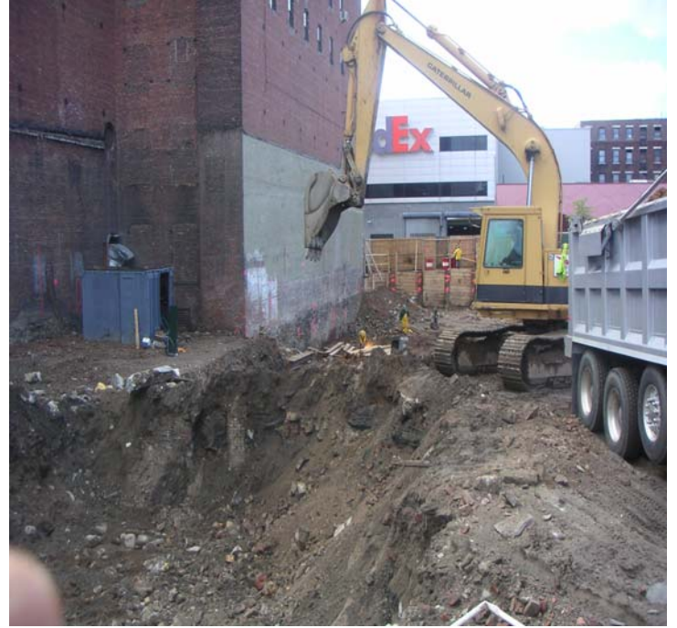
Photo 14: Excavation near adjoining lot (Lot 55) in the northeast corner.
