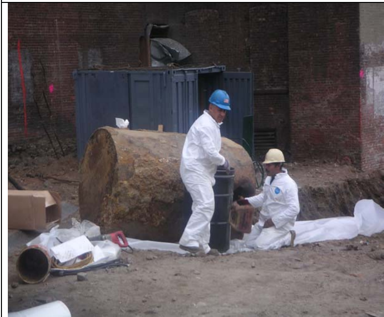
Photo 3: View of underground storage tank cleaning.
