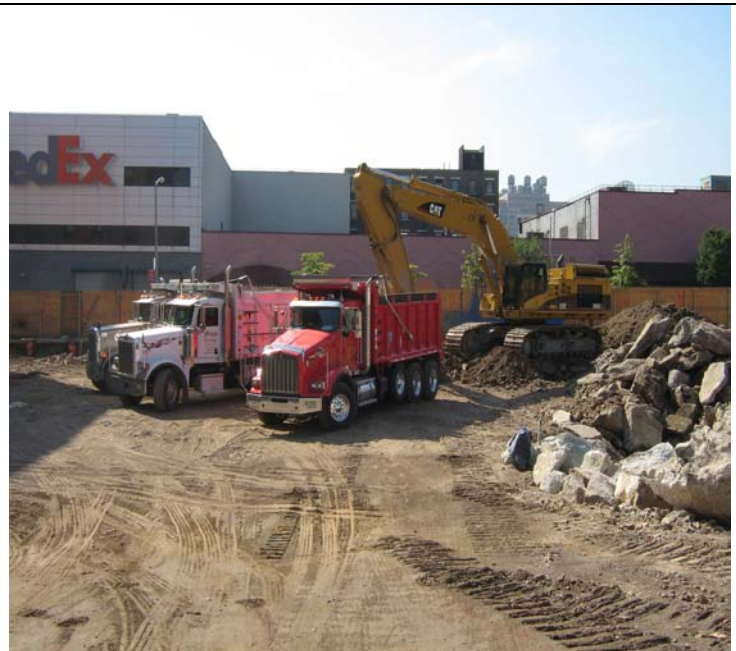
Photo 4: Truck loading of soil for off-site disposal.
