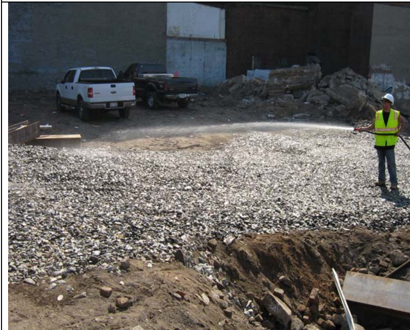
Photo 3: Truck wash ramp at the 35 th Street exit.
