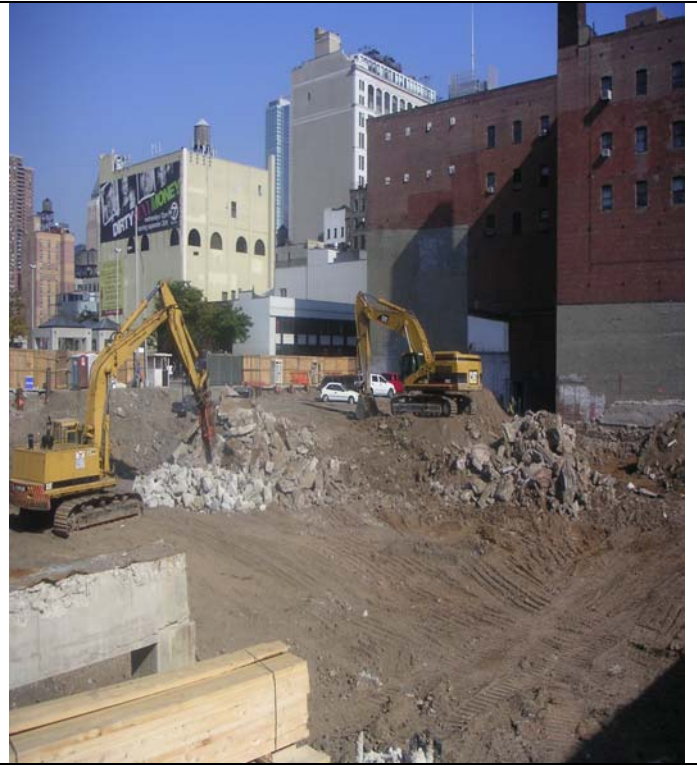
Photo 6: Leveling site grade to at least 3 feet below surrounding grade
