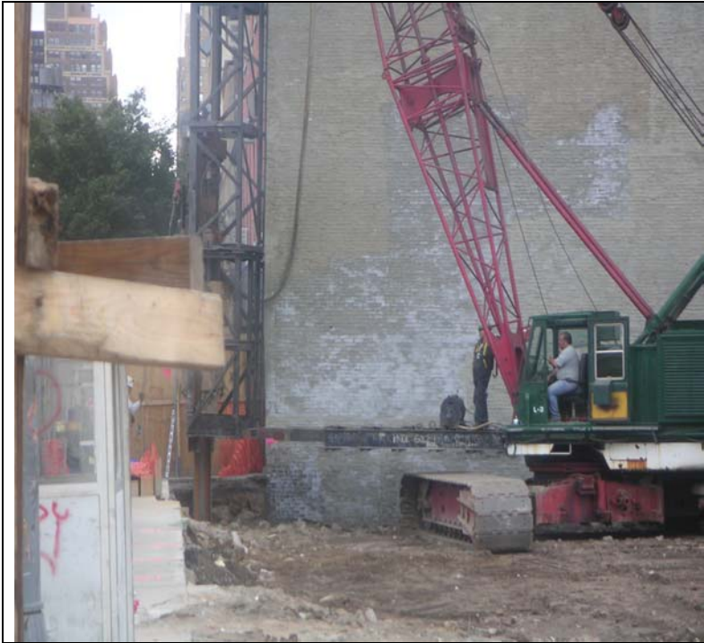
Photo 1: Installation of soldier beam in northeast.
