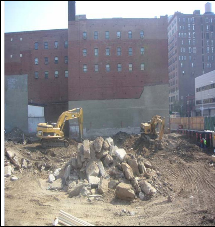
Photo 5: Stockpiling of concrete building slab and foundations
