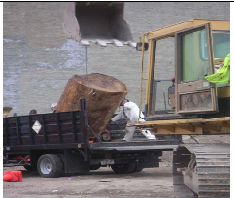
Photo 4: Underground storage tank removal.
