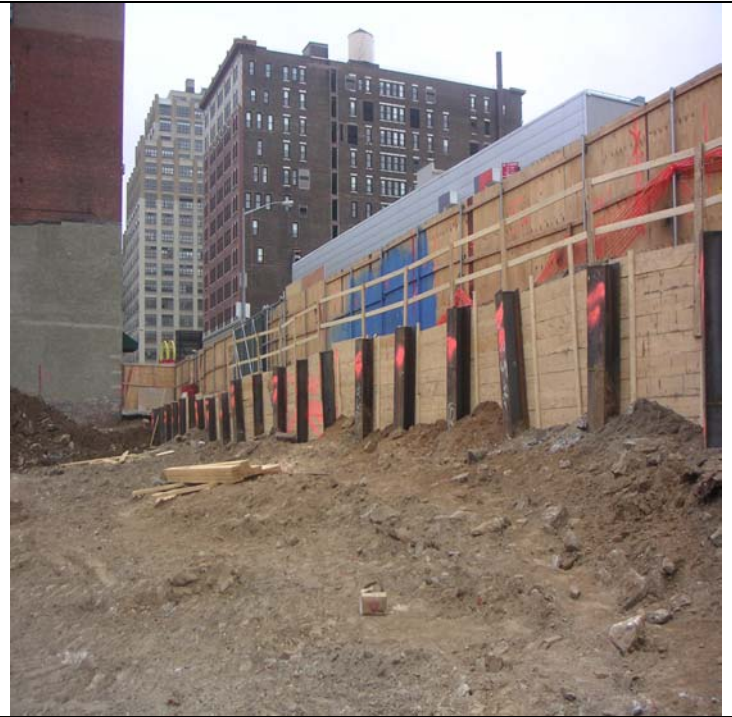
Photo 2: Lagging and sheeting along the southern wall (34 th Street).
