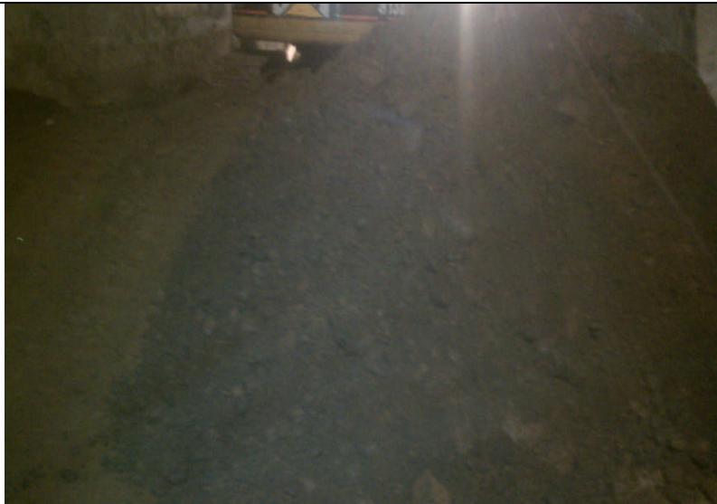
1. Pier #10 excavated to bedrock.
