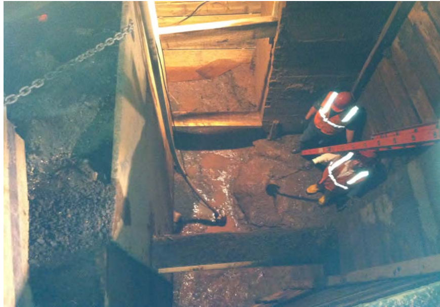
1. Phase II area excavated and cleaned to bedrock.
