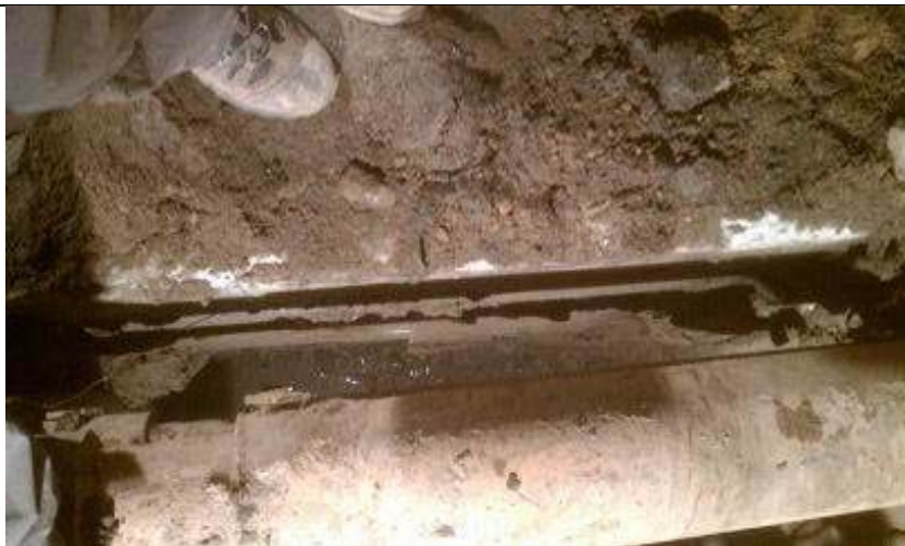
1. Saturated wood sheeting taken during excavation of Pier #13. Slight to moderate odors.
