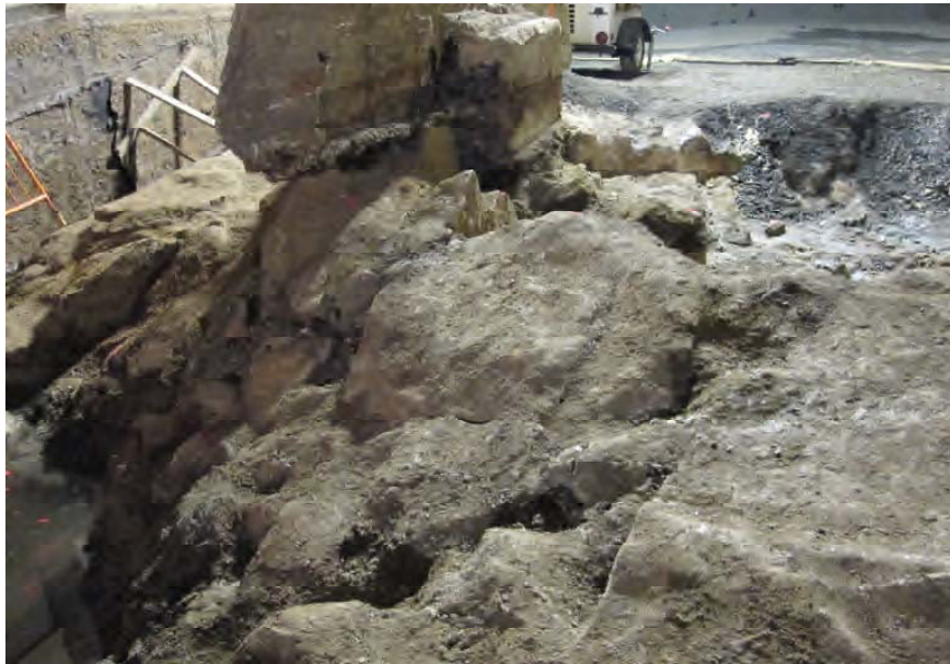
2. North side of Phase II, excavated to bedrock. Inspected and certified by FLS.
