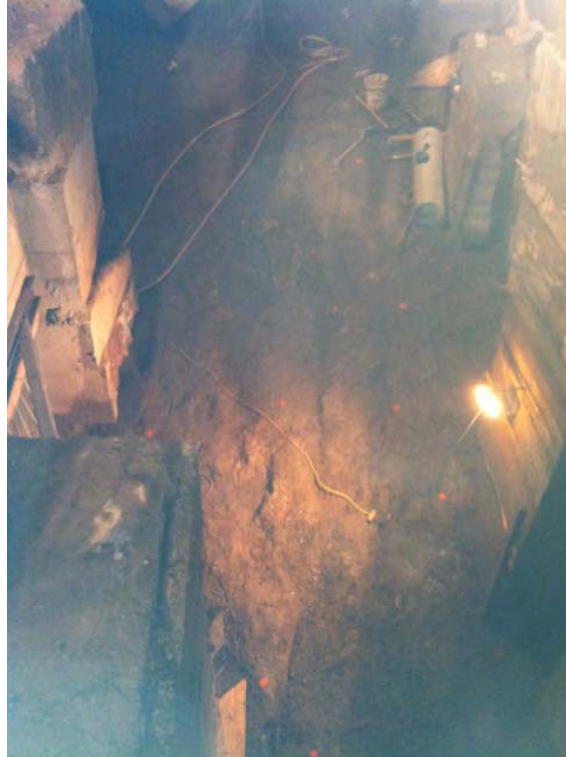
1. Phase II area excavated and cleaned to bedrock.
