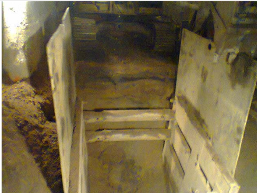
2. Trench boxes and frames were used for the Pier's mold prior to concrete installation.
