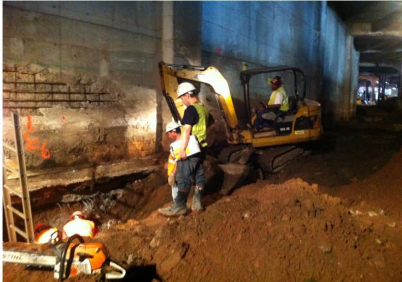
1. Excavation activities being performed via mini excavator.
