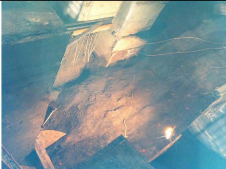
2. Phase II area excavated and cleaned to bedrock.
