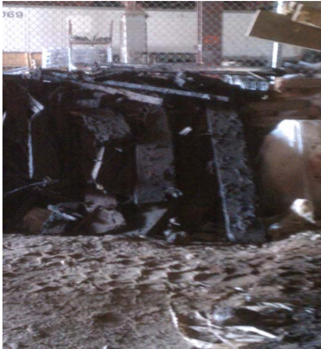
1. Saturated wood sheeting taken during excavation of Pier #13. Slight to moderate odors.
