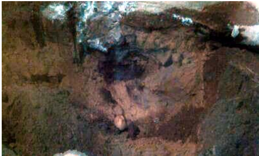
2. Impacted soils at pier # 10 with moderate odors
