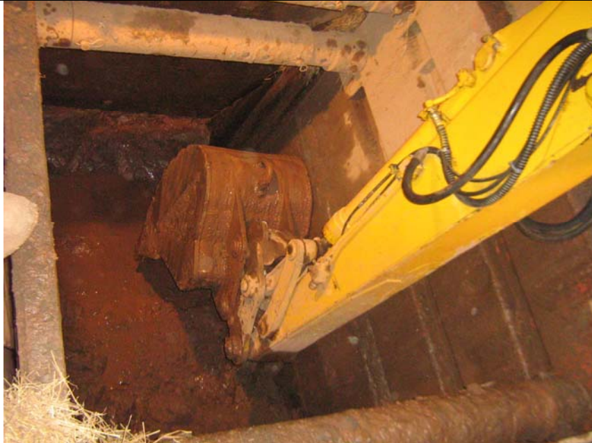
2. Pier #2 Continued excavation of Pier #11 (eventually halted to re-shore excavation and dewater)
