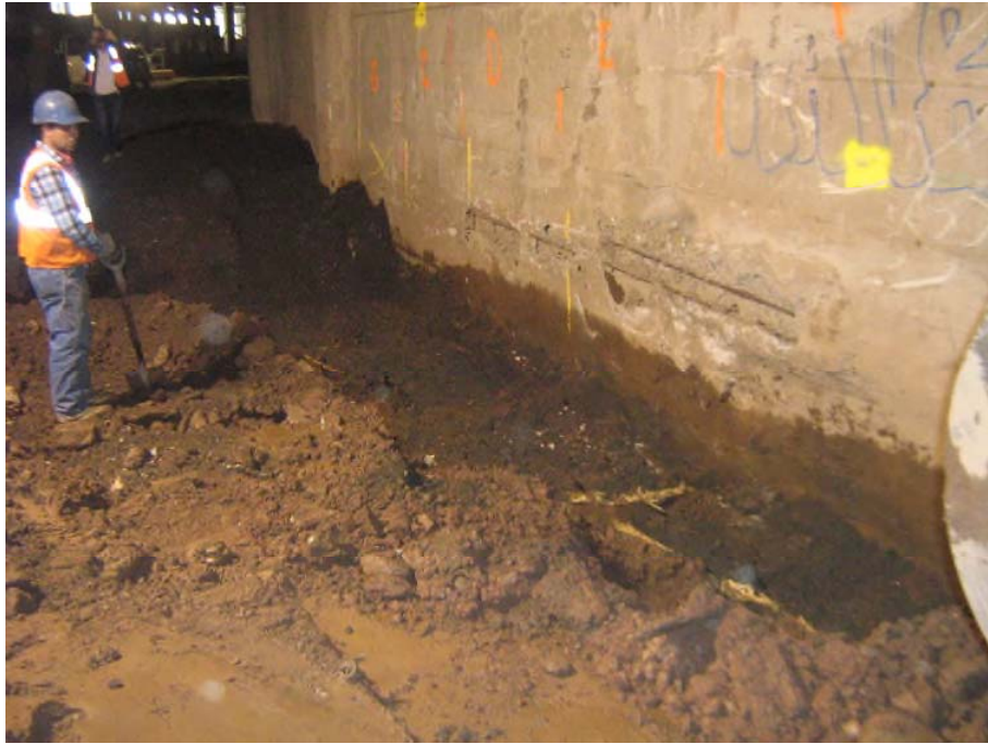
1. Excavation to clean backfill in Phase III and removal of plastic sheeting liner protecting backfill.
