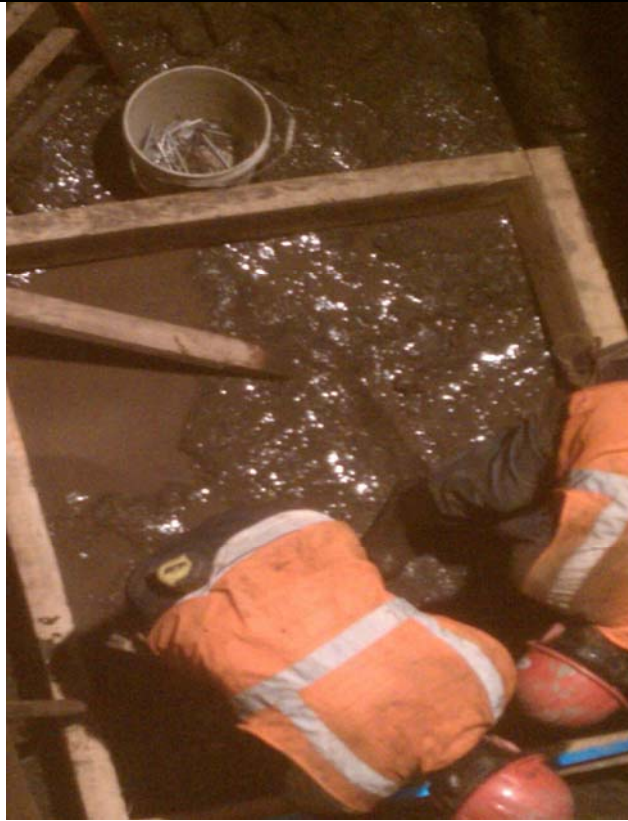
3. Pier #13 excavated down to bedrock.
