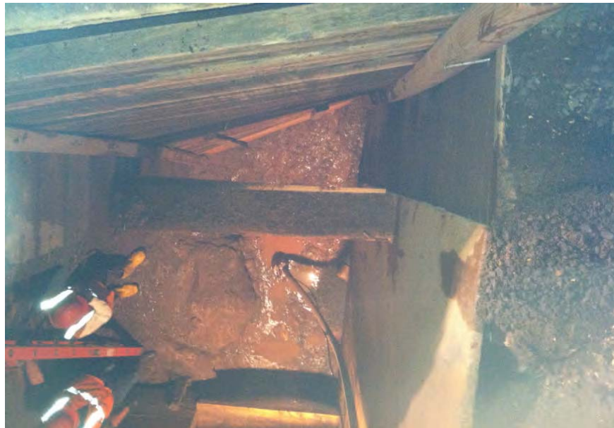
2. Phase II area excavated and cleaned to bedrock.
