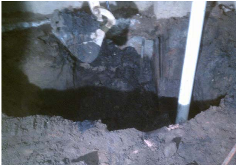
2. Dark soils encountered at Pier #9.
