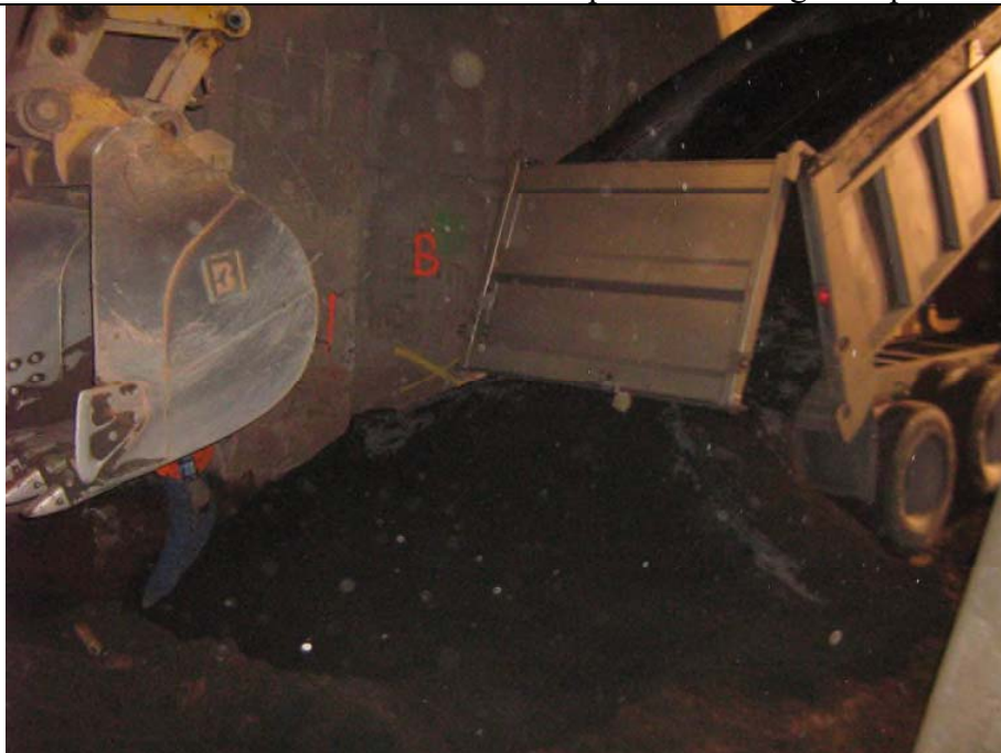
2. Backfilling Phase III area to grade.
