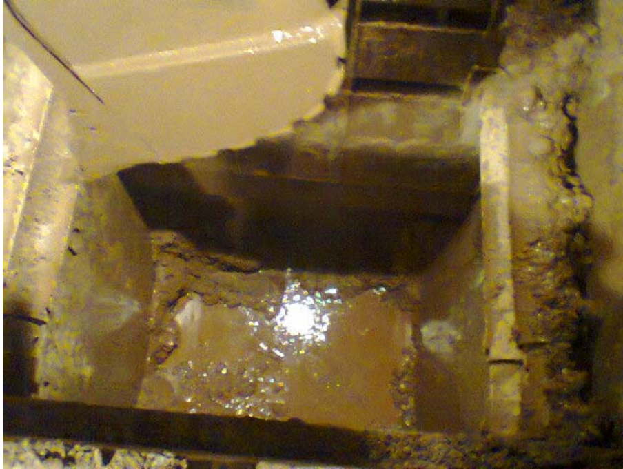
1. Pier # 12 Exposed bedrock.
