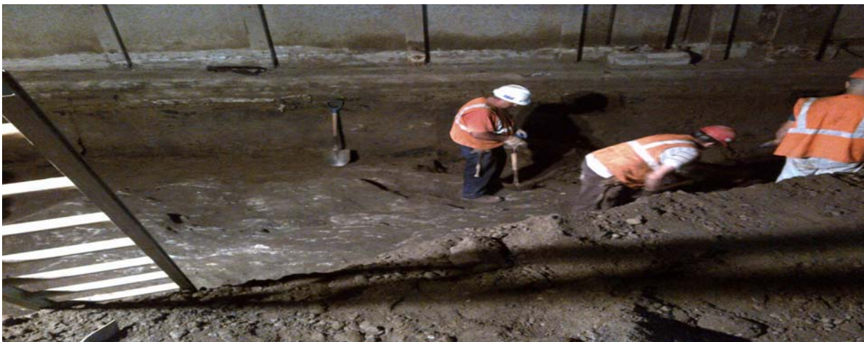
2. Phase 4 Excavation at Bedrock.
