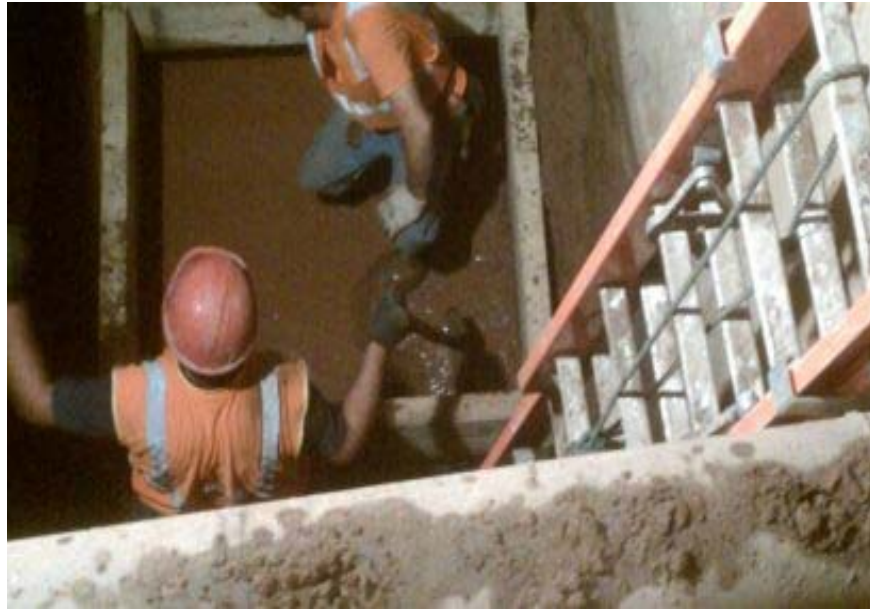
1. Pier #14 excavated to bedrock
