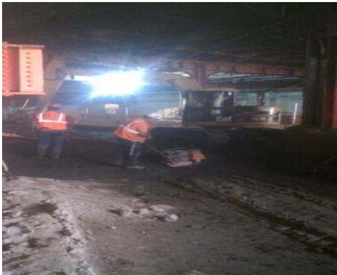
2. Phase 4 backfilled and being compacted at finished grade.
