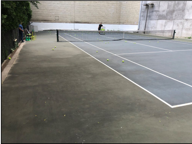
Photograph 5: Tennis court (paved element of the composite cover system.)
