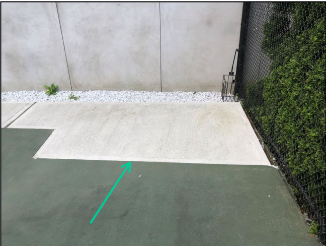
Photograph 7: The southwestern corner of the tennis court, with new concrete pavement installed as part of crack repair.
