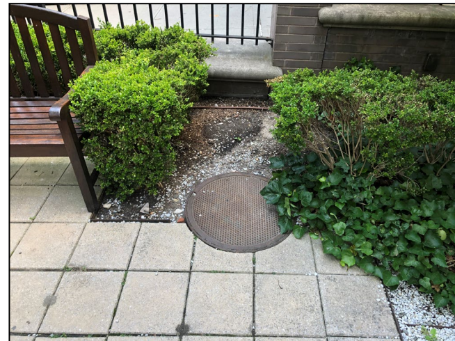
Photograph 4: No soil erosion noted around utilities protruding through the site cover.
