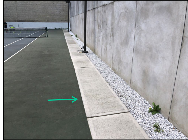
Photograph 8: The southern edge of the tennis court, with new concrete pavement installed as part of crack repair.
