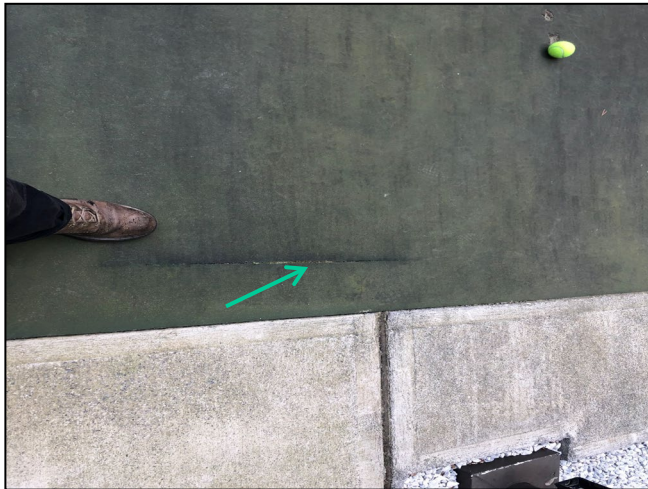
Photograph 9: A new crack along the southern edge of the court (to be repaired).
