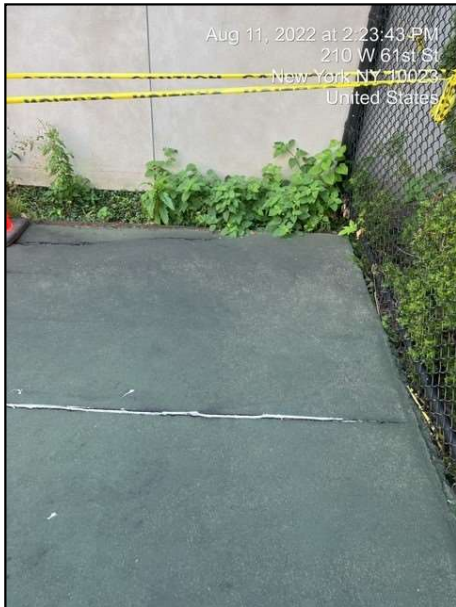
Photograph 7: An approximately 6-foot long crack in the southwestern corner of the tennis court, repaired with grout.
