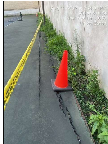
Photograph 8: Cracks, repaired with grout and asphalt, at the southern edge of the tennis court.
