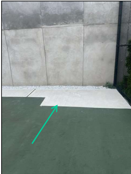
Photograph 7: The southwestern corner of the tennis court, with new concrete pavement installed as part of crack repair.
