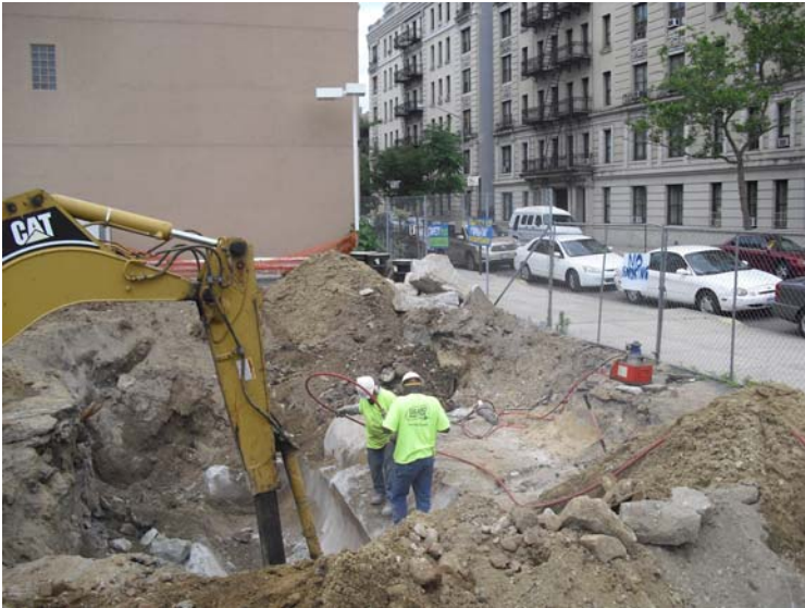
Photo 4 – 4k tanks in concrete
