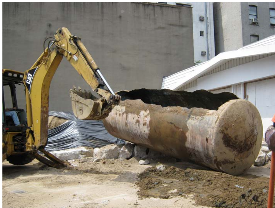
4,000 Gallon UST Removals
