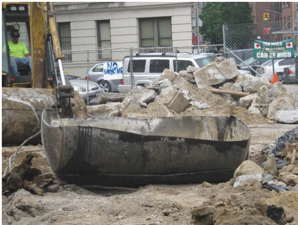
550 Gallon UST Removals
