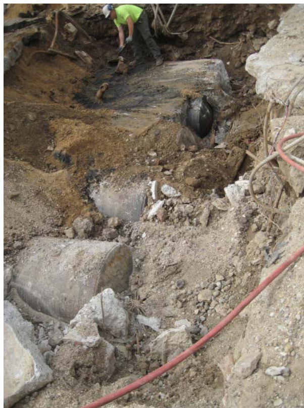
550 Gallon UST Removals
