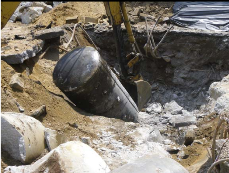
Photo 10 - 550 tank Photo 10 – 550 tank
