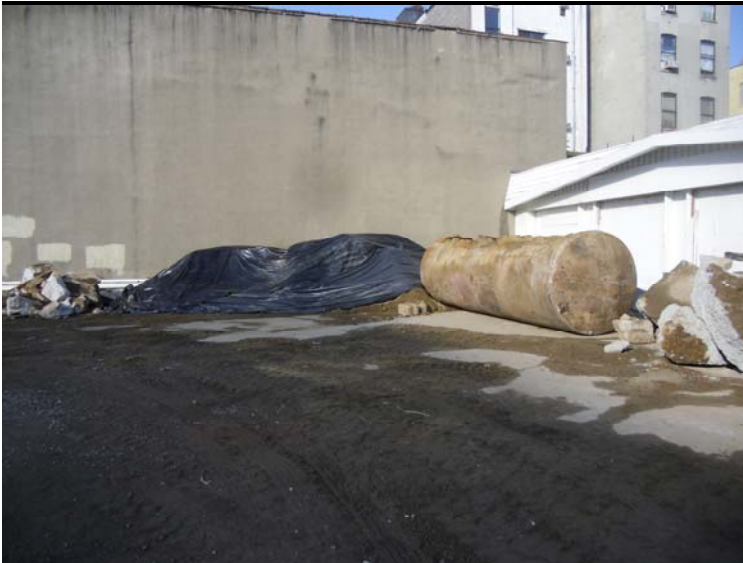
Photo 7 - 4k tank and stockpiled soil
