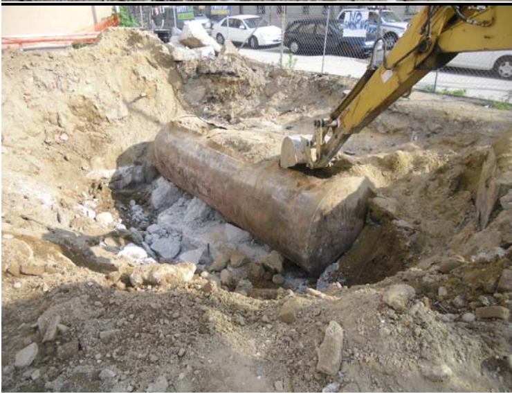
Photo 5 – 4k tank being removed
