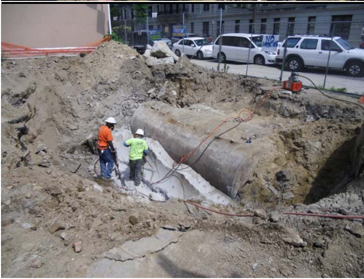
Photo 3 – 4k tank concrete cradle
