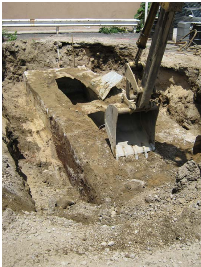
4,000 Gallon UST Removals
