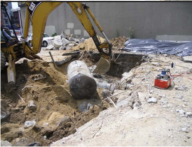
Photo 11 – 550 tank removal
