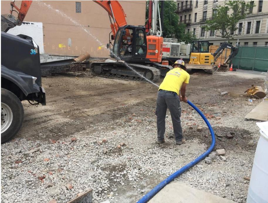
Photo 7: View of Moncon spraying water to prevent offsite dust migration, facing northwest (6/15/2018)
