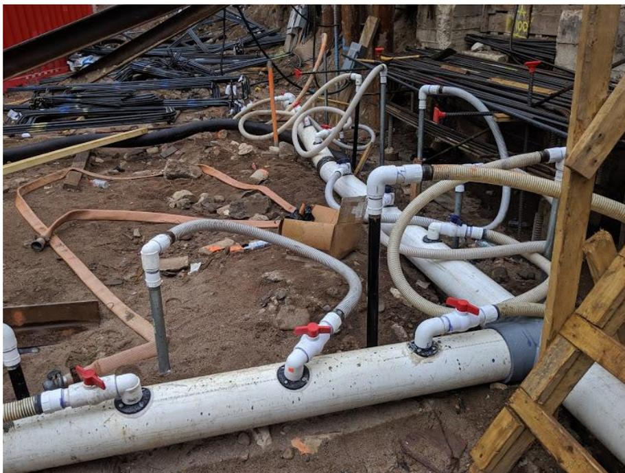
Photo 36: View of dewatering system in Grid 2, facing north (7/5/2019)
