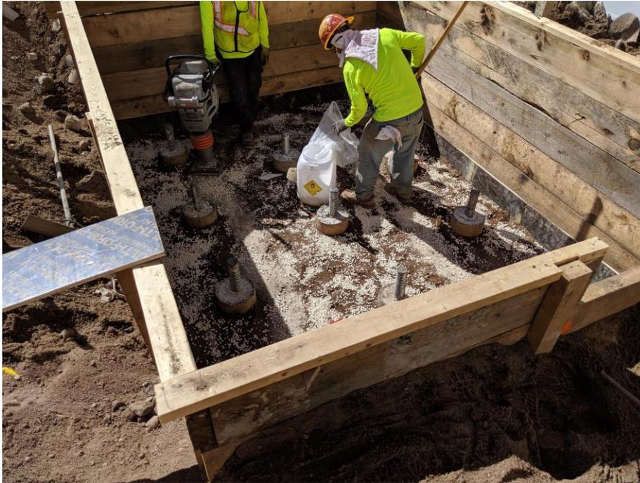
Photo 35: View of Rise applying ORC Advanced® pellets in Area #1 (6/27/2019)
