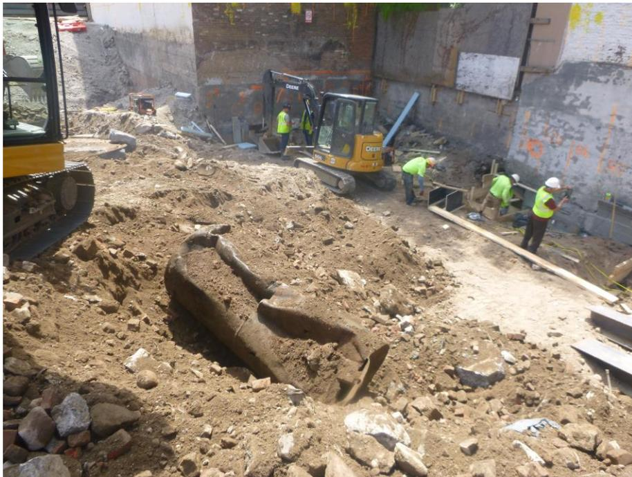
Photo 8: View of 550-gallon steel UST uncovered in Grid 1 during excavation activities, facing south (6/20/2018)
