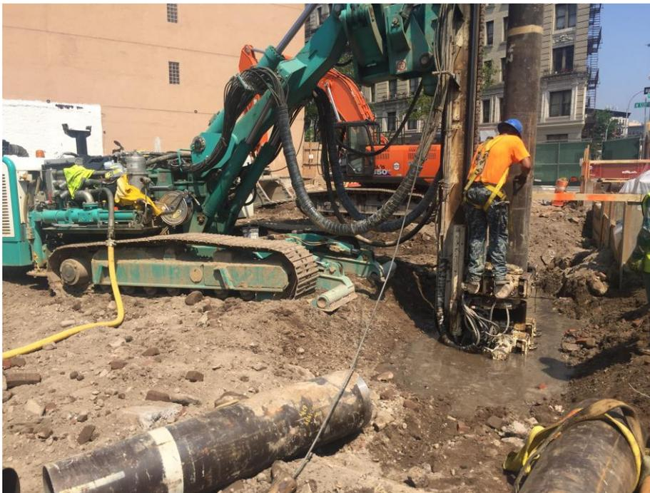
Photo 12: View of Moncon drilling soldier pile S24, facing north (8/7/2018)
