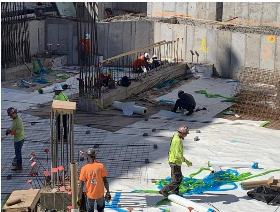
Photo 48: View of DripDrop installing Grace Preprufe® 300R Plus waterproofing membrane in Grid 3, facing southwest (9/29/2019)
