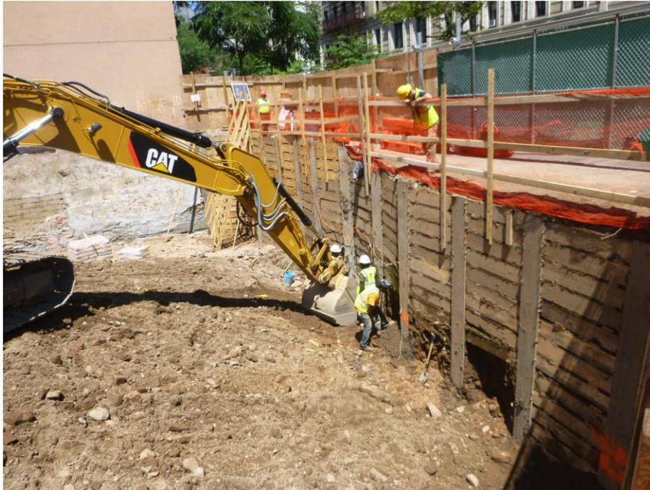
Photo 11: View of Moncon excavating Grid 2 (5-10) for timber lagging installation, facing west (7/19/2018)
