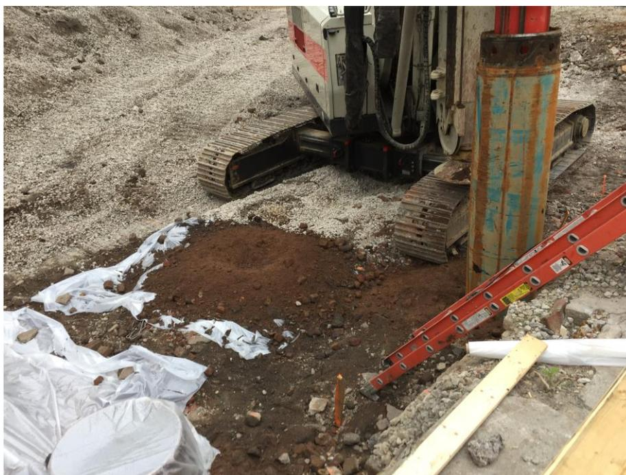
Photo 4: Moncon installing soldier pile S7 casing, facing northwest (5/31/2018)
