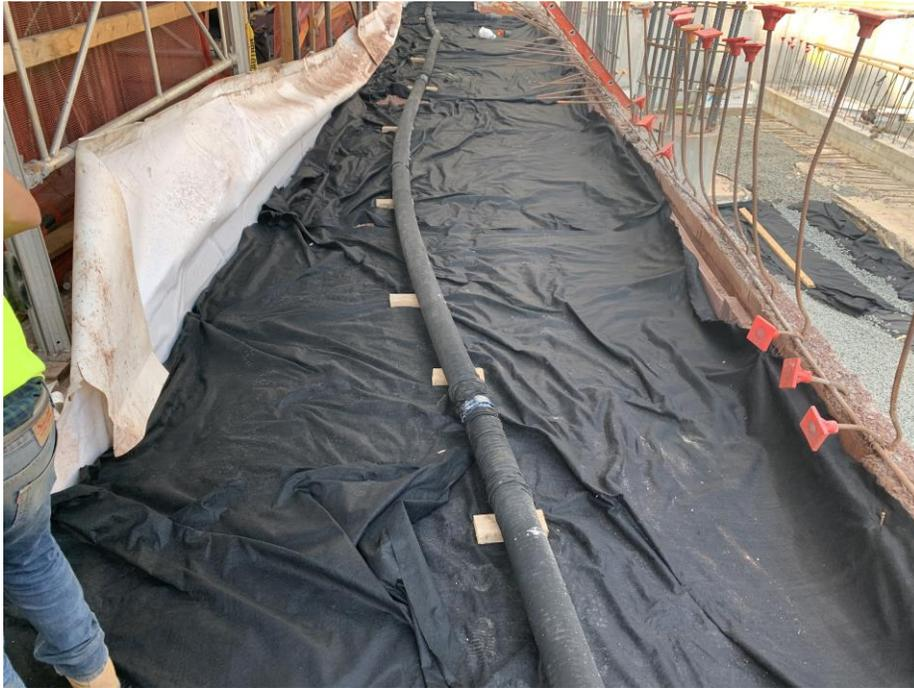
Photo 47: View of SMD system piping before surrounding with stone in Grid 3, facing west (9/26/2019)
