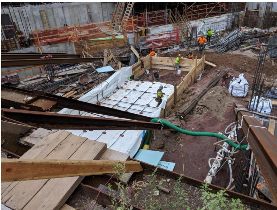
Photo 42: View of DripDrop installing Grace Preprufe® 160R Plus and 300R Plus waterproofing membrane in Grid 4, facing southwest (8/19/2019)
