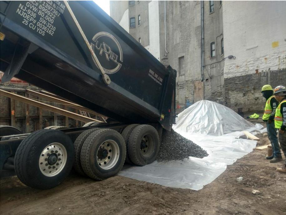
Photo 24: View of Rise importing ¾-inch virgin stone from RockTech of New Jersey, facing southeast (4/11/2019)
