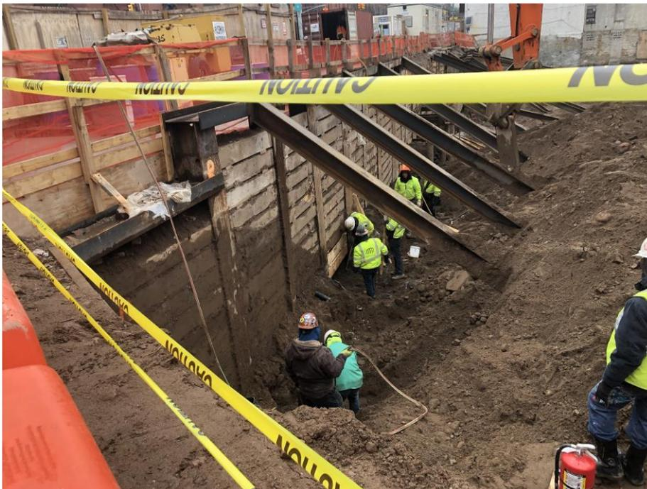
Photo 22: View of Moncon installing lagging along eastern site boundary in Grid 2, facing southeast (2/18/2019)
