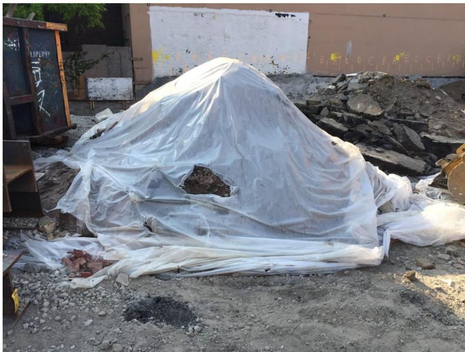
Photo 5: View of stockpiled soil cuttings from soldier piles, facing west (6/7/2018)
