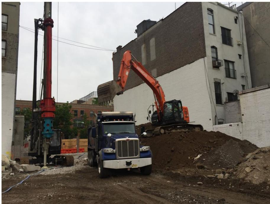
Photo 3: Moncon loading soil from Grid 1 (0-5) material for offsite disposal, facing south (5/18/2018)
