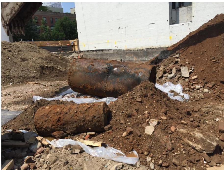
Photo 10: View of a 50-gallon and a 550-gallon steel USTs uncovered during excavation and staged on polyethylene sheeting, facing west (7/11/2018)
