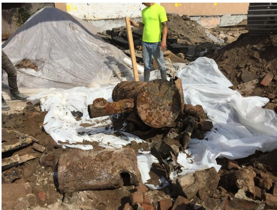
Photo 6: View of uncovered underground storage tank (UST), facing west (6/8/2018)
