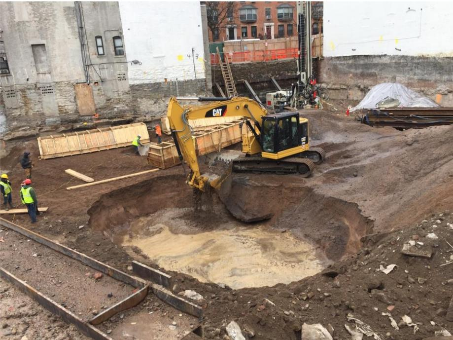
Photo 20: Moncon excavating soil in Grid 4 (14-18) for heel block installation, facing southwest (11/20/2019)
