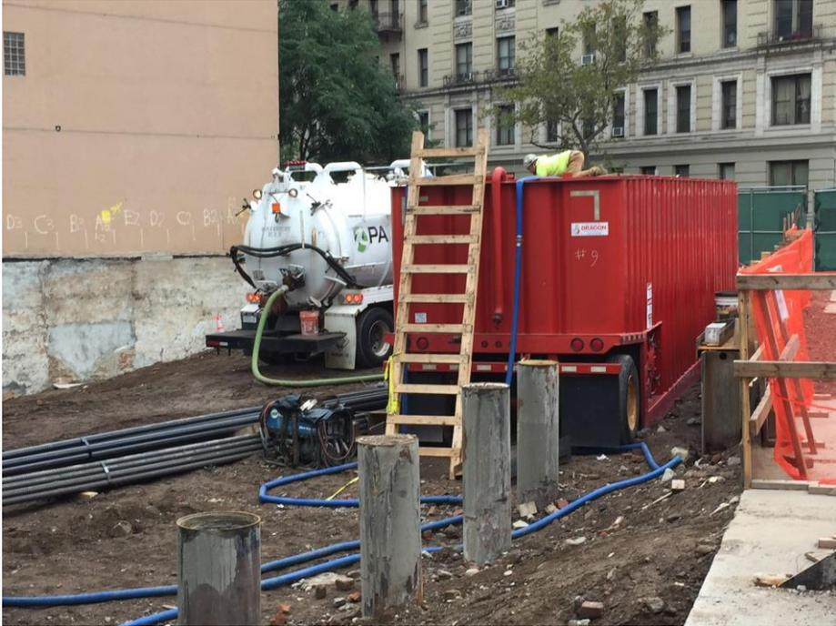
Photo 15: View of PAL Environmental Services Corp. pumping drilling water from frac tank into vacuum truck for offsite disposal, facing northwest (9/14/2018)
