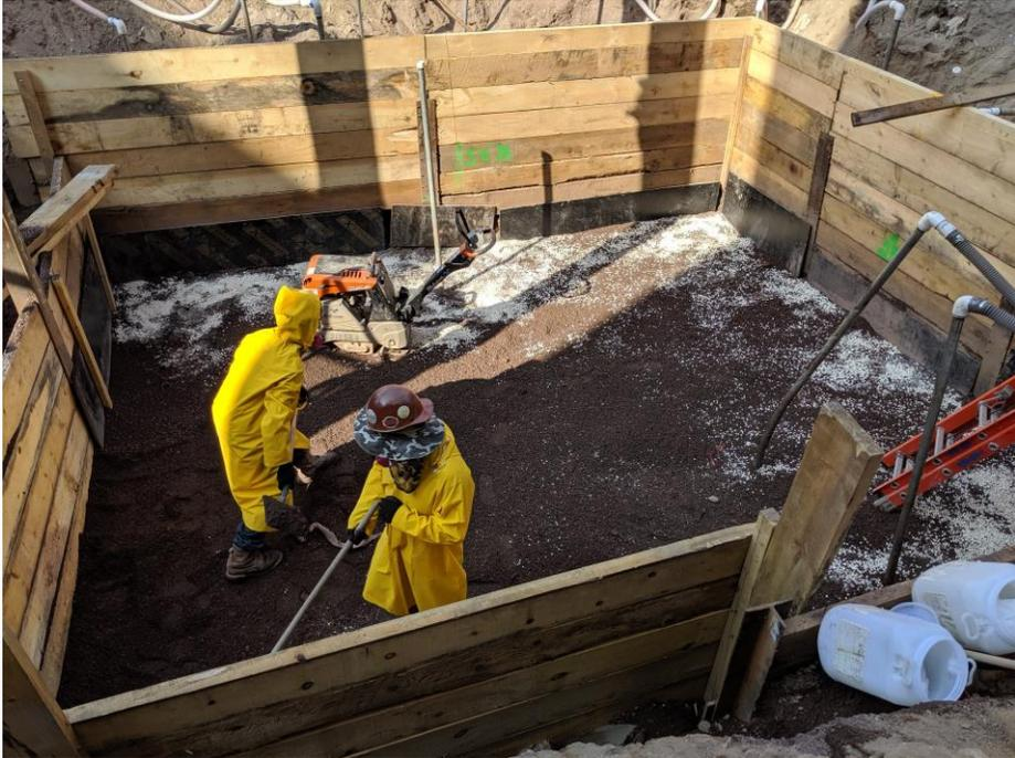
Photo 39: View of Rise mixing ORC Advanced® pellets with ½-inch minus virgin stone, facing northeast (7/10/2019)
