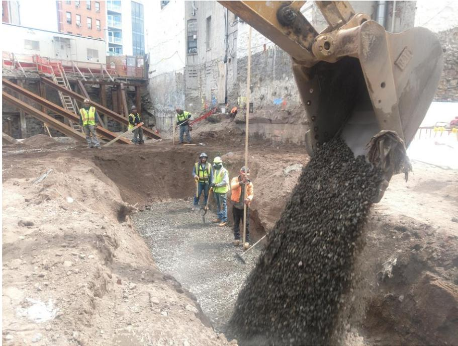
Photo 25: View of Rise backfilling excavation with  $\frac{3}{4}$ -inch virgin stone in Grids 3 and 4 between 19 and 20 feet bgs, facing southeast (4/30/2019)
