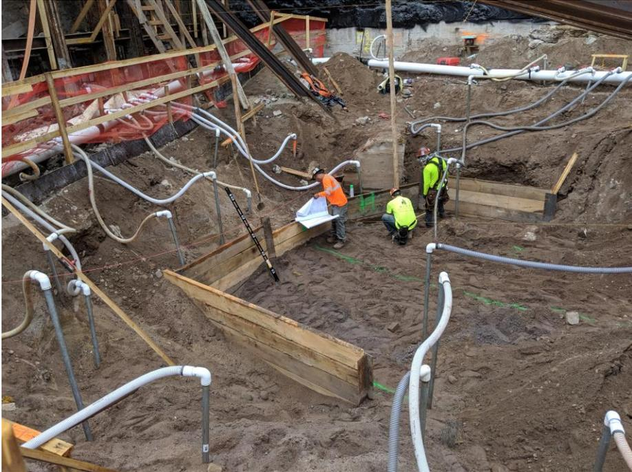
Photo 37: View of elevator pit excavation in Grid 4 and surrounding dewatering system, facing southeast (7/8/2019)
