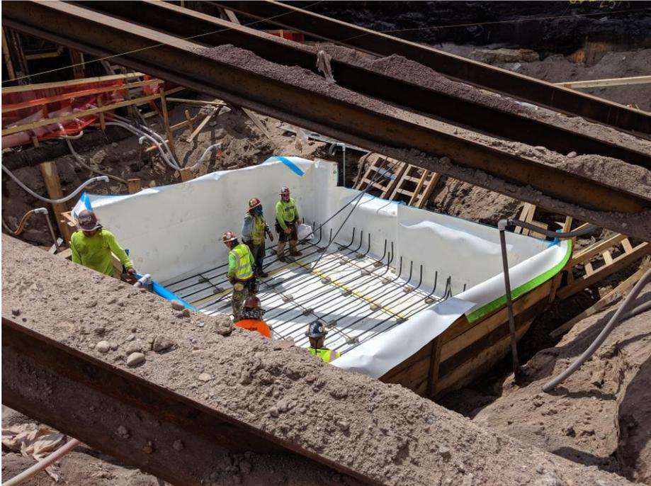
Photo 40: View of Men of Steel installing rebar in Grid 4, facing southeast (7/11/2019)
