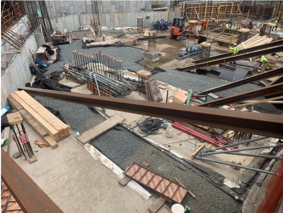
Photo 45: View of Grids 3 and 4 after SMD gravel has been backfilled, facing northwest (9/16/2019)
