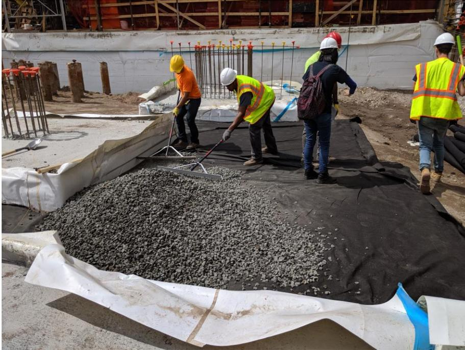
Photo 31: View of Hydrotech spreading 3/4-inch virgin stone from Tilcon – West Nyack Quarry on geotextile fabric for SMD system installation in Grid 3, facing south (6/7/2019)
