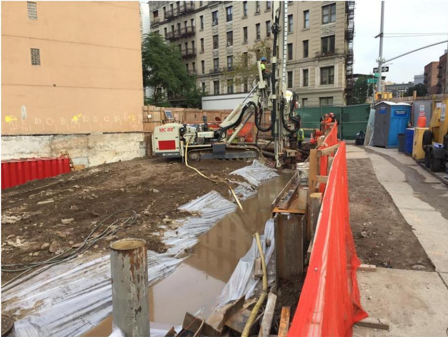
Photo 16: View of Moncon drilling production pile 22 in Grid 3, facing north (10/4/2018)
