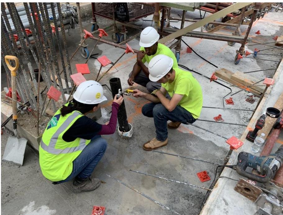
Photo 50: View of Hydrotech installing a sampling port in the riser pipe, facing southeast (10/02/2019)
