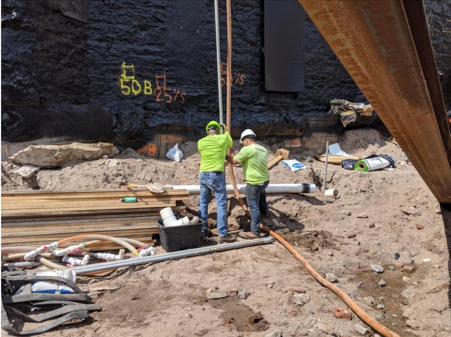
Photo 29: View of Hydrotech installing well points for dewatering system in Grid 4, facing south (6/3/2019)
