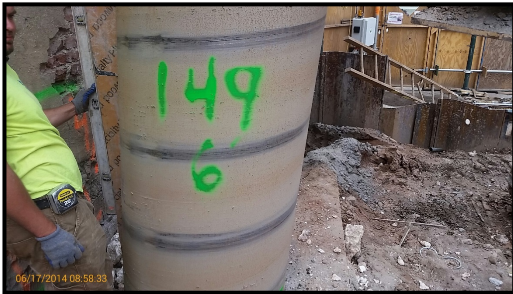
Photo 97: Battered secant pile #149P; confirming 6 degree tilt at EL +5 using a jig and bubble level.
