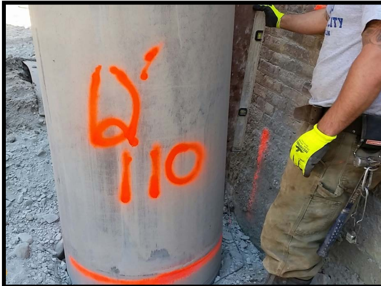
Photo 60: Battered secant pile #110S; confirming 6 degree tilt at EL +0 using a jig and bubble level.
