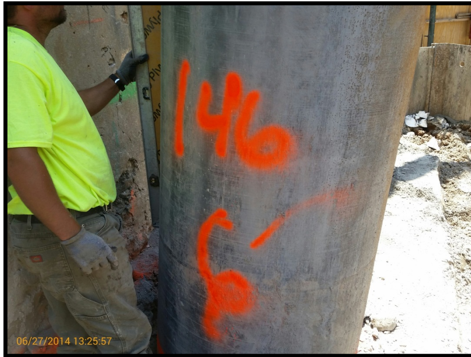
Photo 127: Battered secant pile #146S; confirming 6 degree tilt at EL +5 using a jig and bubble level.
