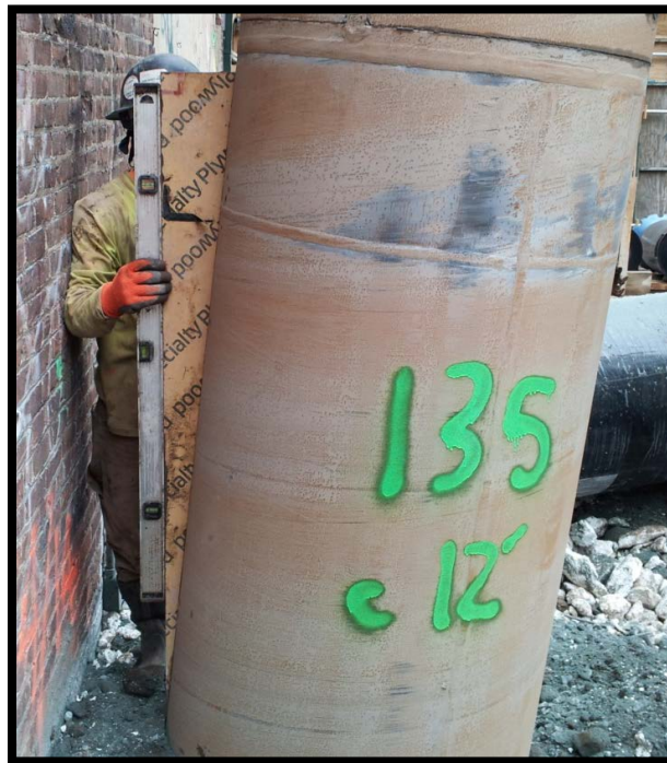
Photo 40: Battered secant pile #135P; confirming 6 degree tilt at EL +0 using a jig and bubble level.
