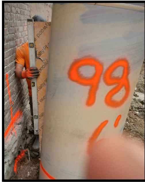
Photo 67: Battered secant pile #98S; confirming 6 degree tilt at EL +5 using a jig and bubble level.
