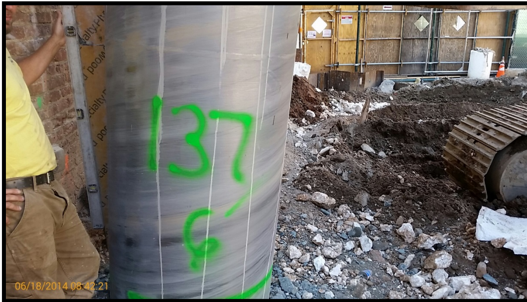
Photo 89: Battered secant pile #137P; confirming 6 degree tilt at EL +5 using a jig and bubble level.
