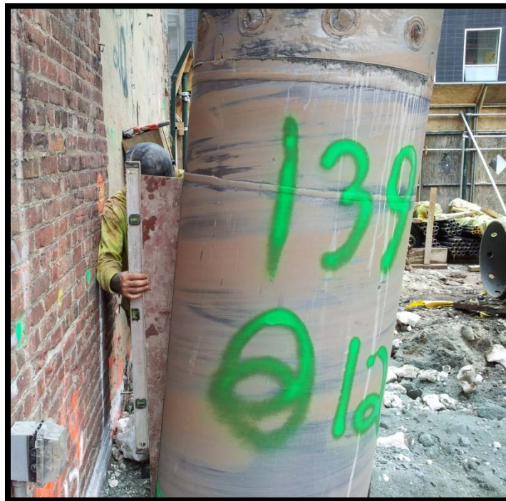
Photo 42: Battered secant pile #139P; confirming 6 degree tilt at EL +0 using a jig and bubble level.
