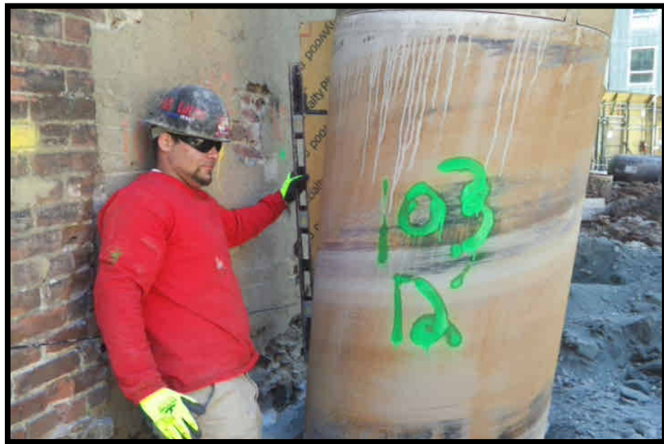
Photo 24: Battered secant pile #103P; confirming 6 degree tilt at EL +0 using a jig and bubble level.
