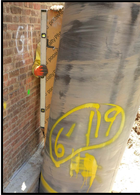
Photo 31: Battered secant pile #119P; confirming 6 degree tilt at EL +5 using a jig and bubble level.
