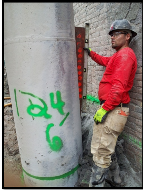
Photo 91: Battered secant pile #124S; confirming 6 degree tilt at EL +5 using a jig and bubble level.
