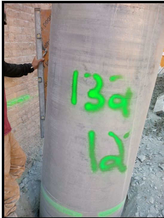
Photo 116: Battered secant pile #132S; confirming 6 degree tilt at EL +0 using a jig and bubble level.
