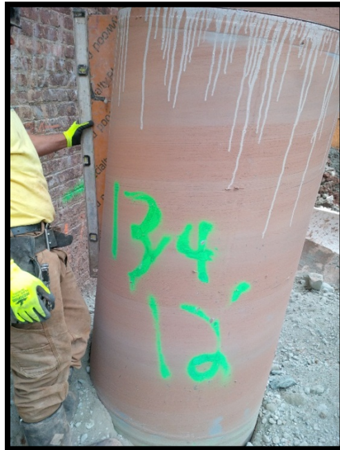
Photo 106: Battered secant pile #134S; confirming 6 degree tilt at EL +0 using a jig and bubble level.
