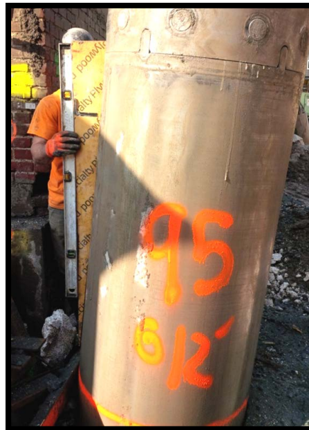
Photo 64: Battered secant pile #95P; confirming 6 degree tilt at EL +0 using a jig and bubble level.
