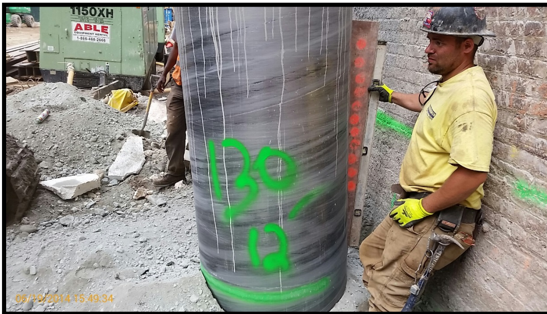
Photo 110: Battered secant pile #130S; confirming 6 degree tilt at EL +0 using a jig and bubble level.
