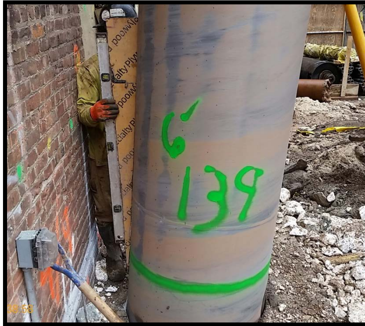
Photo 41: Battered secant pile #139P; confirming 6 degree tilt at EL +5 using a jig and bubble level.
