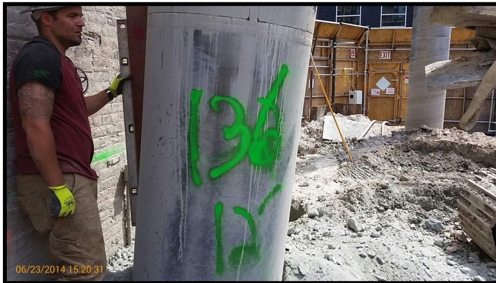
Photo 118: Battered secant pile #136S; confirming 6 degree tilt at EL +0 using a jig and bubble level.
