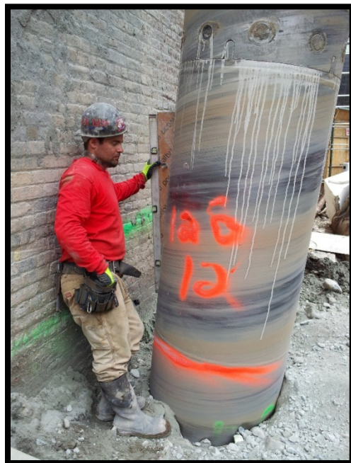
Photo 94: Battered secant pile #128S; confirming 6 degree tilt at EL +0 using a jig and bubble level.
