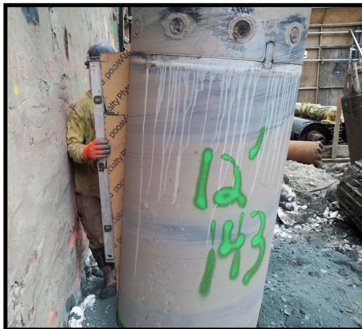
Photo 44: Battered secant pile #143P; confirming 6 degree tilt at EL +0 using a jig and bubble level.
