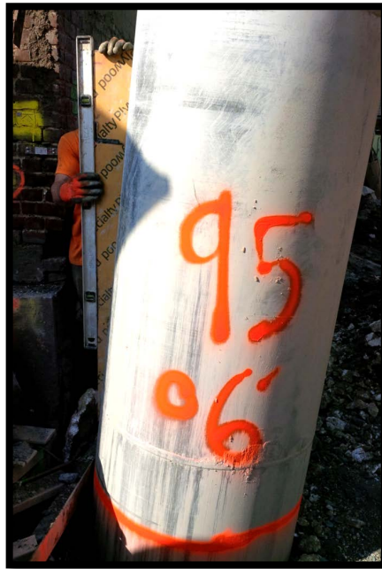
Photo 63: Battered secant pile #95P; confirming 6 degree tilt at EL +5 using a jig and bubble level.
