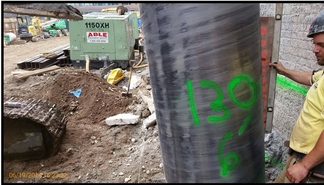
Photo 109: Battered secant pile #130S; confirming 6 degree tilt at EL +5 using a jig and bubble level.
