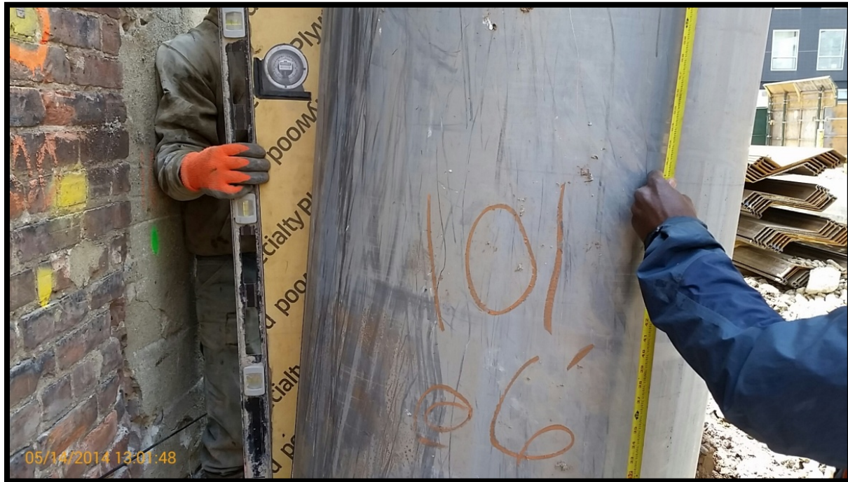
Photo 5: Battered secant pile #101P; confirming 6 degree tilt at EL +5 using a jig and bubble level.
