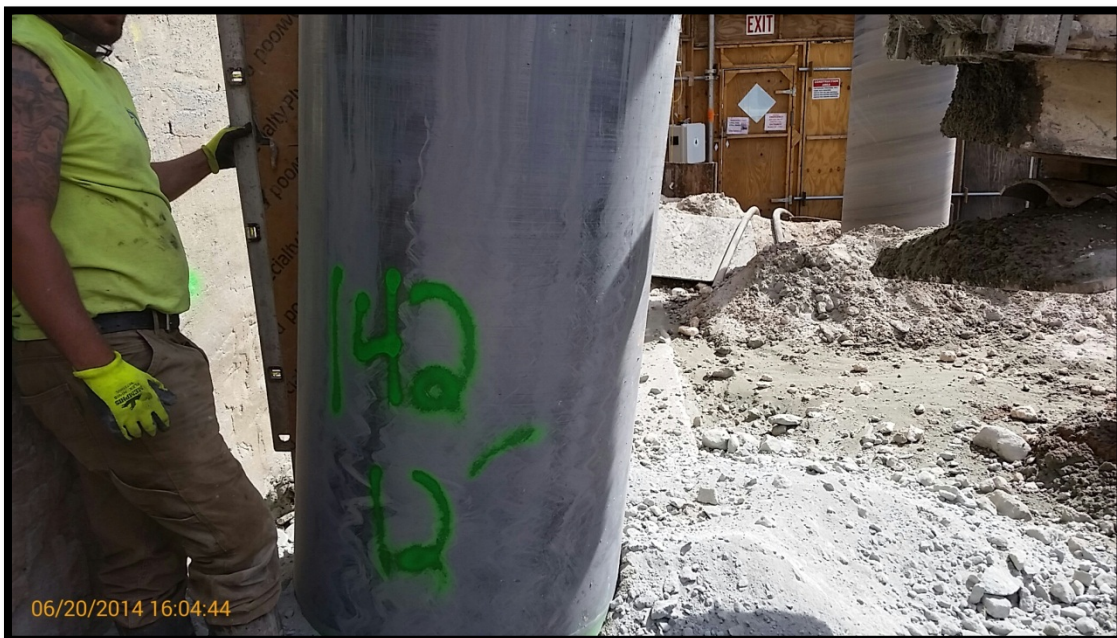
Photo 114: Battered secant pile #142S; confirming 6 degree tilt at EL +0 using a jig and bubble level.
