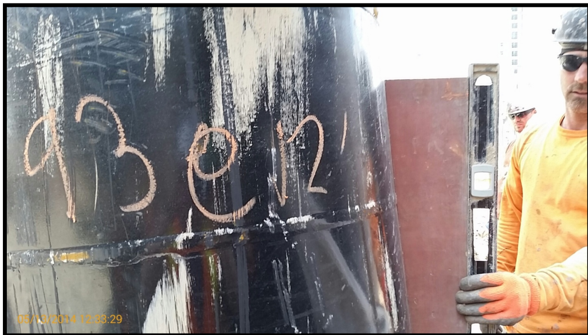
Photo 4: Battered secant pile #93P; confirming 6 degree tilt at EL +0 using a jig and bubble level.
