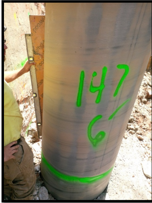
Photo 101: Battered secant pile #147P; confirming 6 degree tilt at EL +5 using a jig and bubble level.
