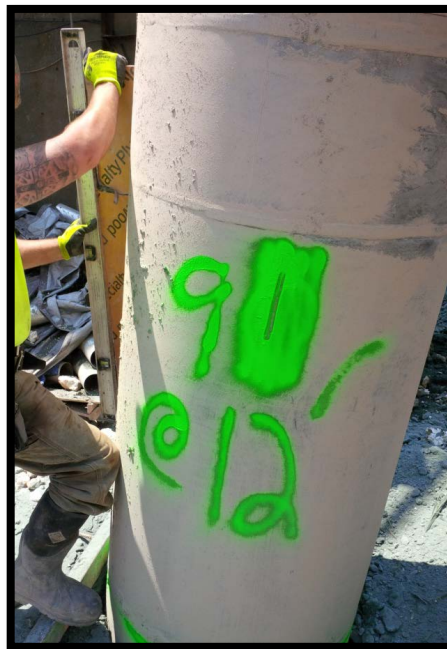
Photo 62: Battered secant pile #91P; confirming 6 degree tilt at EL +0 using a jig and bubble level.
