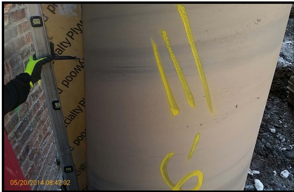
Photo 27: Battered secant pile #111P; confirming 6 degree tilt at EL +5 using a jig and bubble level.
