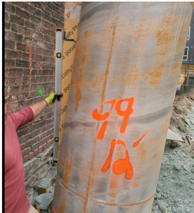
Photo 22: Battered secant pile #99P; confirming 6 degree tilt at EL +0 using a jig and bubble level.
