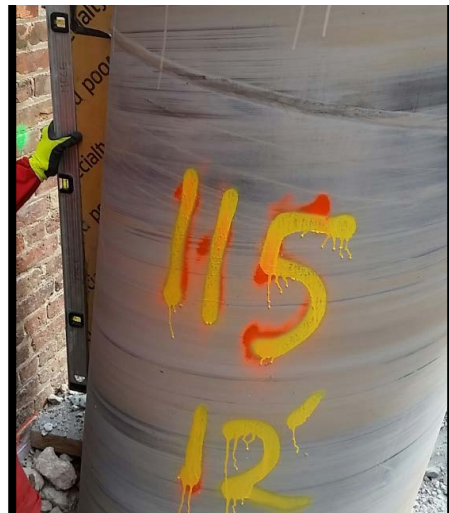
Photo 26: Battered secant pile #115P; confirming 6 degree tilt at EL +0 using a jig and bubble level.
