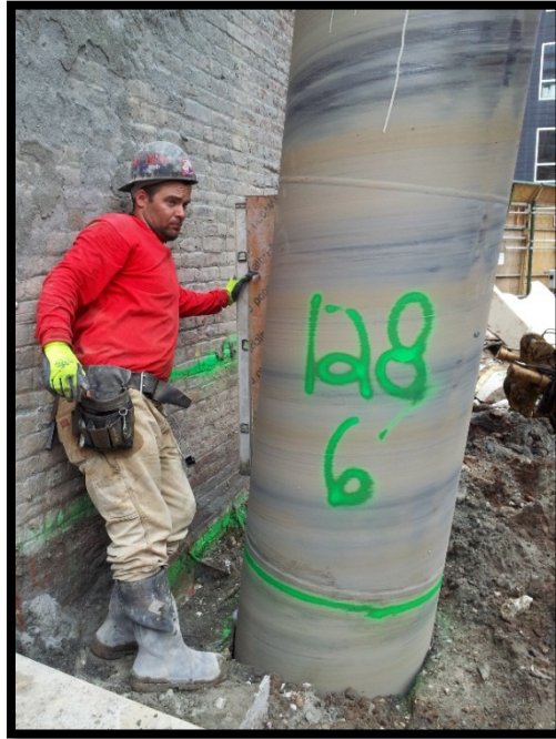
Photo 93: Battered secant pile #128S; confirming 6 degree tilt at EL +5 using a jig and bubble level.
