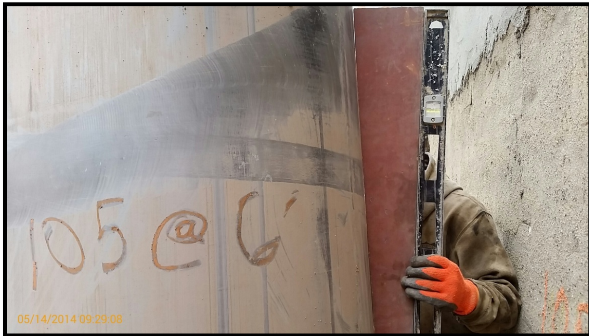
Photo 7: Battered secant pile #105P; confirming 6 degree tilt at EL +5 using a jig and bubble level.
