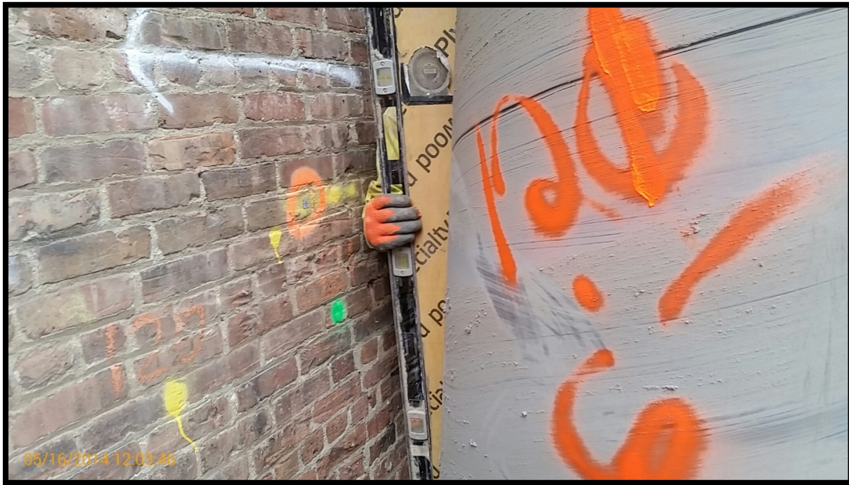
Photo 17: Battered secant pile #121P; confirming 6 degree tilt at EL +5 using a jig and bubble level.
