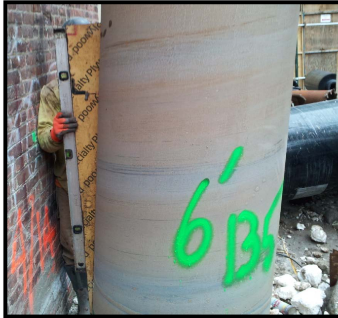
Photo 39: Battered secant piling #135P; confirming 6 degree tilt at EL +5 using a jig and bubble level.
