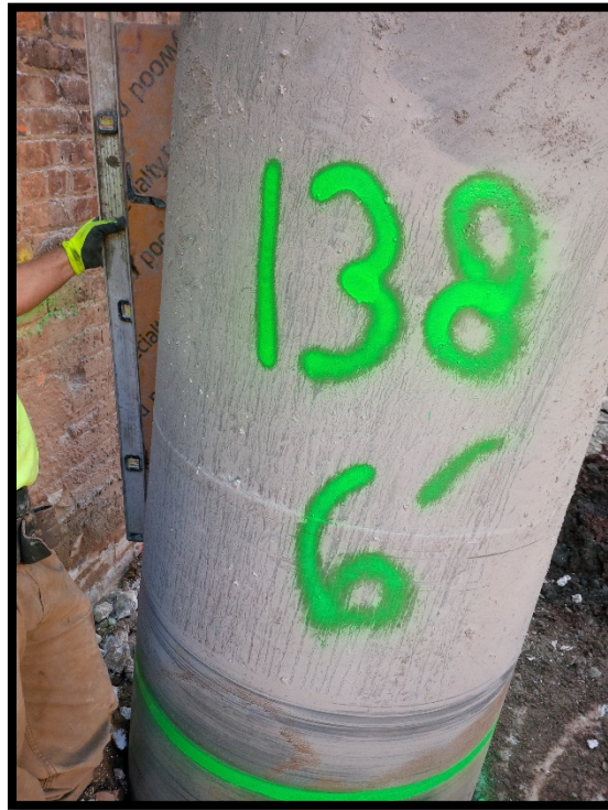
Photo 111: Battered secant pile #138S; confirming 6 degree tilt at EL +5 using a jig and bubble level.
