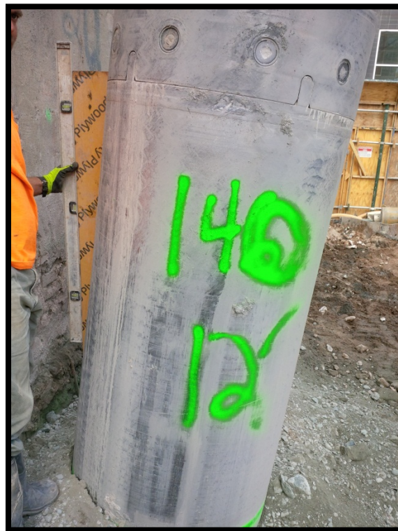
Photo 126: Battered secant pile #140S; confirming 6 degree tilt at EL +0 using a jig and bubble level.
