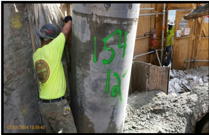
Photo 132A (left) & 132B (right): Battered secant pile #154S; confirming 6 degree tilt at EL +0 using a jig and bubble level.
