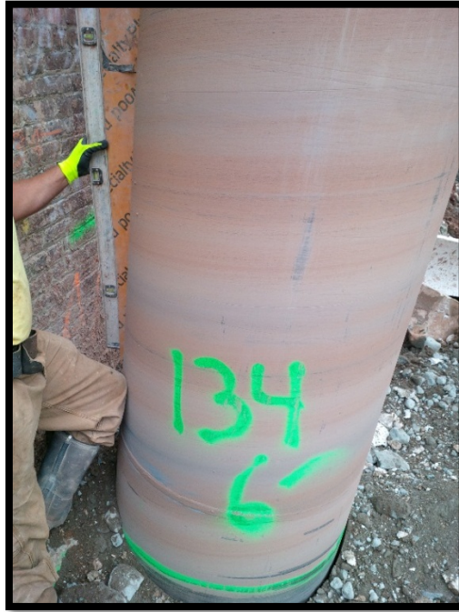
Photo 105: Battered secant pile #134S; confirming 6 degree tilt at EL +5 using a jig and bubble level.
