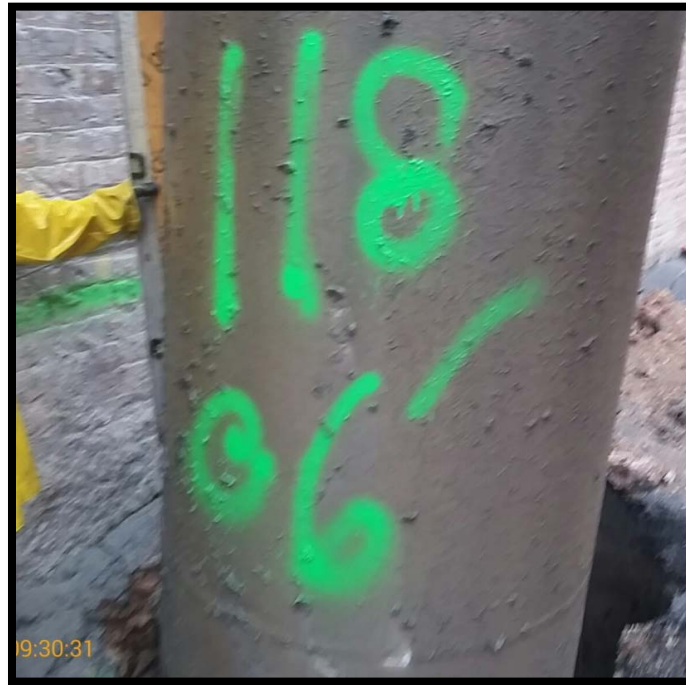
Photo 79: Battered secant pile #118S; confirming 6 degree tilt at EL +5 using a jig and bubble level.
