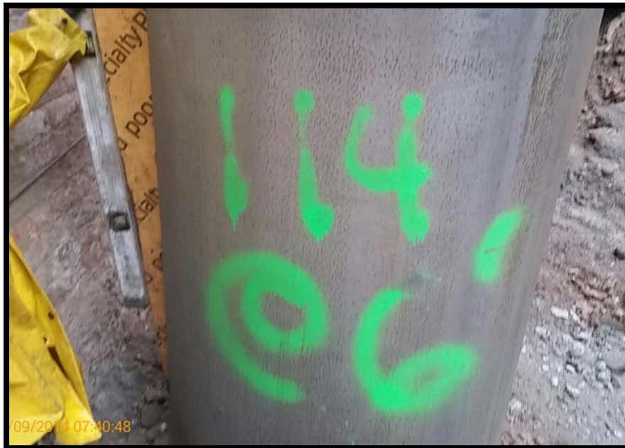
Photo 77: Battered secant pile #114S; confirming 6 degree tilt at EL +5 using a jig and bubble level.
