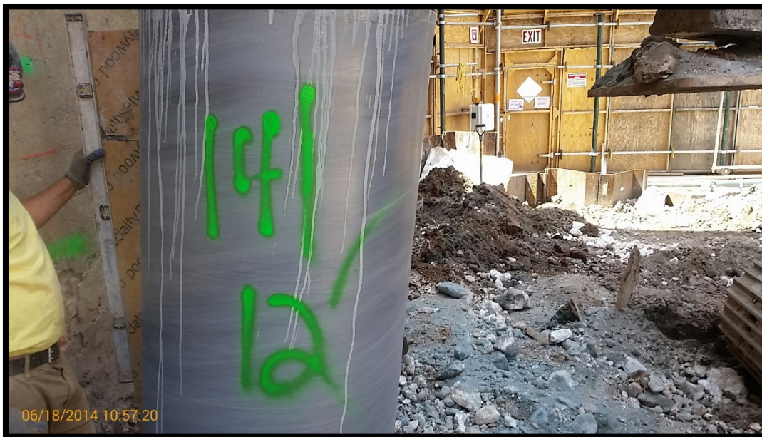
Photo 104: Battered secant pile #141P; confirming 6 degree tilt at EL +0 using a jig and bubble level.
