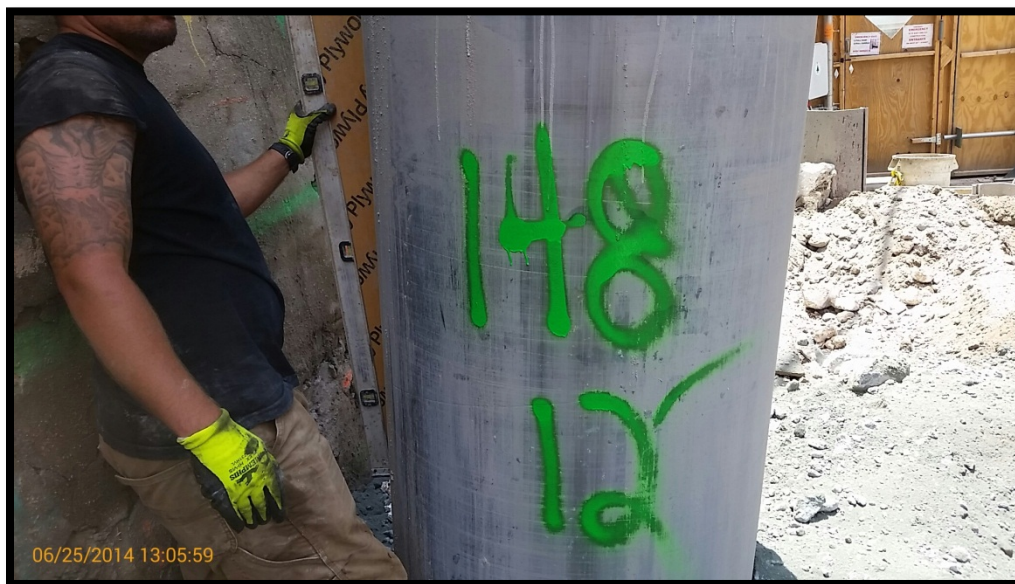
Photo 124: Battered secant pile #148S; confirming 6 degree tilt at EL +0 using a jig and bubble level.
