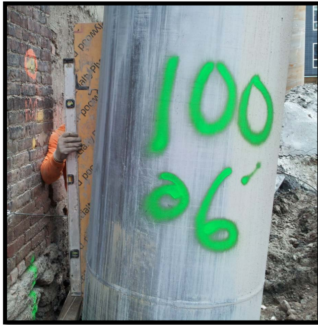
Photo 49: Battered secant pile #100S; confirming 6 degree tilt at EL +5 using a jig and bubble level.
