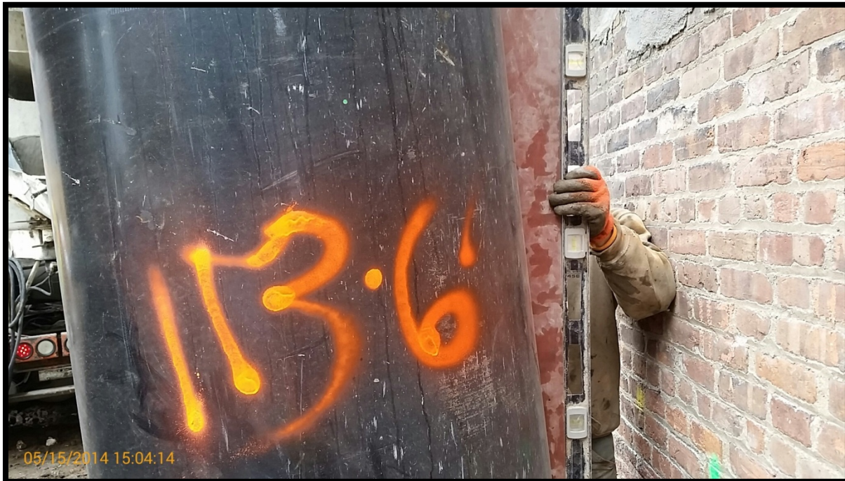
Photo 13: Battered secant pile #113P; confirming 6 degree tilt at EL +5 using a jig and bubble level.
