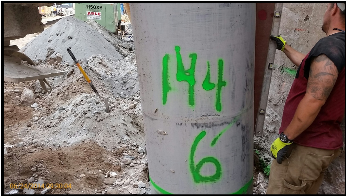
Photo 119: Battered secant pile #144S; confirming 6 degree tilt at EL +5 using a jig and bubble level.
