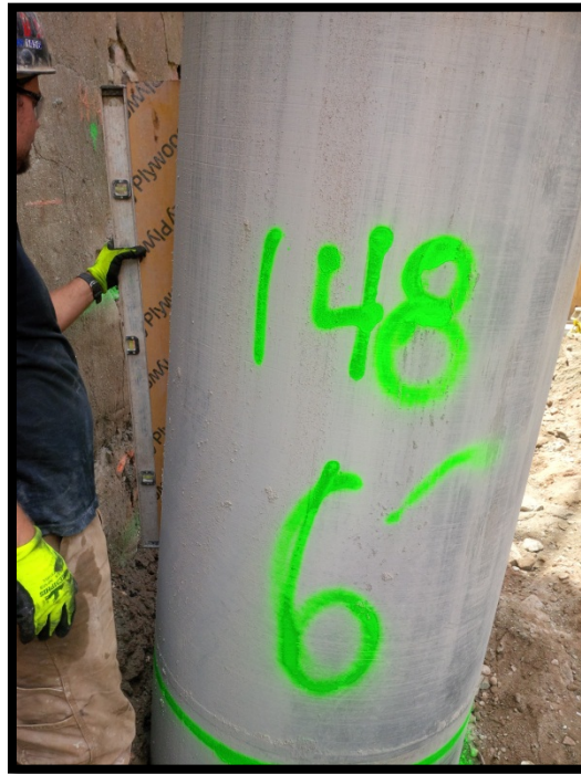
Photo 123: Battered secant pile #148S; confirming 6 degree tilt at EL +5 using a jig and bubble level.
