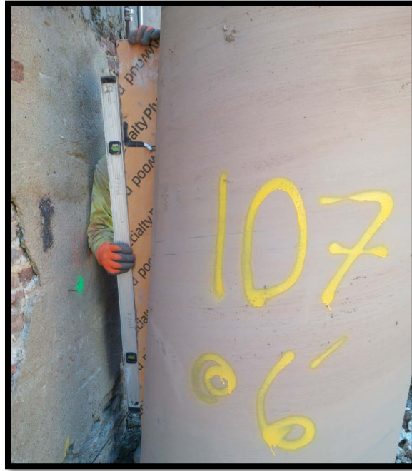
Photo 29: Battered secant pile #107P; confirming 6 degree tilt at EL +5 using a jig and bubble level.
