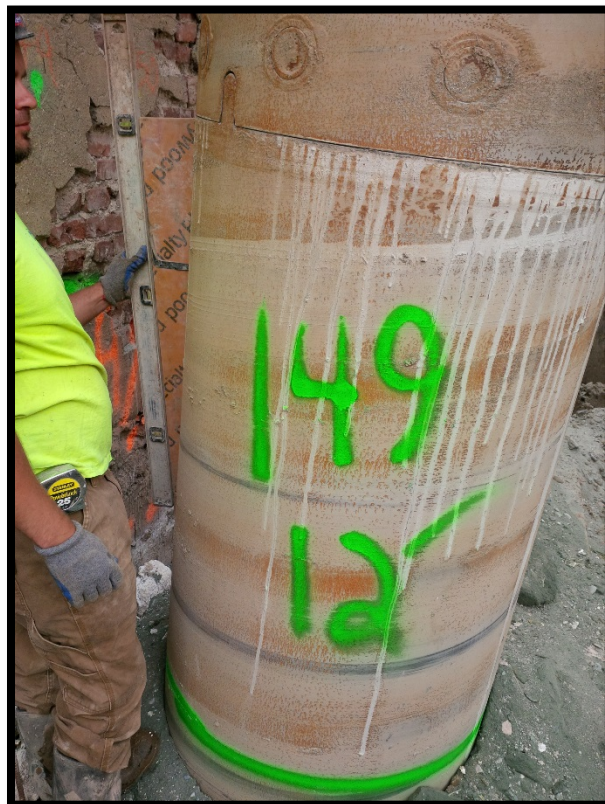
Photo 98: Battered secant pile #149P; confirming 6 degree tilt at EL +0 using a jig and bubble level.
