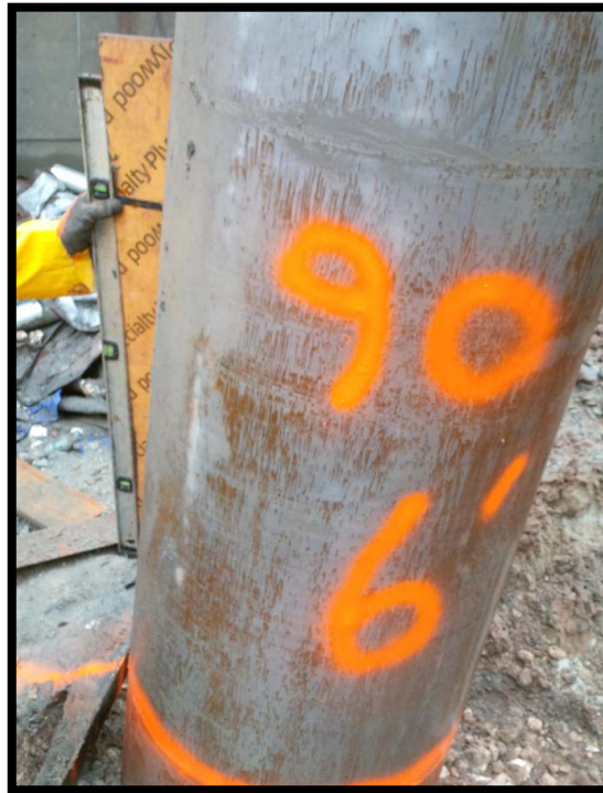
Photo 69: Battered secant pile #90S; confirming 6 degree tilt at EL +5 using a jig and bubble level.
