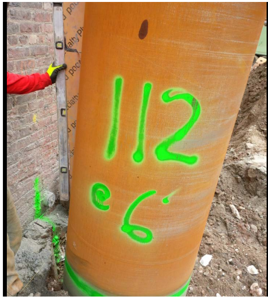
Photo 51: Battered secant pile #112S; confirming 6 degree tilt at EL +5 using a jig and bubble level.
