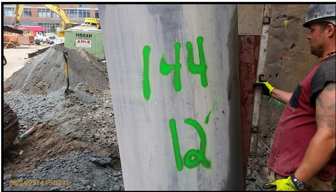
Photo 120: Battered secant pile #144S; confirming 6 degree tilt at EL +0 using a jig and bubble level.
