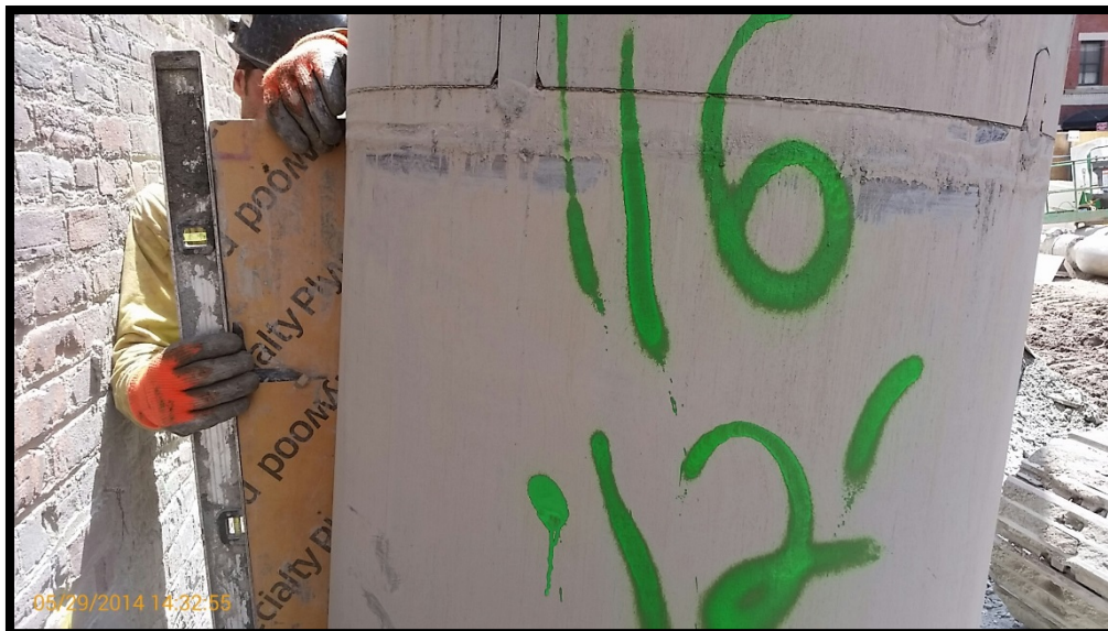
Photo 56: Battered secant pile #116S; confirming 6 degree tilt at EL +0 using a jig and bubble level.
