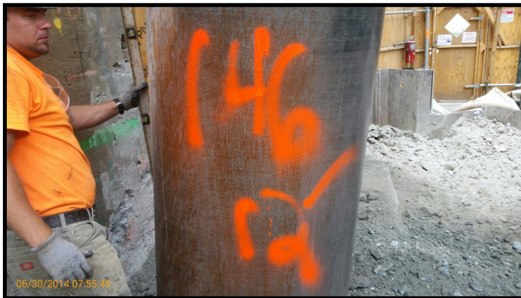
Photo 128: Battered secant pile #146S; confirming 6 degree tilt at EL +0 using a jig and bubble level.
