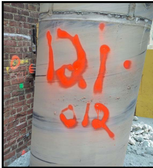
Photo 18: Battered secant pile #121P; confirming 6 degree tilt at EL +0 using a jig and bubble level.
