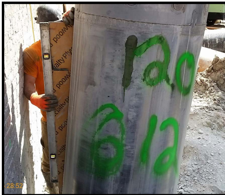
Photo 58: Battered secant pile #120S; confirming 6 degree tilt at EL +0 using a jig and bubble level.
