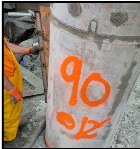
Photo 70: Battered secant pile #90S; confirming 6 degree tilt at EL +0 using a jig and bubble level.
