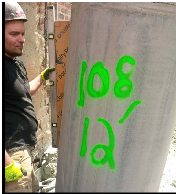
Photo 48: Battered secant pile #108S; confirming 6 degree tilt at EL +0 using a jig and bubble level.
