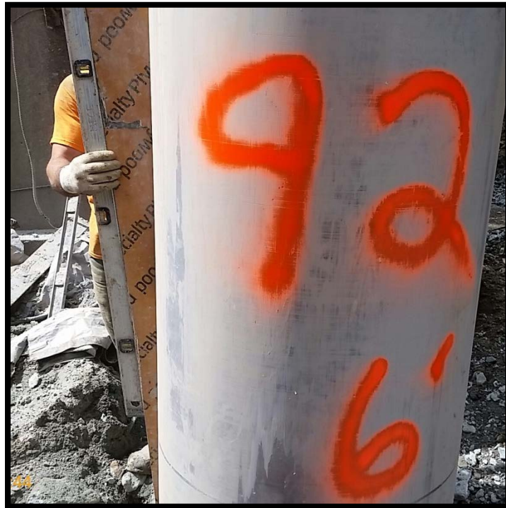
Photo 73: Battered secant pile #92S; confirming 6 degree tilt at EL +5 using a jig and bubble level.
