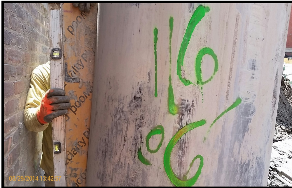
Photo 55: Battered secant pile #116S; confirming 6 degree tilt at EL +5 using a jig and bubble level.
