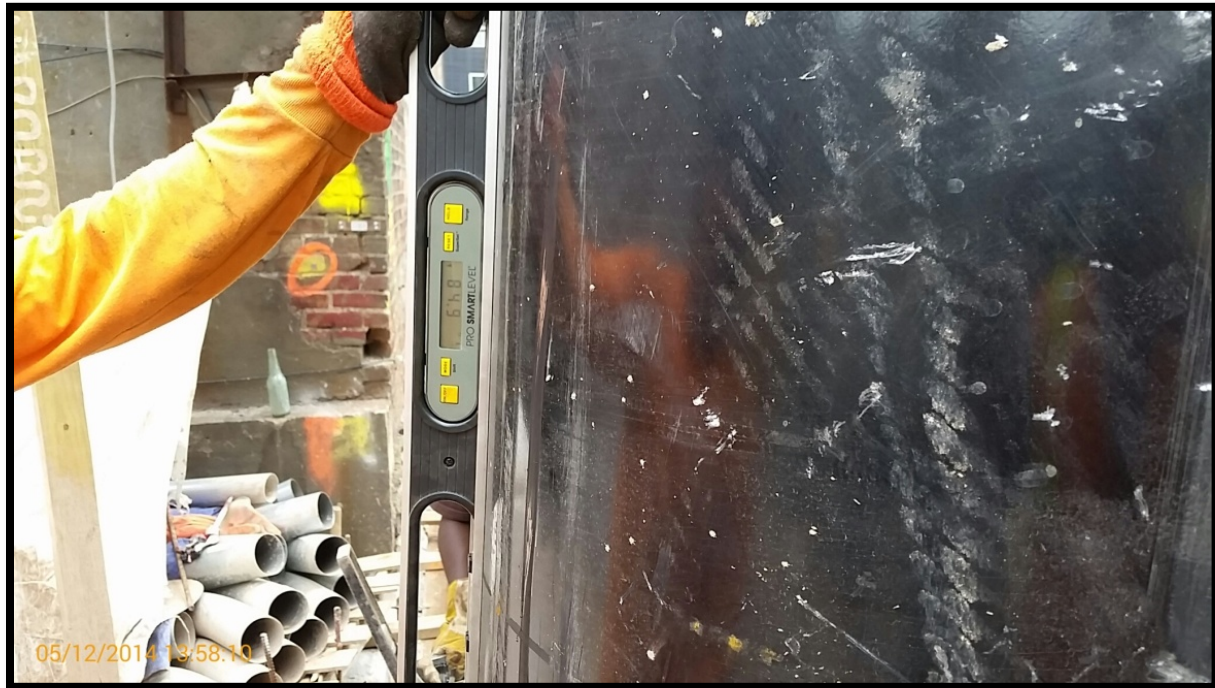
Photo 1: Battered secant pile #89P; confirming 6 degree casing tilt at EL +5 using a jig and bubble level.
