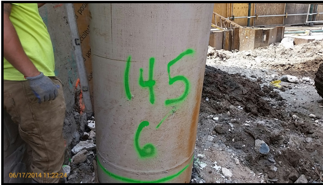
Photo 95: Battered secant pile #145P; confirming 6 degree tilt at EL +5 using a jig and bubble level.
