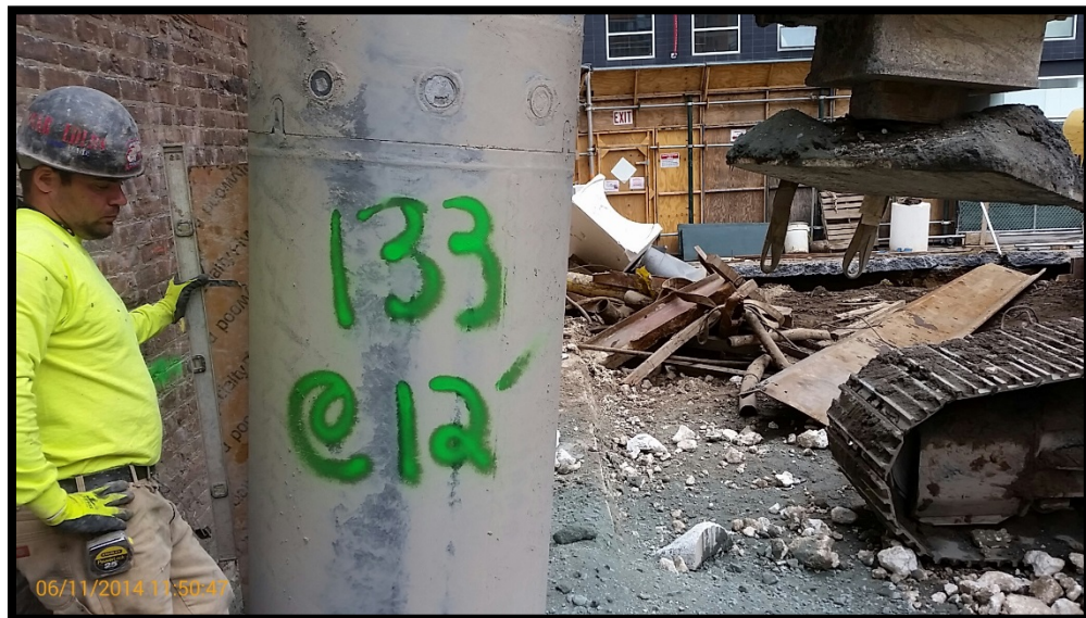
Photo 88: Battered secant pile #133P; confirming 6 degree tilt at EL +0 using a jig and bubble level.
