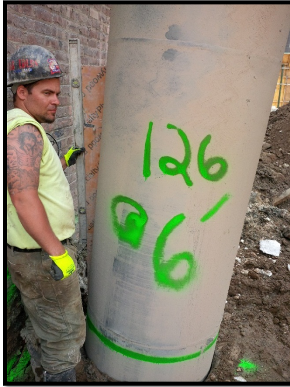
Photo 83: Battered secant pile #126S; confirming 6 degree tilt at EL +5 using a jig and bubble level.
