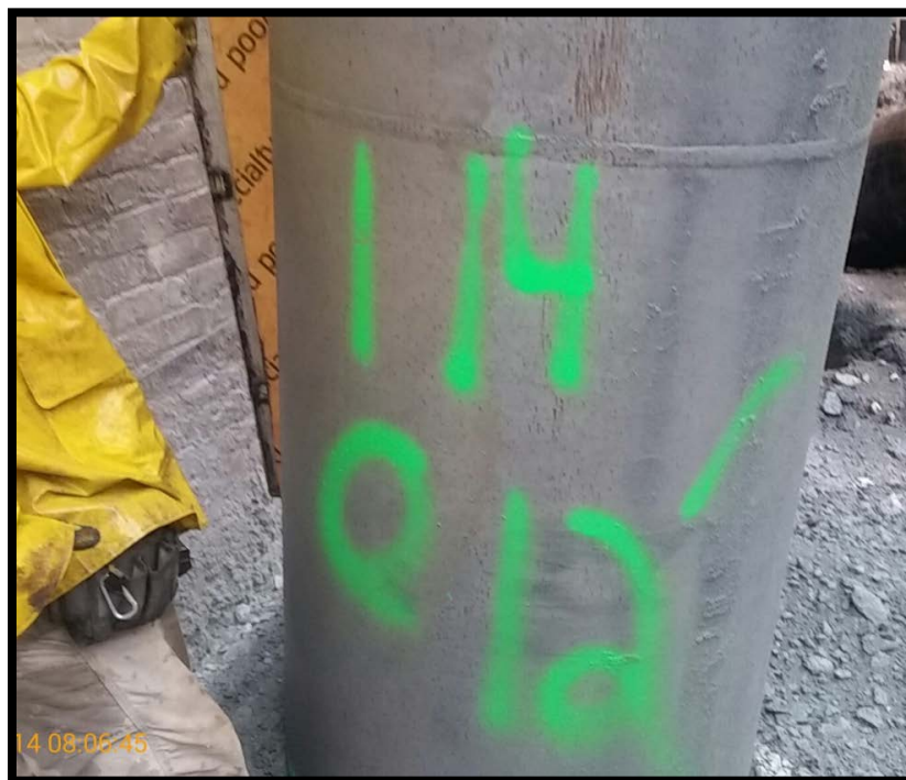
Photo 78: Battered secant pile #114S; confirming 6 degree tilt at EL +0 using a jig and bubble level.
