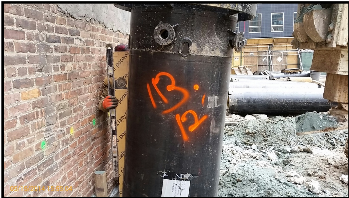
Photo 14: Battered secant pile #113P; confirming 6 degree tilt at EL +0 using a jig and bubble level.
