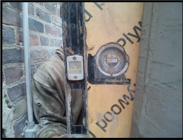
Photo 11A (left ) & 11B (right): Battered secant pile #109P; confirming 6 degree tilt at EL +5 using a jig and bubble level.
