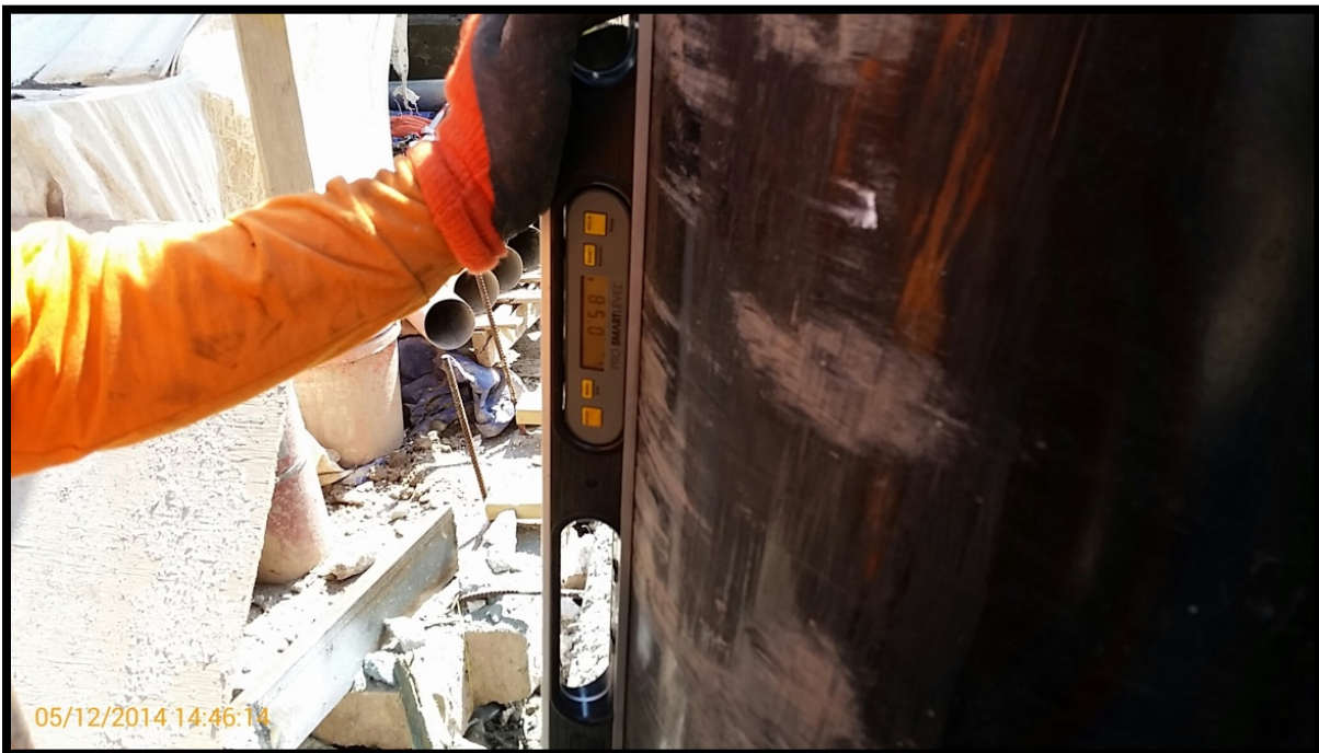
Photo 2: Battered secant pile #89P; confirming 6 degree tilt at EL +0 using a jig and bubble level.
