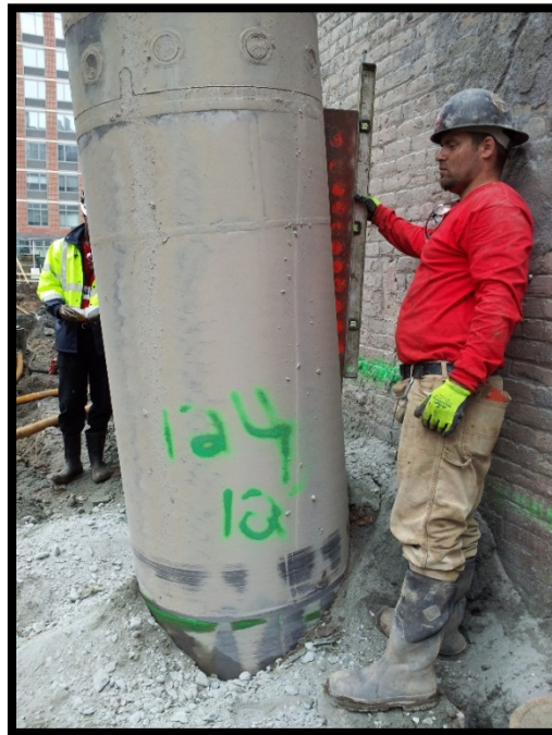
Photo 92: Battered secant pile #124S; confirming 6 degree tilt at EL +0 using a jig and bubble level.
