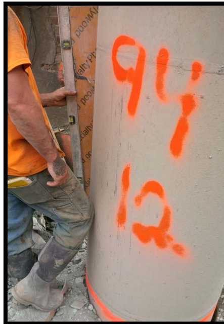
Photo 72: Battered secant pile #94S; confirming 6 degree tilt at EL +0 using a jig and bubble level.
