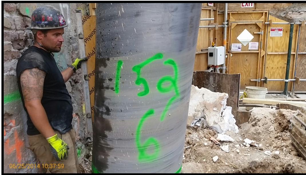
Photo 121: Battered secant pile #152S; confirming 6 degree tilt at EL +5 using a jig and bubble level.
