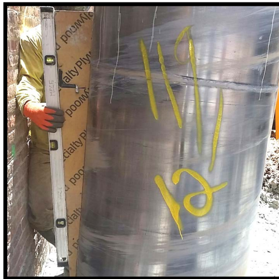
Photo 32: Battered secant pile #119P; confirming 6 degree tilt at EL +0 using a jig and bubble level.
