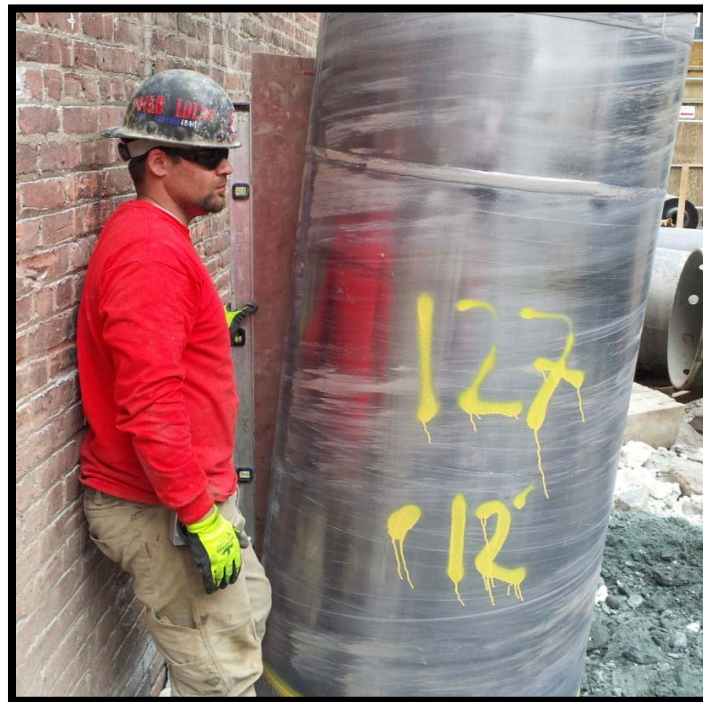
Photo 36: Battered secant pile #127P; confirming 6 degree tilt at EL +0 using a jig and bubble level.
