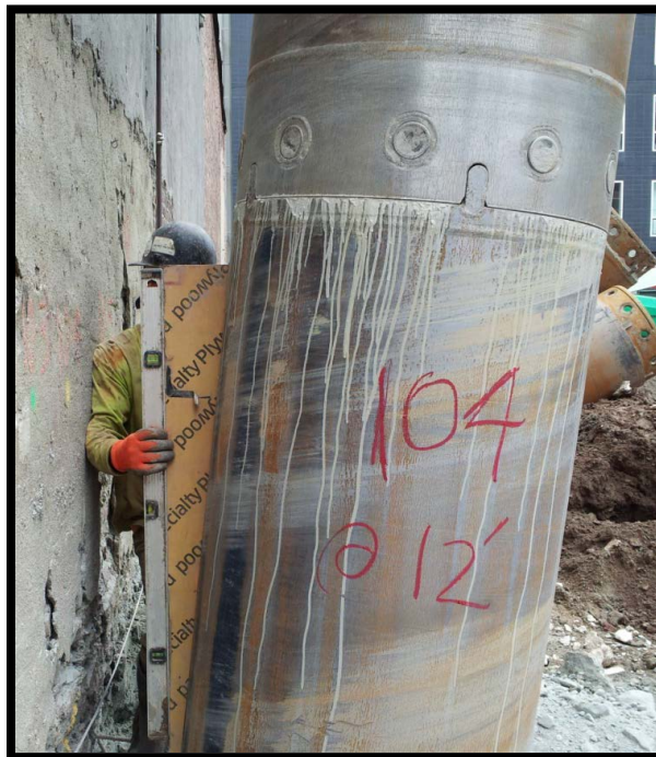
Photo 46: Battered secant pile #104S; confirming 6 degree tilt at EL +0 using a jig and bubble level.
