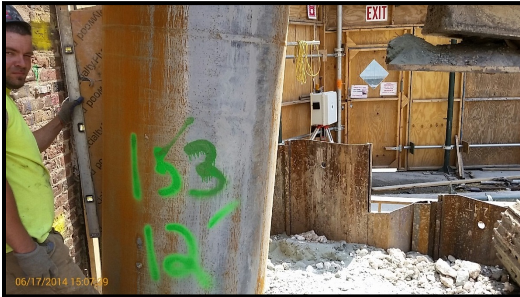
Photo 100: Battered secant pile #153P; confirming 6 degree tilt at EL +0 using a jig and bubble level.
