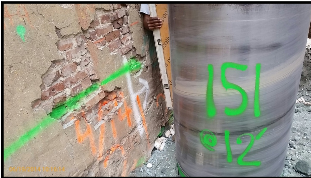
Photo 108: Battered secant pile #151P; confirming 6 degree tilt at EL +0 using a jig and bubble level.
