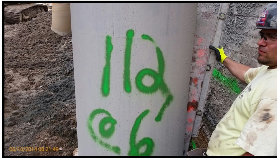
Photo 81: Battered secant pile #122S; confirming 6 degree tilt at EL +5 using a jig and bubble level.
