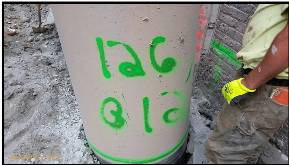
Photo 84: Battered secant pile #126S; confirming 6 degree tilt at EL +0 using a jig and bubble level.
