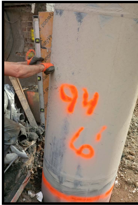
Photo 71: Battered secant pile #94S; confirming 6 degree tilt at EL +5 using a jig and bubble level.
