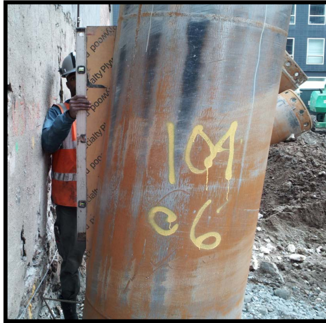
Photo 45: Battered secant pile #104S; confirming 6 degree tilt at EL +5 using a jig and bubble level.
