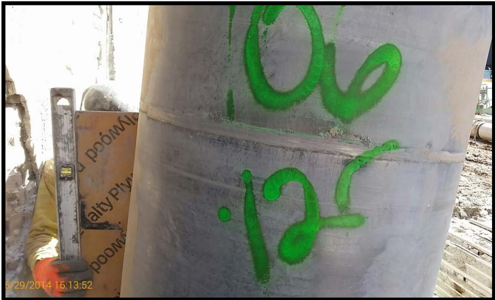
Photo 54: Battered secant pile #106S; confirming 6 degree tilt at EL +0 using a jig and bubble level.
