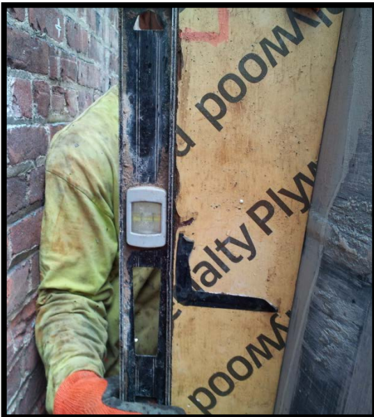
Photo 20A (left) & 20B (right): Battered secant pile #125P; confirming 6 degree tilt at EL +0 using a jig and bubble level.
