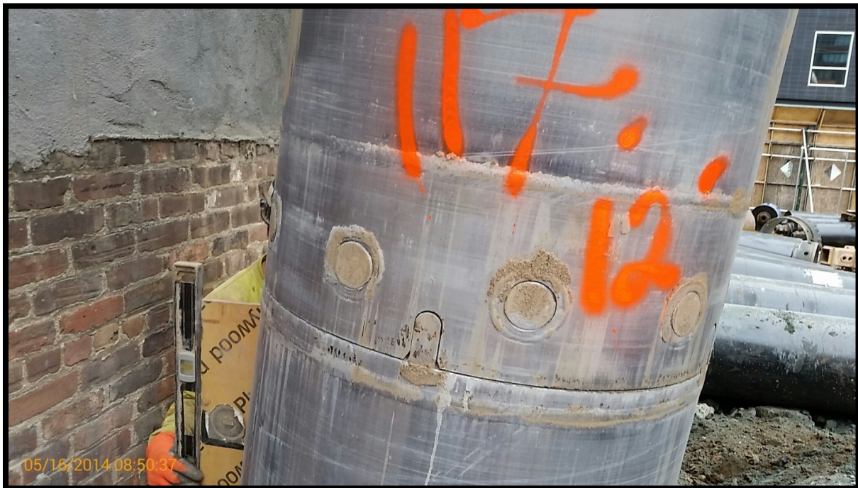
Photo 16: Battered secant pile #117P; confirming 6 degree tilt at EL +0 using a jig and bubble level.
