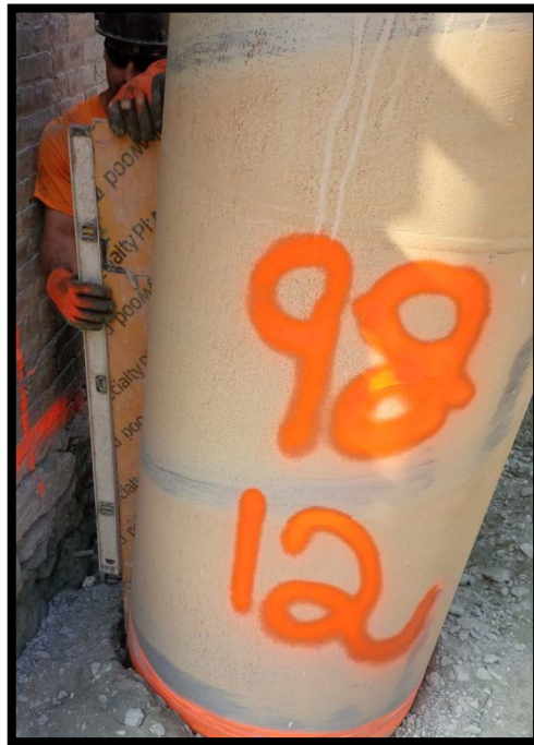
Photo 68: Battered secant pile #98S; confirming 6 degree tilt at EL +0 using a jig and bubble level.
