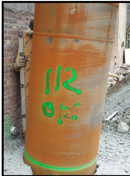
Photo 52: Battered secant pile #112S; confirming 6 degree tilt at EL +0 using a jig and bubble level.
