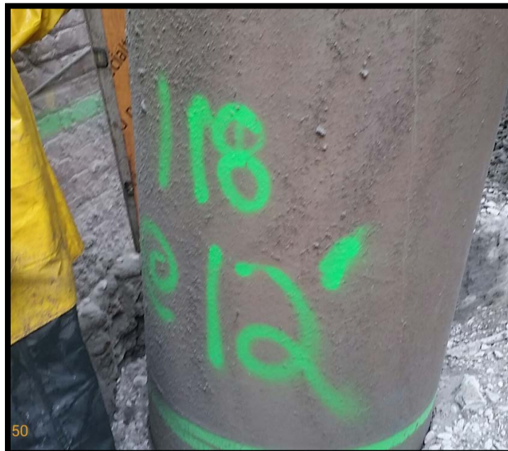
Photo 80: Battered secant pile #118S; confirming 6 degree tilt at EL +0 using a jig and bubble level.
