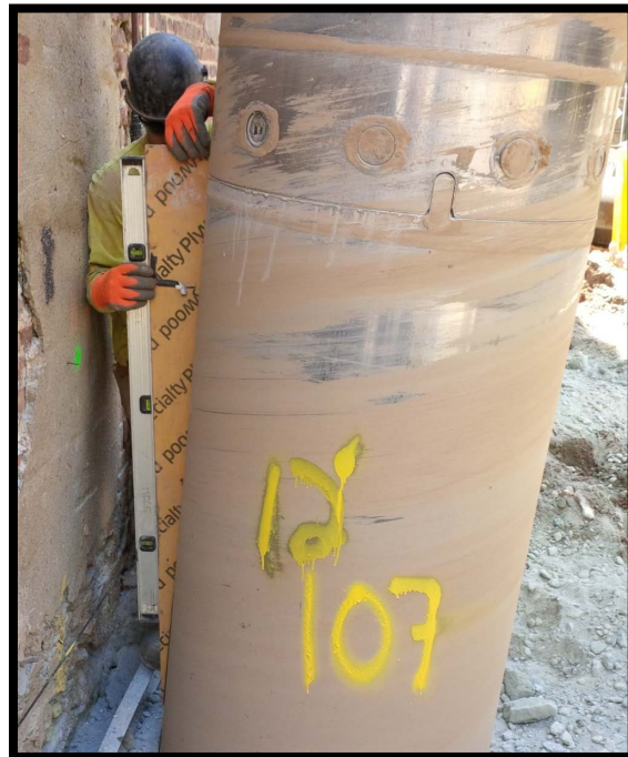
Photo 30: Battered secant pile #107P; confirming 6 degree tilt at EL +0 using a jig and bubble level.
