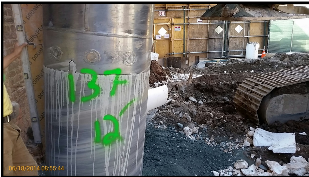
Photo 90: Battered secant pile #137P; confirming 6 degree tilt at EL +0 using a jig and bubble level.
