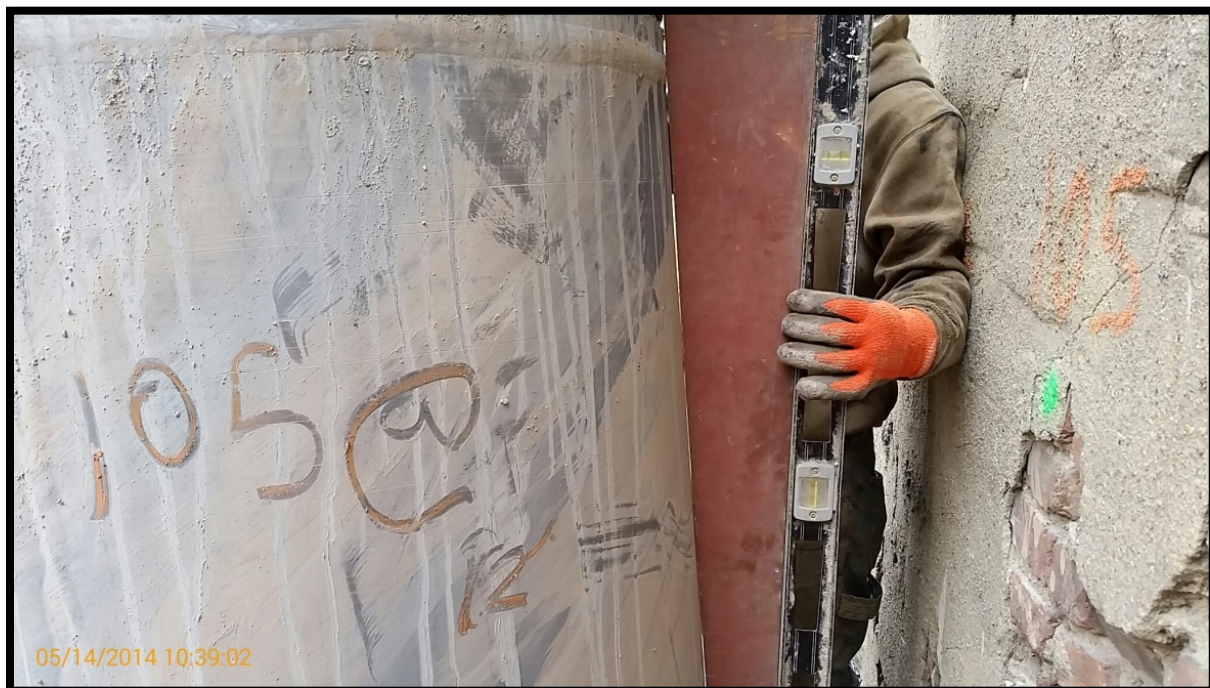
Photo 8: Battered secant pile #105P; confirming 6 degree tilt at EL +0 using a jig and bubble level.
