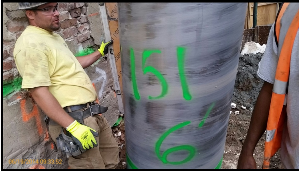
Photo 107: Battered secant pile #151P; confirming 6 degree tilt at EL +5 using a jig and bubble level.
