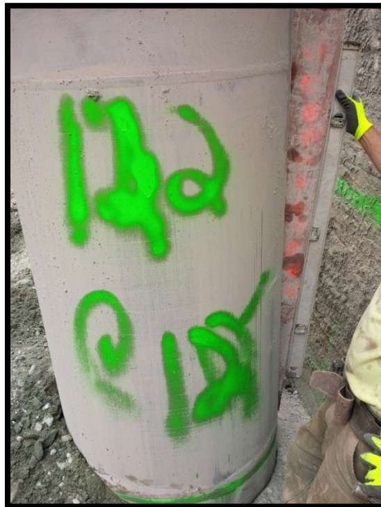
Photo 81: Battered secant pile #122S; confirming 6 degree tilt at EL +0 using a jig and bubble level.
