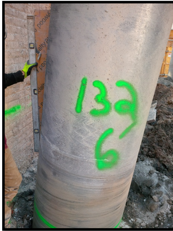
Photo 115: Battered secant pile #132S; confirming 6 degree tilt at EL +5 using a jig and bubble level.
