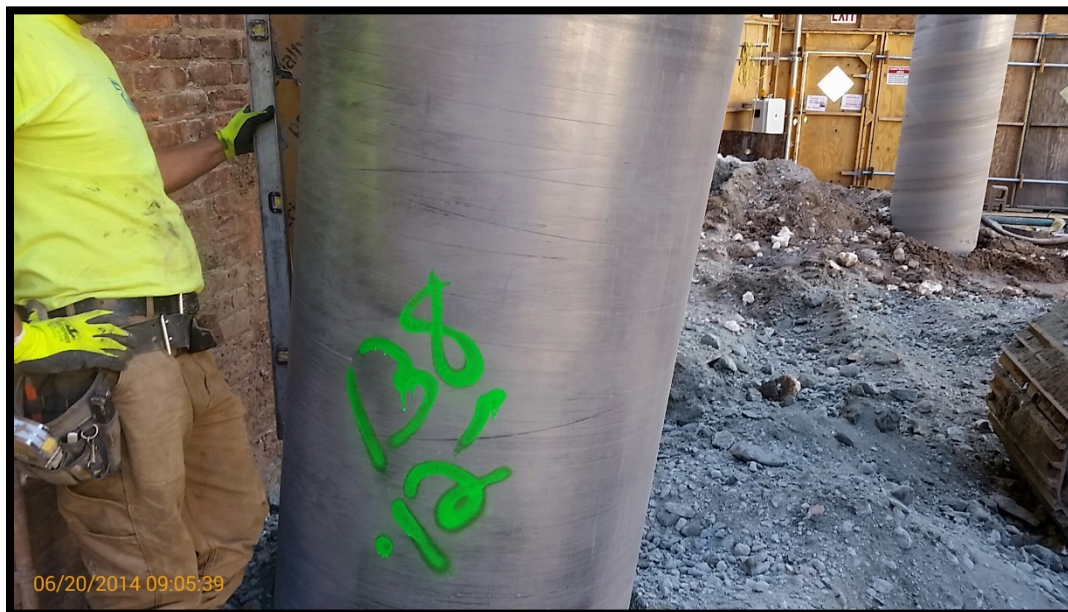
Photo 112: Battered secant pile #138S; confirming 6 degree tilt at EL +0 using a jig and bubble level.
