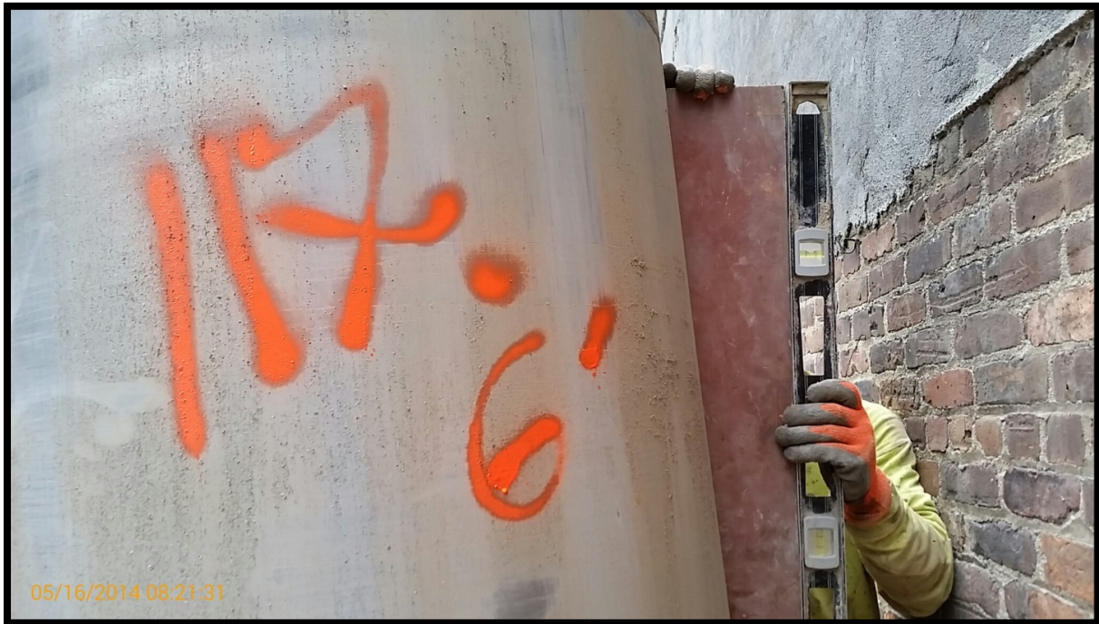
Photo 15: Battered secant pile #117P; confirming 6 degree tilt at EL +5 using a jig and bubble level.
