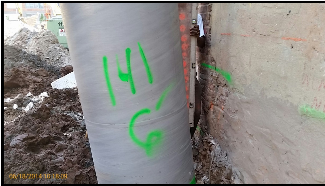
Photo 103: Battered secant pile #141P; confirming 6 degree tilt at EL +5 using a jig and bubble level.
