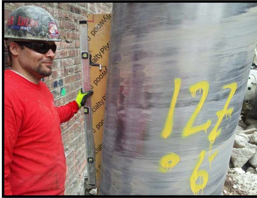
Photo 35: Battered secant pile #127P; confirming 6 degree tilt at EL +5 using a jig and bubble level.
