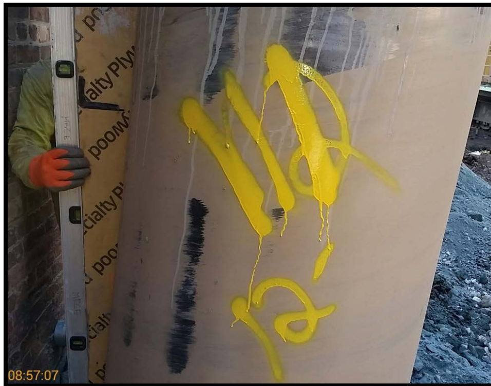
Photo 28: Battered secant pile #111P; confirming 6 degree tilt at EL +0 using a jig and bubble level.
