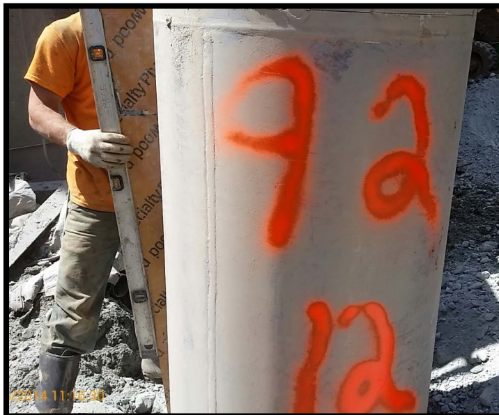
Photo 74: Battered secant pile #92S; confirming 6 degree tilt at EL +0 using a jig and bubble level.
