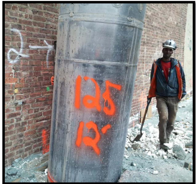
Photo 20A (left) & 20B (right): Battered secant pile #125P; confirming 6 degree tilt at EL +0 using a jig and bubble level.
