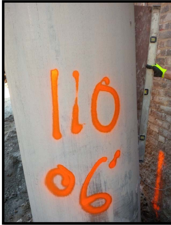
Photo 59: Battered secant pile #110S; confirming 6 degree tilt at EL +5 using a jig and bubble level.
