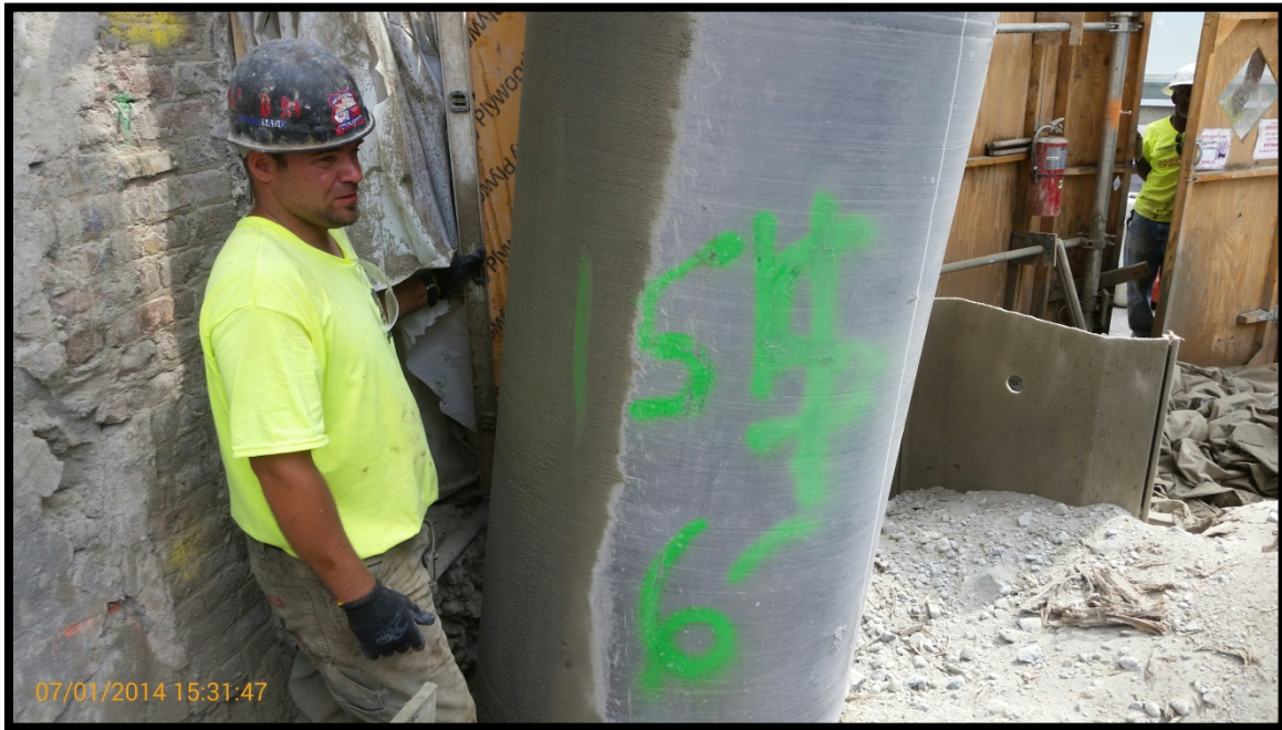
Photo 131: Battered secant pile #154S; confirming 6 degree tilt at EL +5 using a jig and bubble level.
