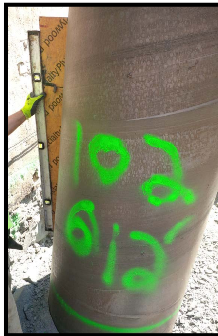
Photo 66: Battered secant pile #102S; confirming 6 degree tilt at EL +0 using a jig and bubble level.
