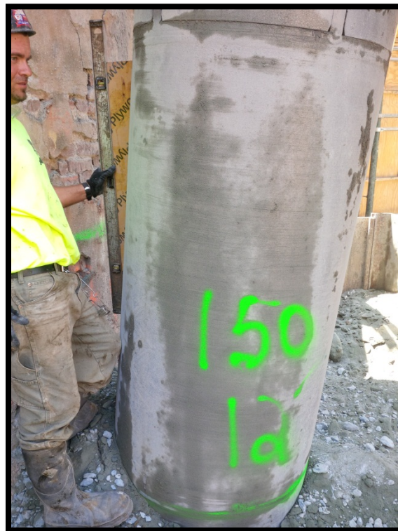
Photo 130: Battered secant pile #150S; confirming 6 degree tilt at EL +0 using a jig and bubble level.
