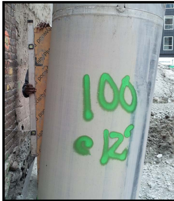
Photo 50: Battered secant pile #100S; confirming 6 degree tilt at EL +0 using a jig and bubble level.
