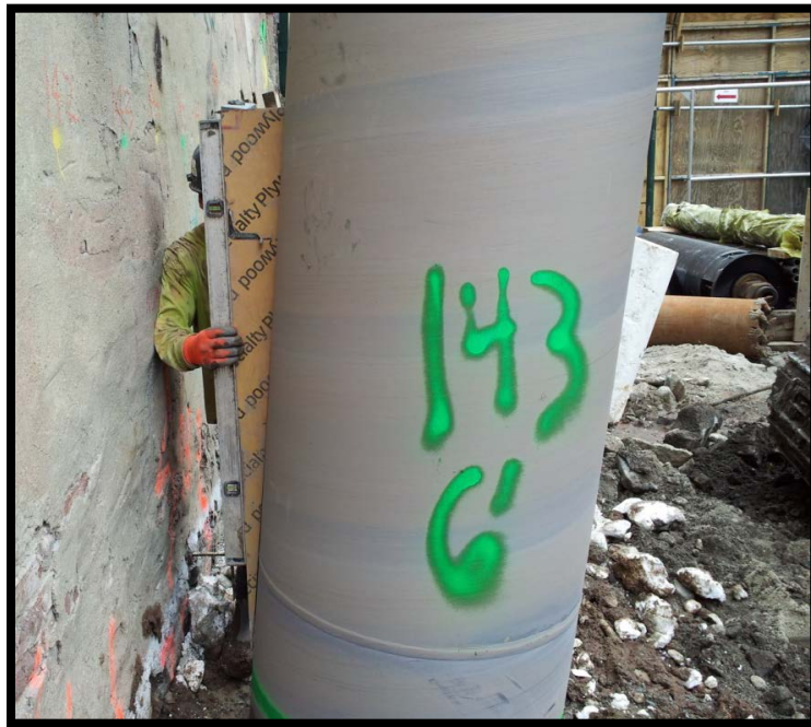
Photo 43: Battered secant pile #143P; confirming 6 degree tilt at EL +5 using a jig and bubble level.
