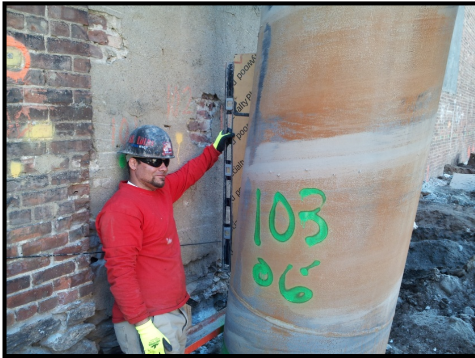
Photo 23: Battered secant pile #103P; confirming 6 degree tilt at EL +5 using a jig and bubble level.
