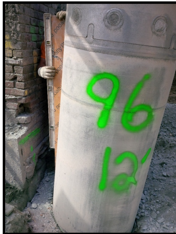
Photo 76: Battered secant pile #96S; confirming 6 degree tilt at EL +0 using a jig and bubble level.
