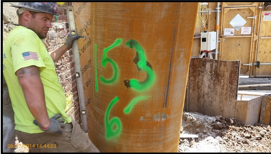
Photo 99: Battered secant pile #153P; confirming 6 degree tilt at EL +5 using a jig and bubble level.
