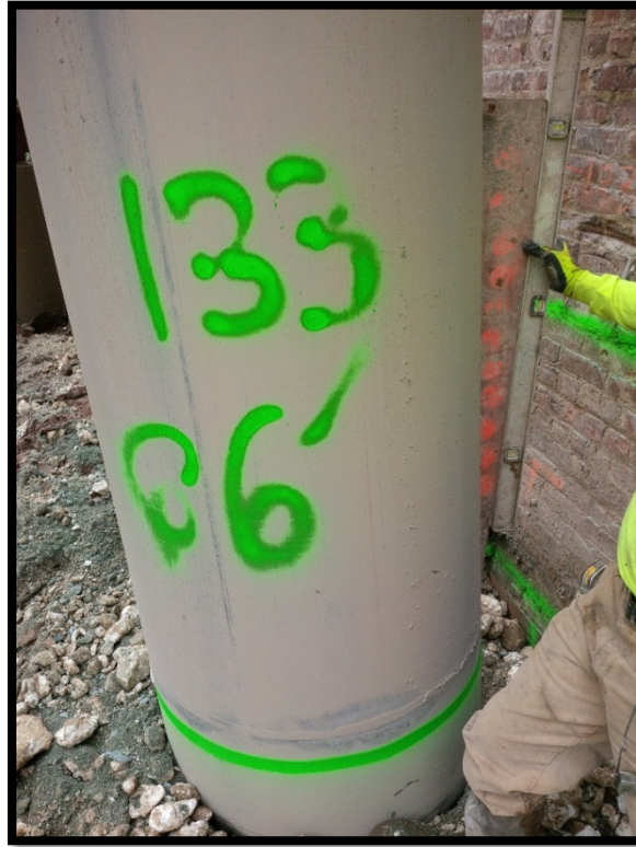
Photo 87: Battered secant pile #133P; confirming 6 degree tilt at EL +5 using a jig and bubble level.
