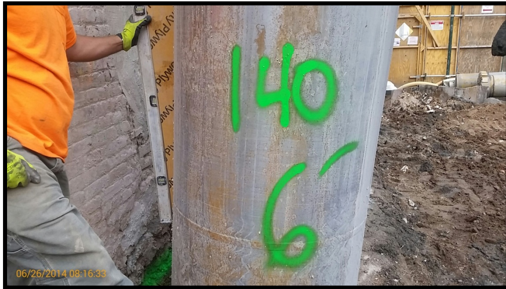
Photo 125: Battered secant pile #140S; confirming 6 degree tilt at EL +5 using a jig and bubble level.
