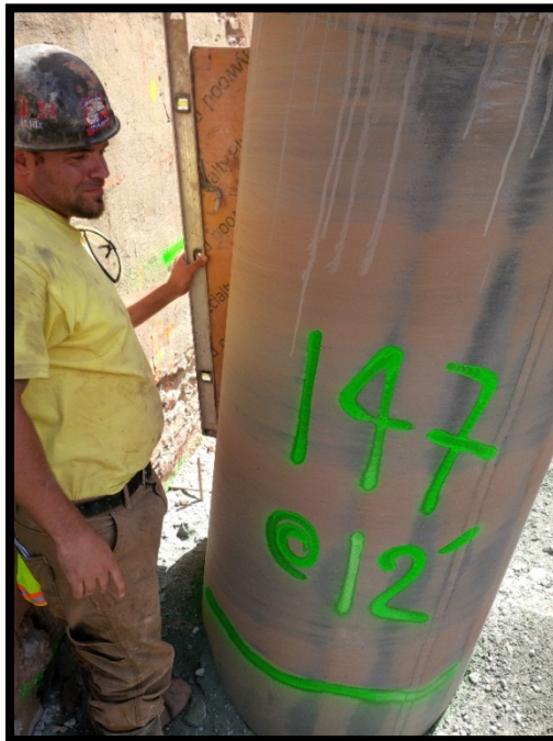
Photo 102: Battered secant pile #147P; confirming 6 degree tilt at EL +0 using a jig and bubble level.
