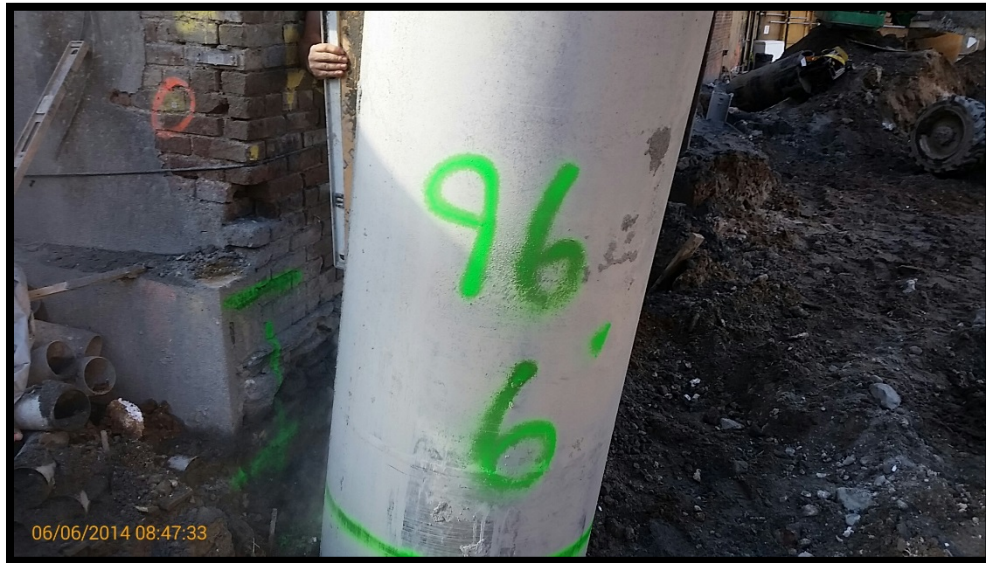
Photo 75: Battered secant pile #96S; confirming 6 degree tilt at EL +5 using a jig and bubble level.
