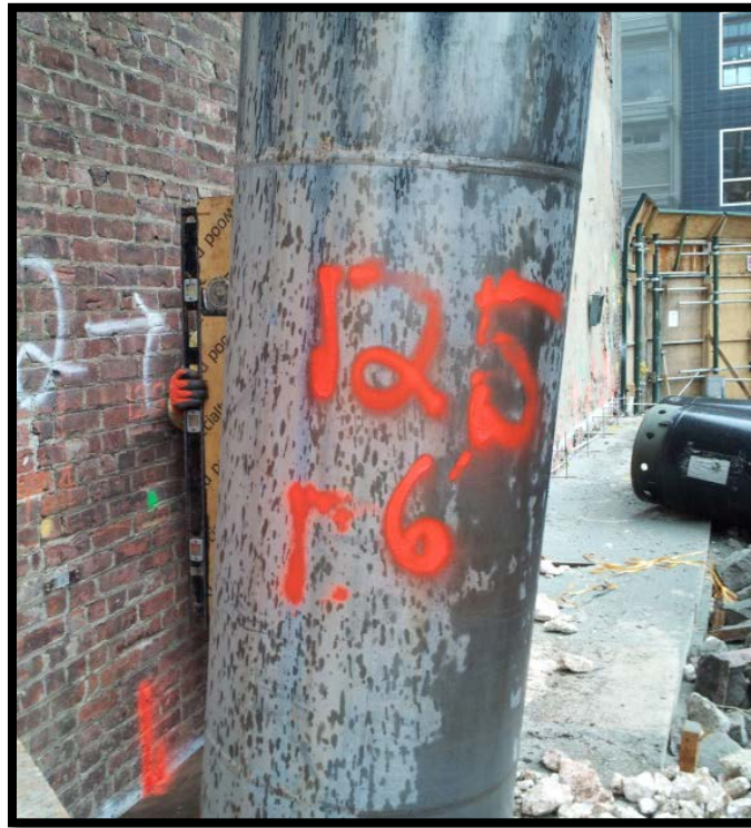
Photo 19: Battered secant pile #125P; confirming 6 degree tilt at EL +5 using a jig and bubble level.
