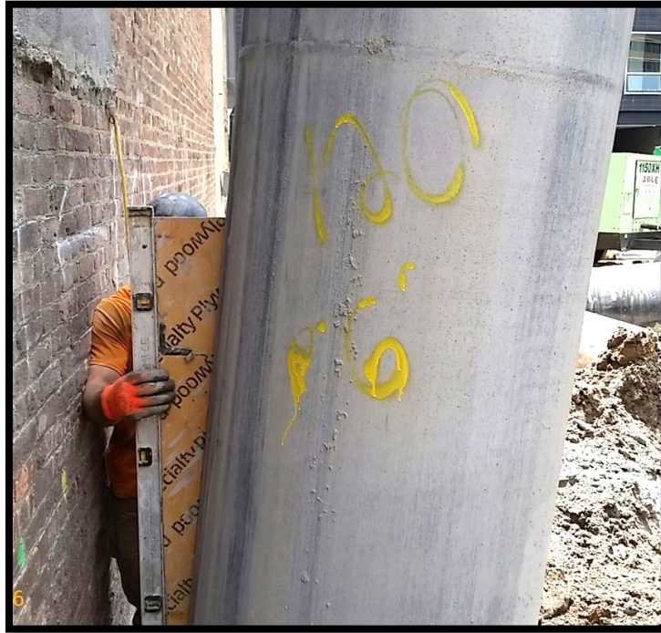
Photo 57: Battered secant pile #120S; confirming 6 degree tilt at EL +5 using a jig and bubble level.
