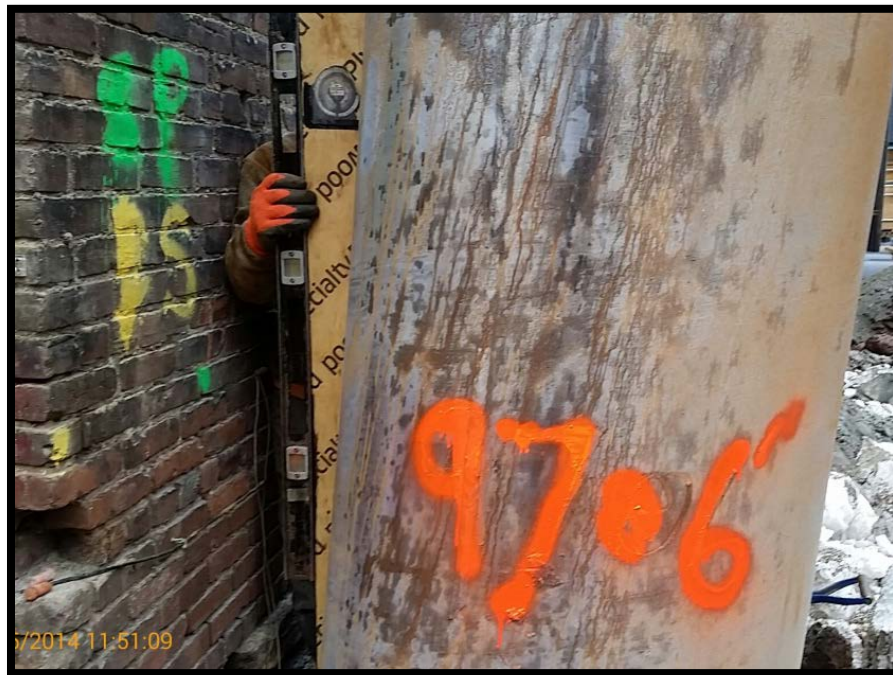
Photo 9: Battered secant pile #97P: confirming 6 degree tilt at EL +5 using a jig and bubble level.
