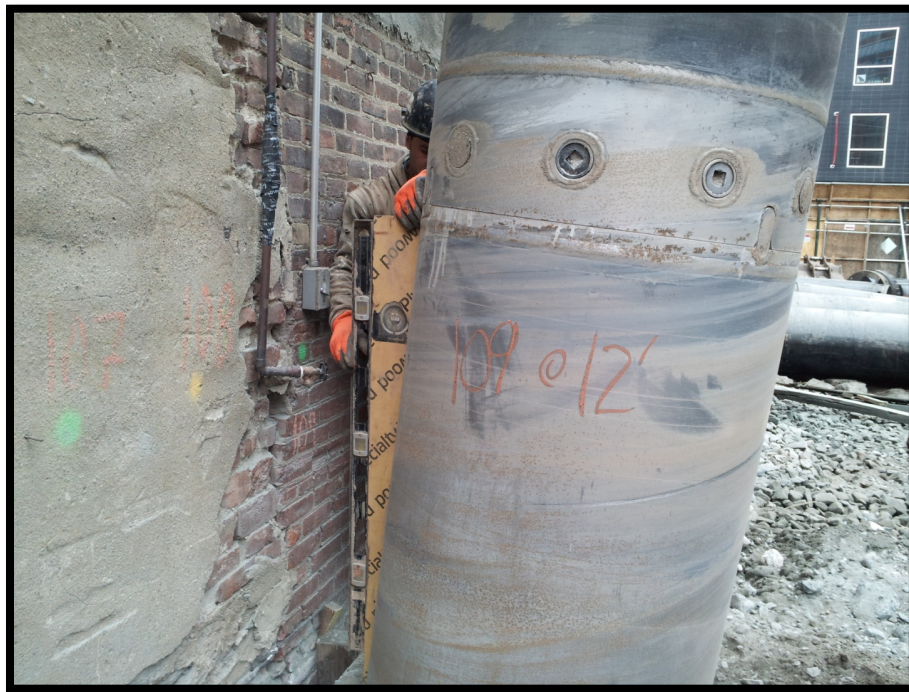
Photo 12: Battered secant pile #109P; confirming 6 degree tilt at EL +0 using a jig and bubble.
