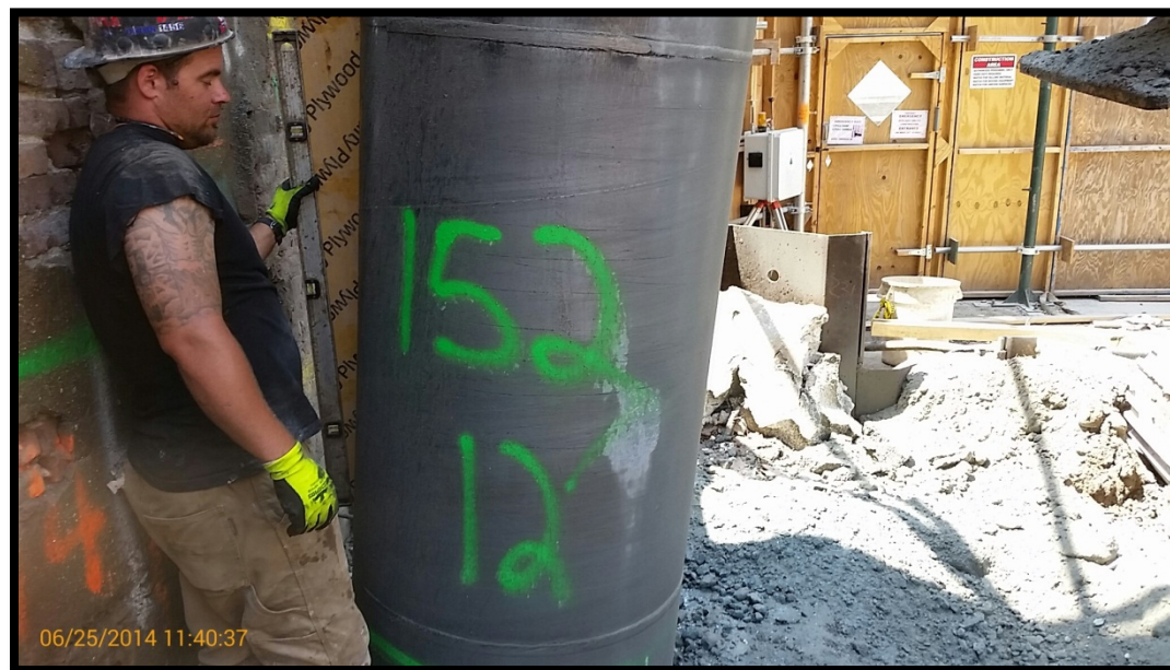
Photo 122: Battered secant pile #152S; confirming 6 degree tilt at EL +0 using a jig and bubble level.
