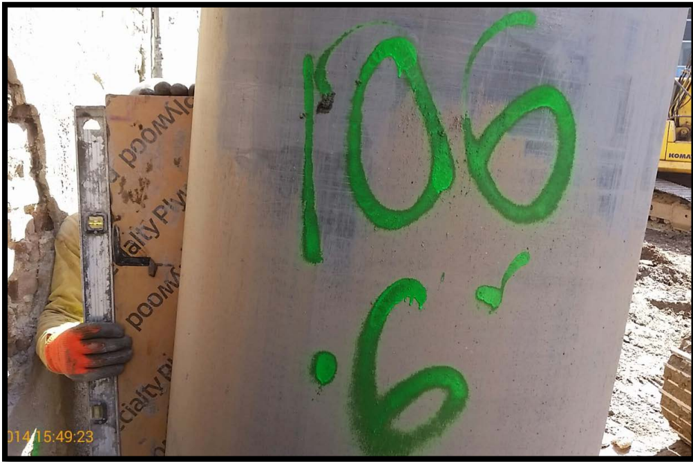
Photo 53: Battered secant pile #106S; confirming 6 degree tilt at EL +5 using a jig and bubble level.
