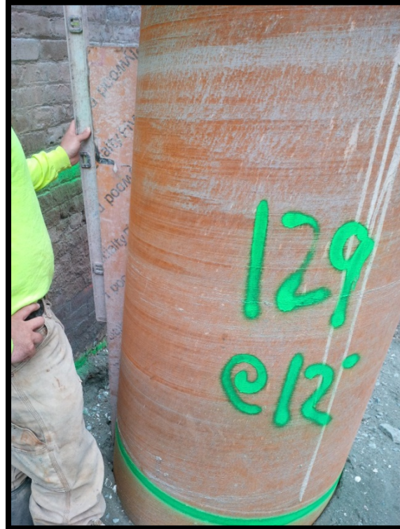
Photo 86: Battered secant pile #129P; confirming 6 degree tilt at EL +0 using a jig and bubble level.
