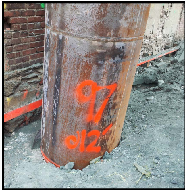
Photo 10A (left) & 10B (right): Battered secant pile #97P; confirming 6 degree tilt at EL +0 using a jig and bubble level.
