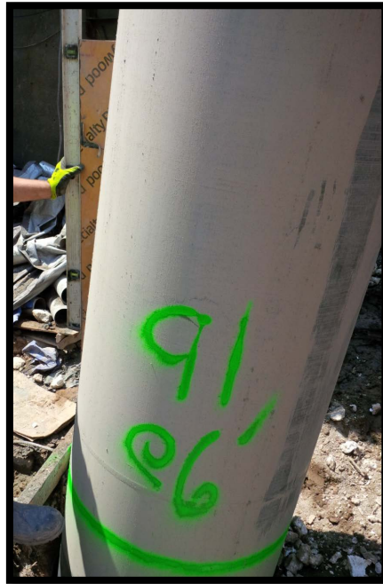
Photo 61: Battered secant pile #91P; confirming 6 degree tilt at EL +5 using a jig and bubble level.
