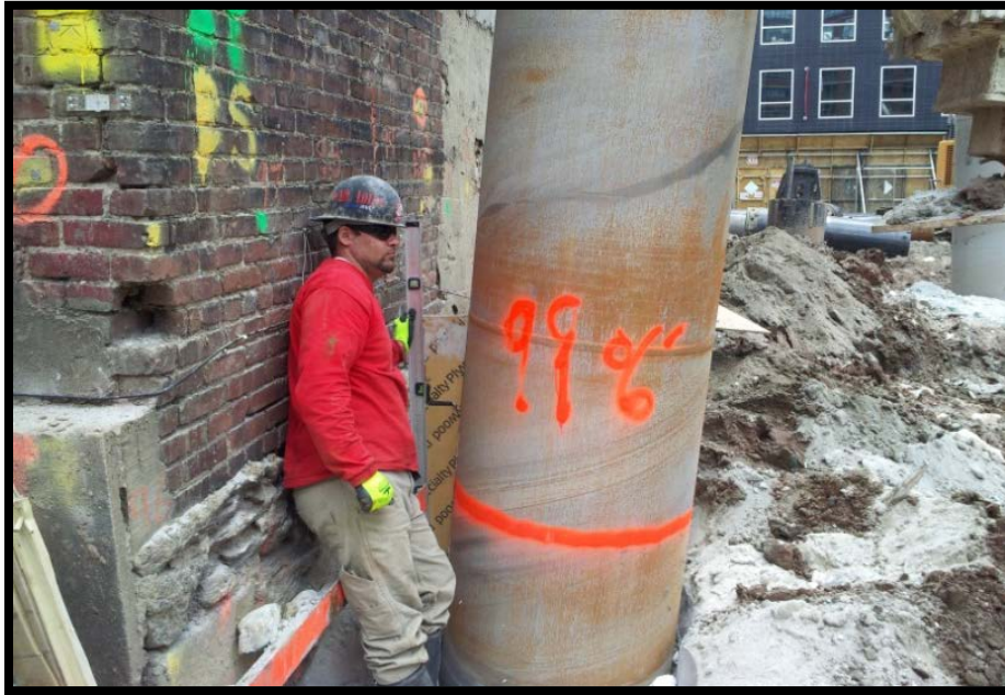
Photo 21: Battered secant pile #99P; confirming 6 degree tilt at EL +5 using a jig and bubble level.
