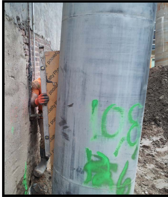
Photo 47: Battered secant pile #108S; confirming 6 degree tilt at EL +5 using a jig and bubble level.
