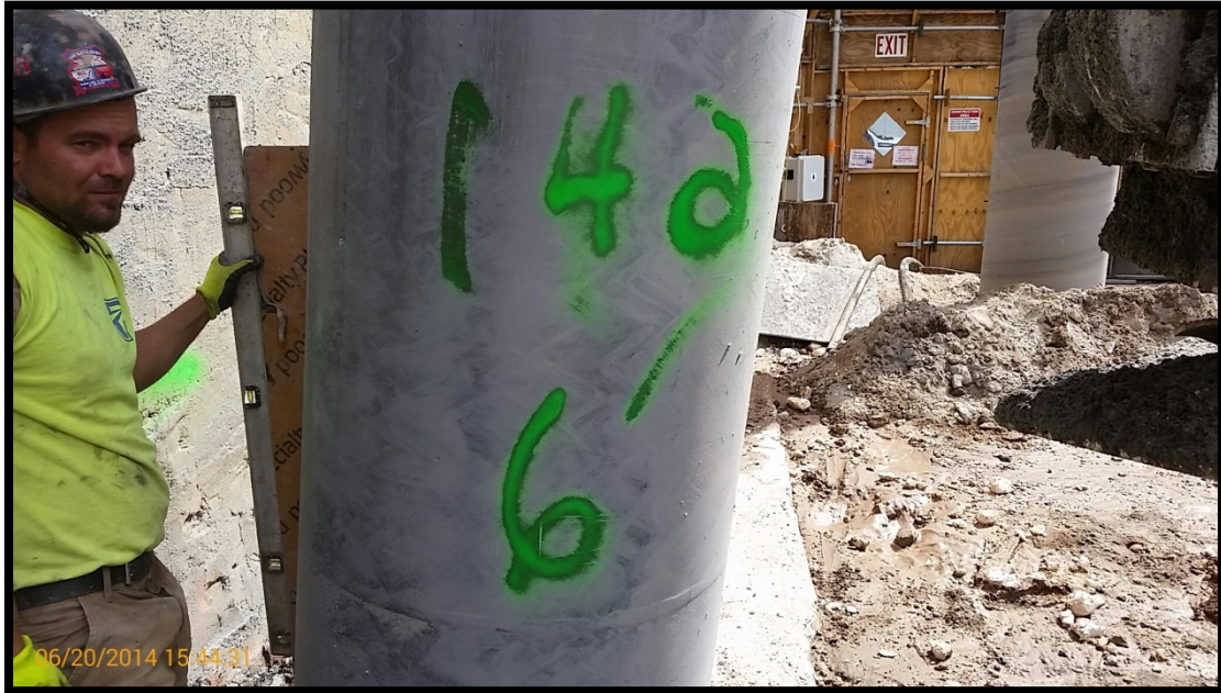
Photo 113: Battered secant pile #142S; confirming 6 degree tilt at EL +5 using a jig and bubble level.
