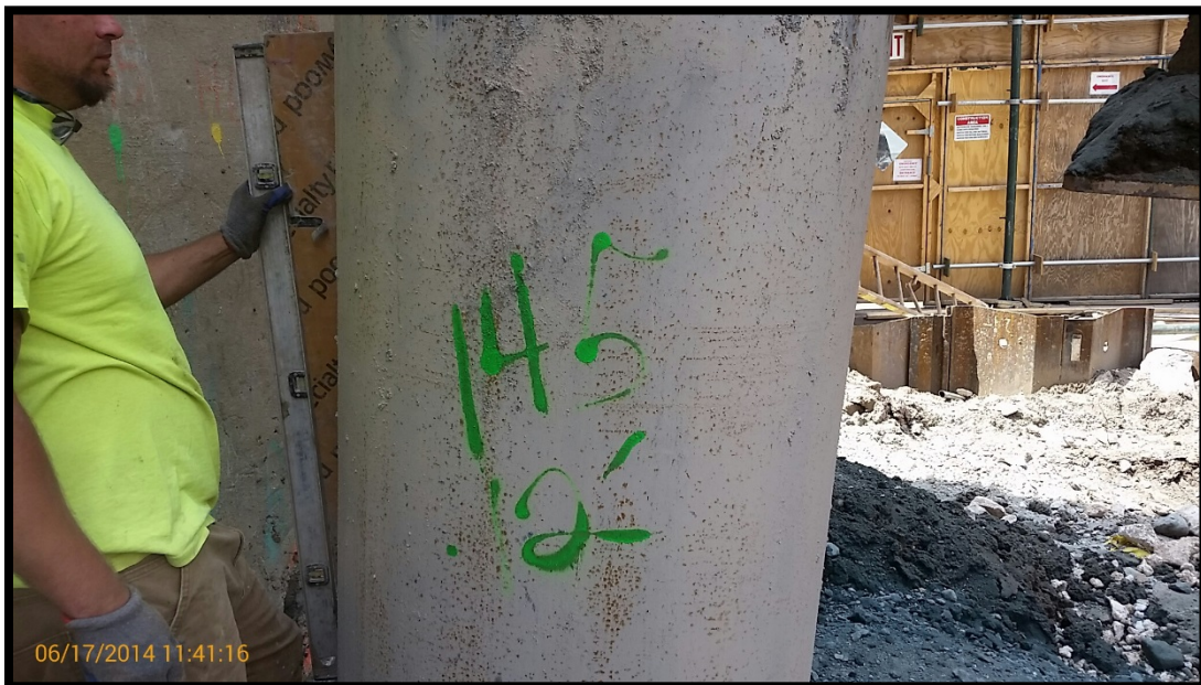
Photo 96: Battered secant pile #145P; confirming 6 degree tilt at EL +0 using a jig and bubble level.
