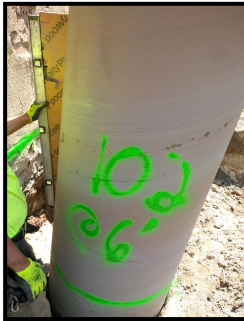
Photo 65: battered secant pile #102S; confirming 6 degree tilt at 6 EL +5 using a jig and bubble level.
