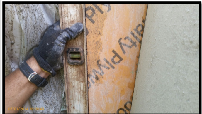
Photo 132A (left) & 132B (right): Battered secant pile #154S; confirming 6 degree tilt at EL +0 using a jig and bubble level.
