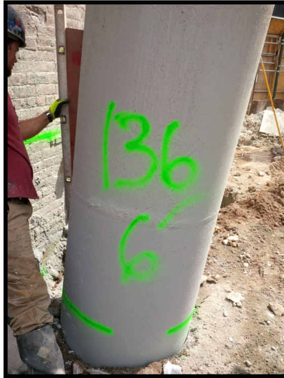
Photo 117: Battered secant pile #136S; confirming 6 degree tilt at EL +5 using a jig and bubble level.
