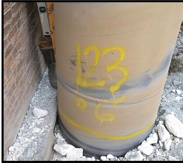
Photo 33: Battered secant pile #123; confirming 6 degree tilt at EL +5 using a jig and bubble level.
