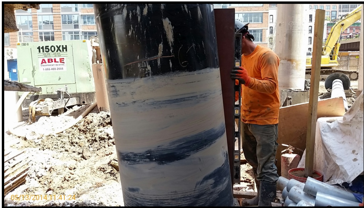
Photo 3: Battered secant pile #93P; confirming 6 degree tilt at EL +5 using a jig and bubble level.
