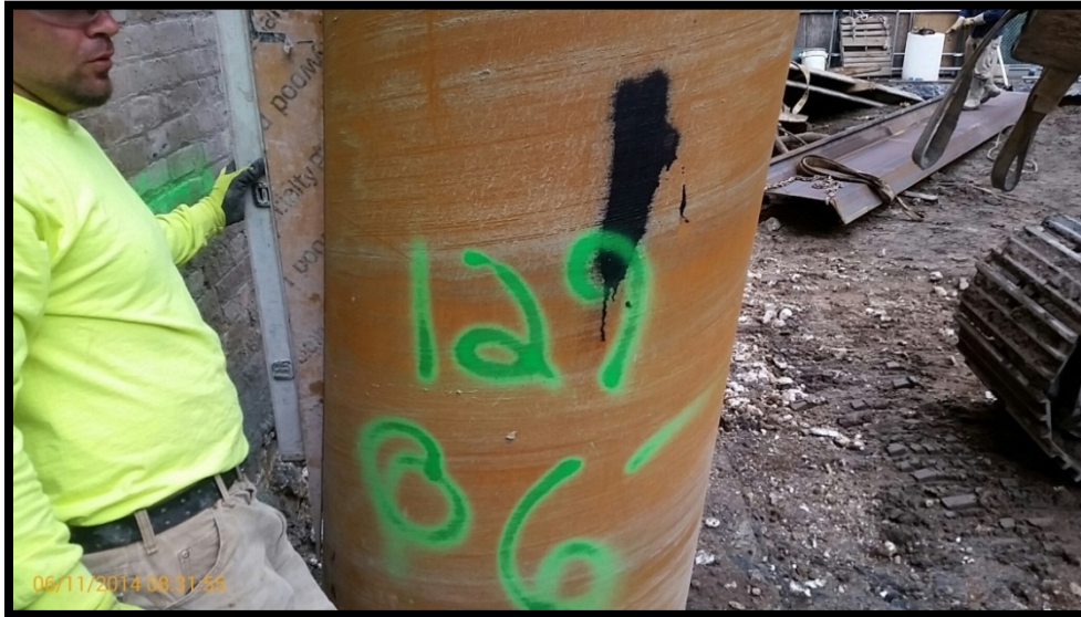
Photo 85: Battered secant pile #129P; confirming 6 degree tilt at EL +5 using a jig and bubble level.
