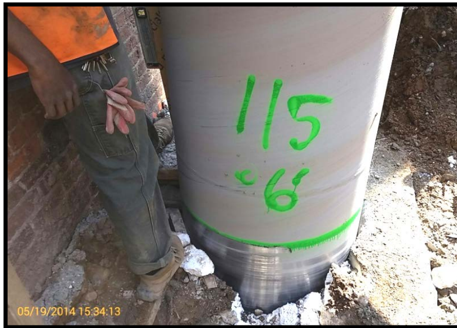
Photo 25: Battered secant pile #115P; confirming 6 degree tilt at EL +5 using a jig and bubble level.
