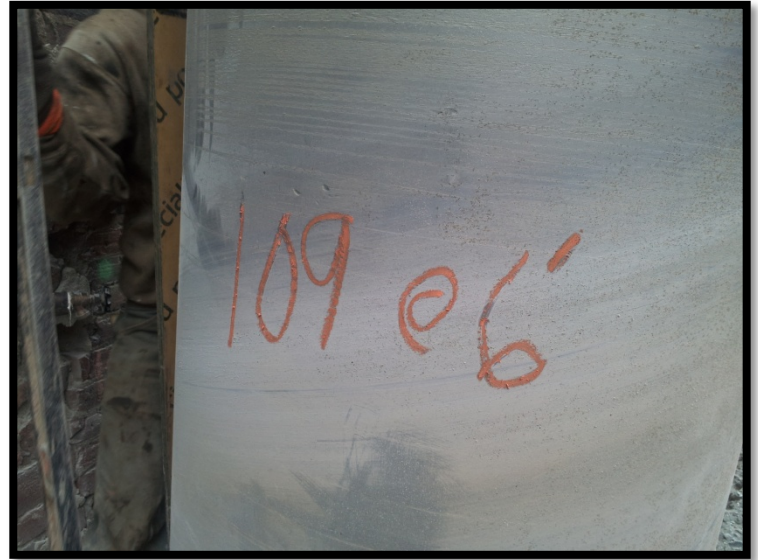
Photo 11A (left ) & 11B (right): Battered secant pile #109P; confirming 6 degree tilt at EL +5 using a jig and bubble level.
