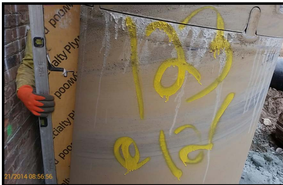
Photo 34: Battered secant pile #123P; confirming 6 degree tilt at EL +0 using a jig and bubble level.
