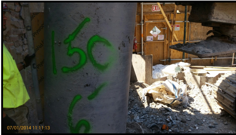
Photo 129: Battered secant pile #150S; confirming 6 degree tilt at EL +5 using a jig and bubble level.
