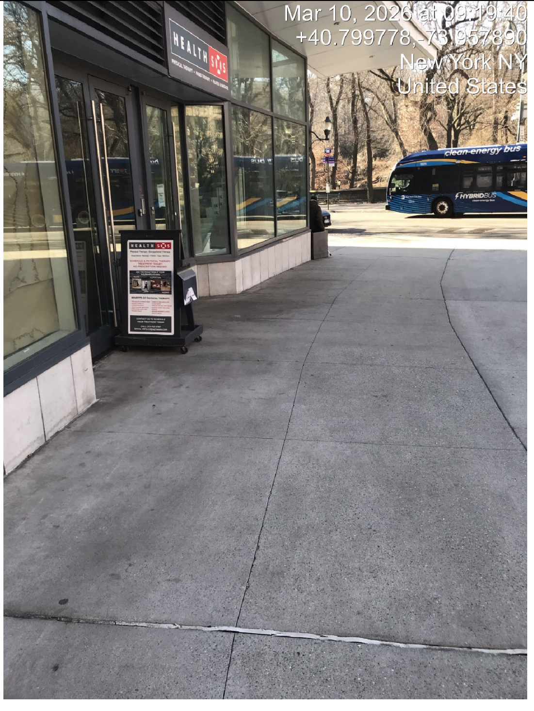
Photo 3 – Sidewalk outside at grade level
