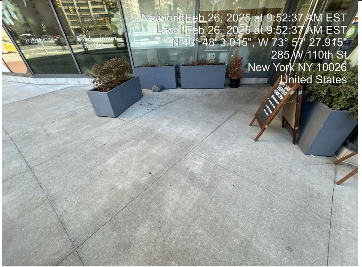
Photo 3 – Sidewalk outside at grade level
