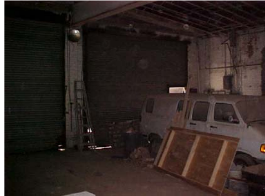
Interior of garage building.
