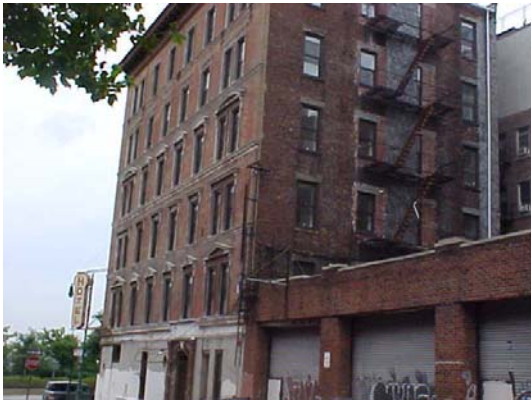
Subject property – six story hotel (150 Barrow Street) and single story garage building (144-148 Barrow Street).
