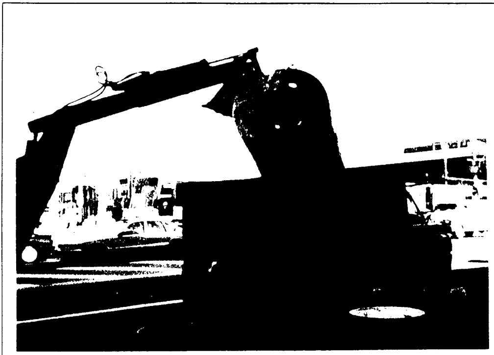
VIEW OF TANK BEING CUT, CLEANED AND READY FOR TRANSPORT
