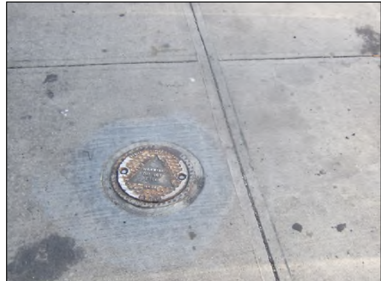
Photograph 8. A groundwater monitoring well in the Ninth Avenue sidewalk west-adjacent to the Property.
