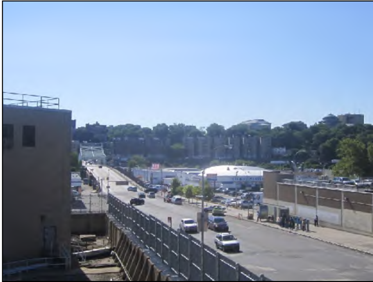
Photograph 9. The University Heights bridge approach southwest of the Property, view east.
