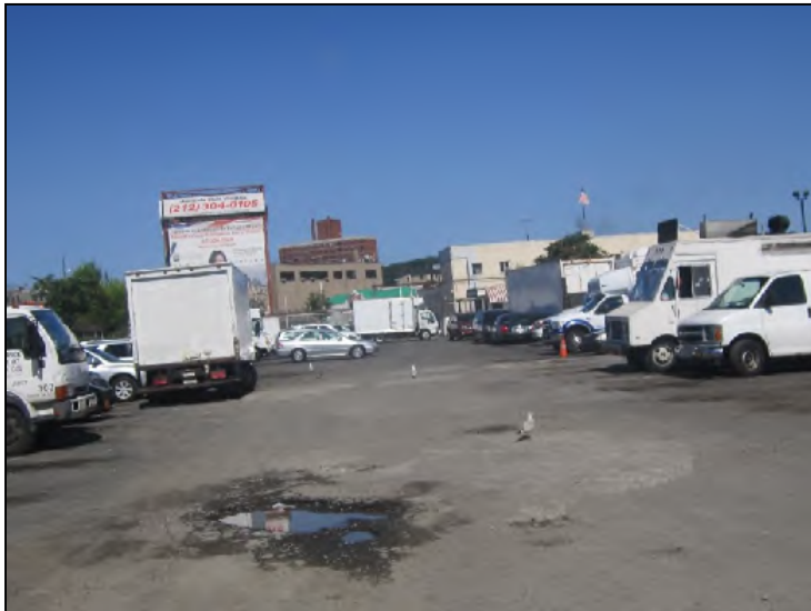
Photograph 3. The Property, view west. Note an area of pitted pavement in the foreground.
