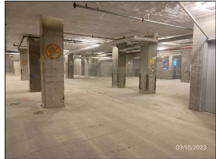
Photograph 2: Interior of the Controlled Property.
