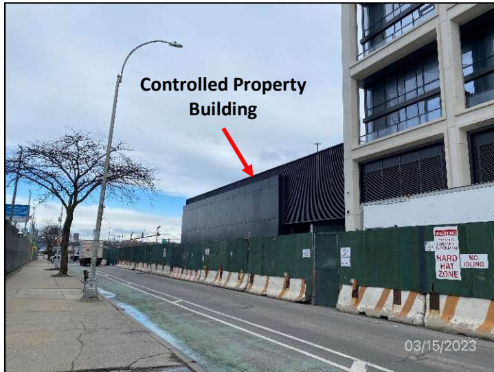
Photograph 1: Exterior of the Controlled Property building as seen from West 29 th Street.
