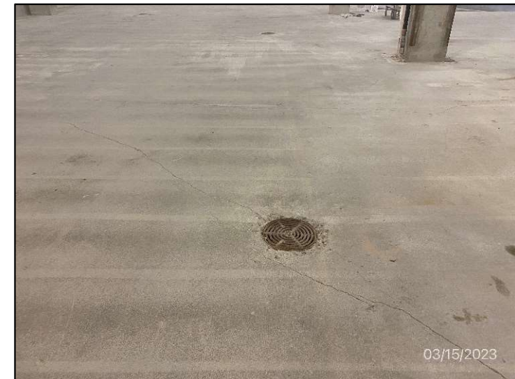
Photograph 4: Controlled Building slab.
