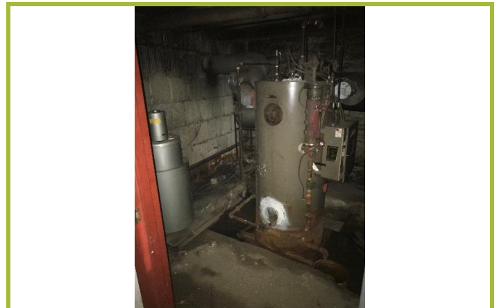
Photo #12: Former drycleaner boiler room located in the basement.
