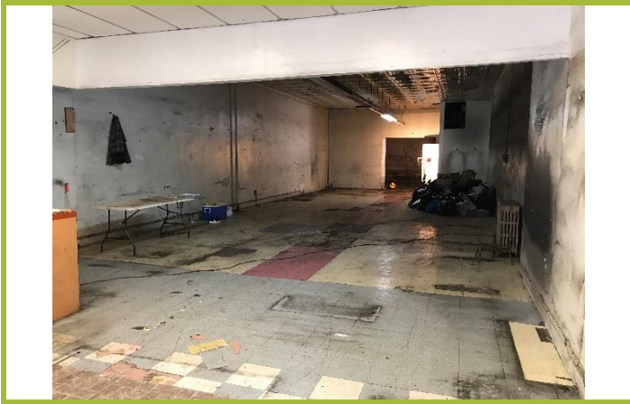
Photo #1: Eastern-facing interior on the 1 st floor of the site.
