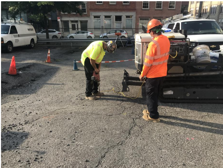
Photo 2: AARCO installing sub-slab vapor probe at Void 1 (facing south)
