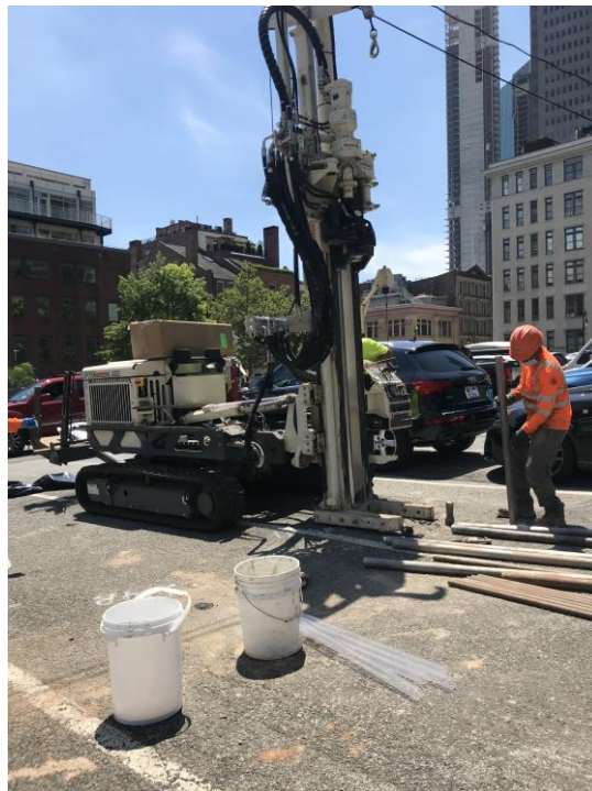
Photo 1: AARCO advancing soil boring SB4W1 (facing southwest)
