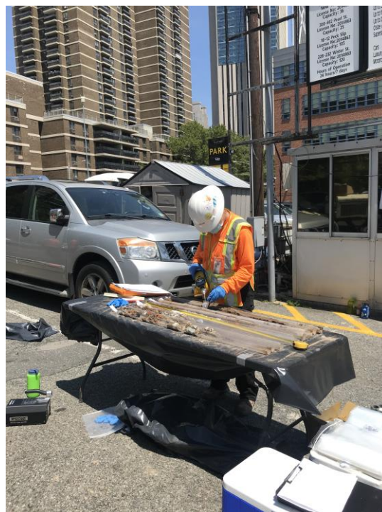
Photo 2: Langan collecting VOC readings from a soil boring (facing northeast)
