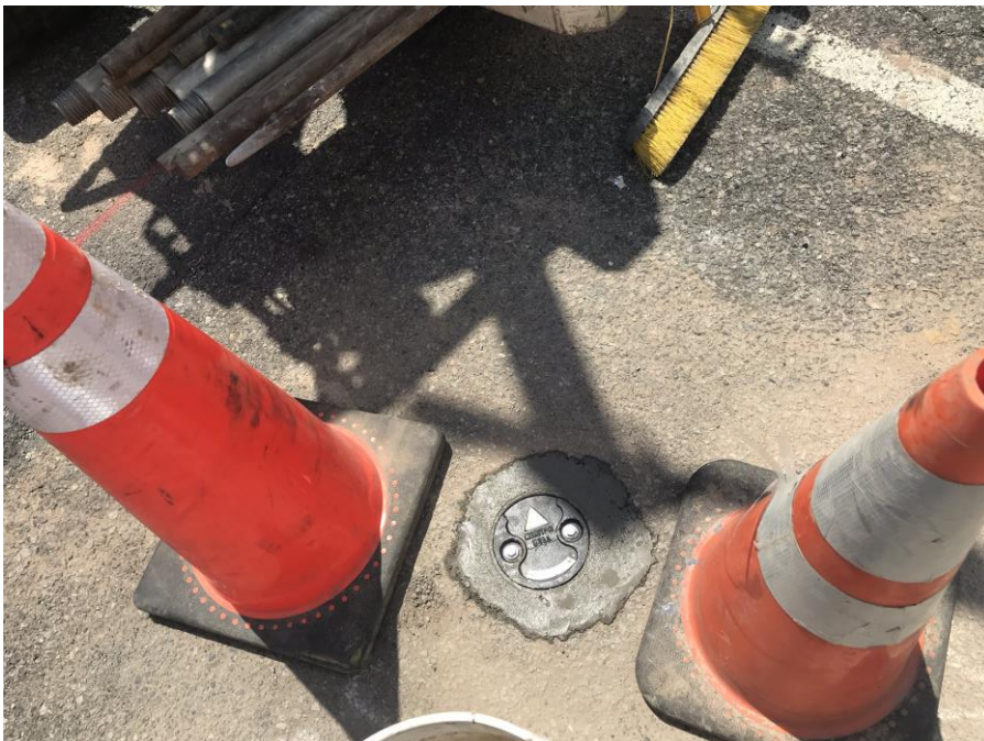
Photo 2: Monitoring well MW25 installed by AARCO
