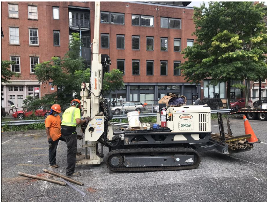
Photo 1: AARCO advancing soil boring SB17 in the southern part of the site (facing south)
