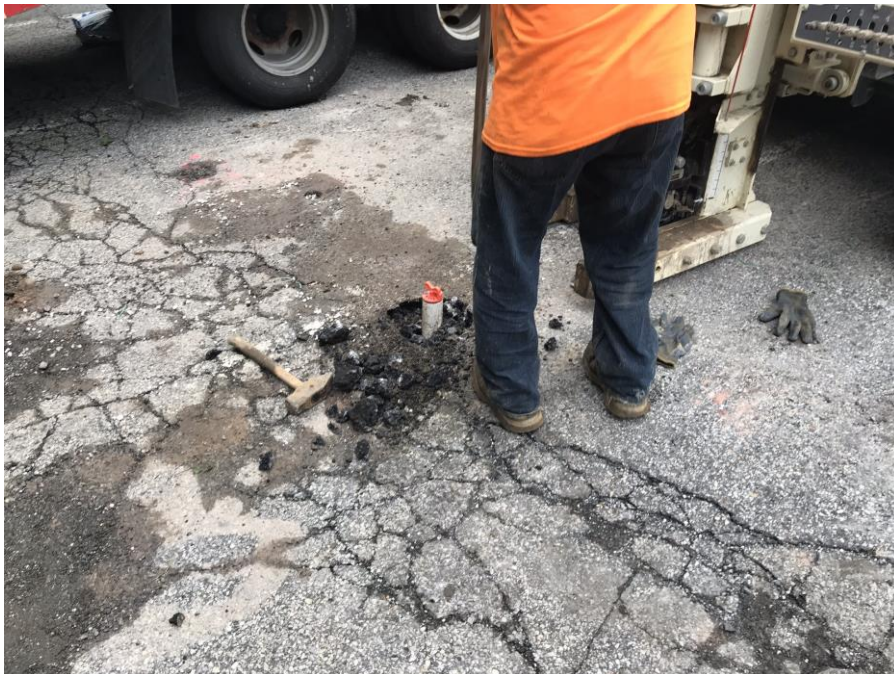
Photo 2: AARCO installing monitoring well MW17 (facing northwest)
