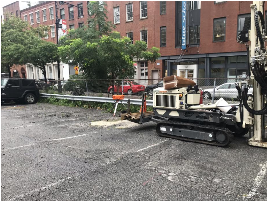
Photo 4: AARCO advancing SB-23 (facing southeast)
