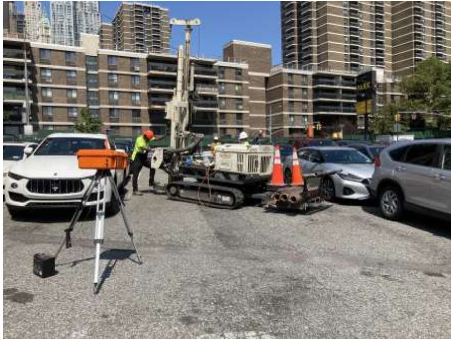
Photo 3: AARCO drilling boring SB36 (facing northwest).
