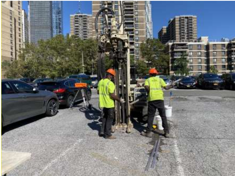
Photo 4: AARCO drilling boring SB22 (facing northeast).
