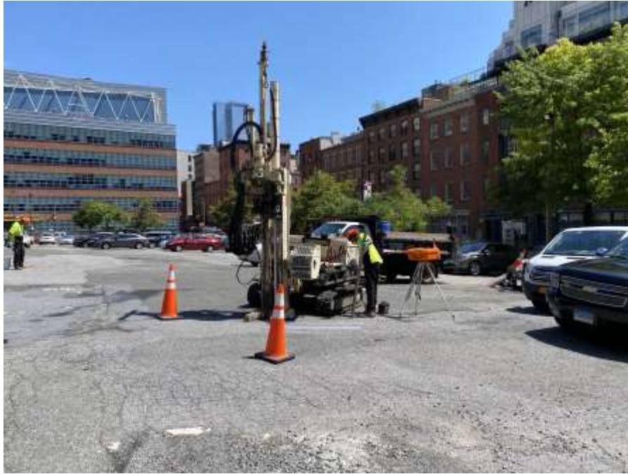
Photo 3: AARCO drilling boring SB16 (facing east).
