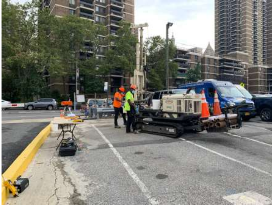
Photo 3: AARCO drilling boring SB15 (facing northwest).
