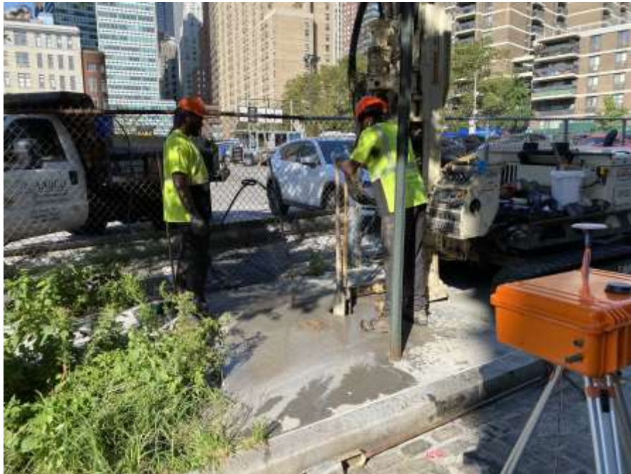
Photo 4: AARCO attempting to hand clear boring SB34 (facing west)
