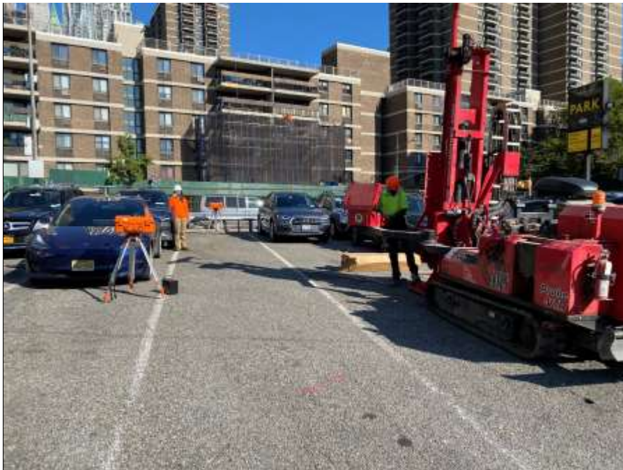
Photo 2: CAMP station WZ-1 and perimeter CAMP station PM-4 along Pearl Street during the drilling of boring SB36 (facing northwest)
