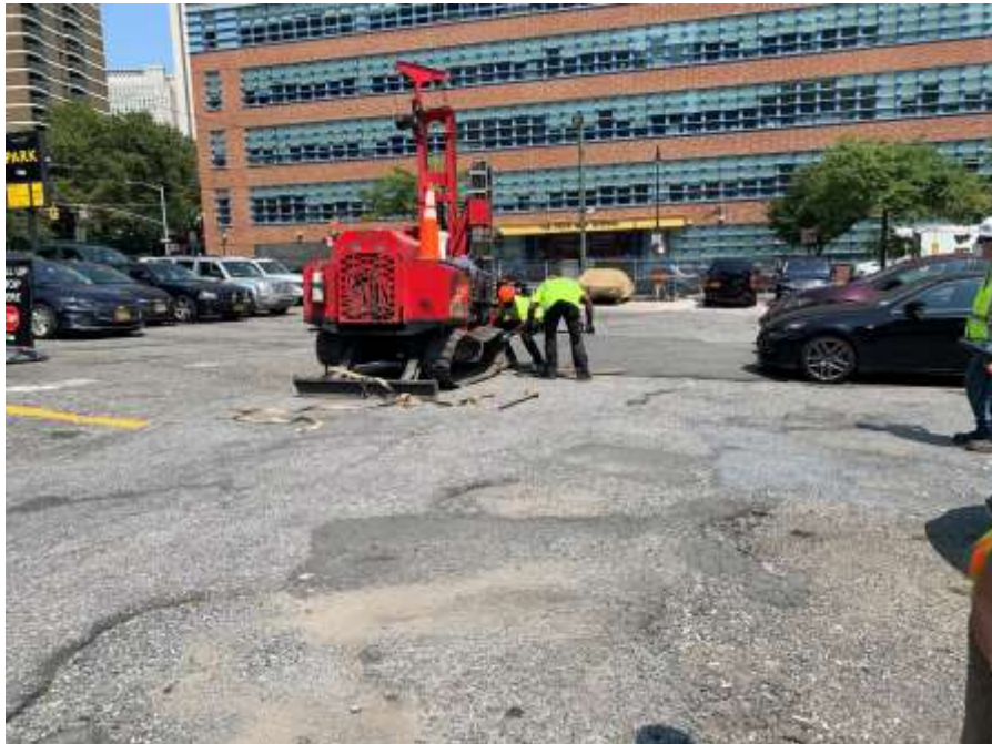
Photo 4: AARCO troubleshooting drill rig track (facing north)
