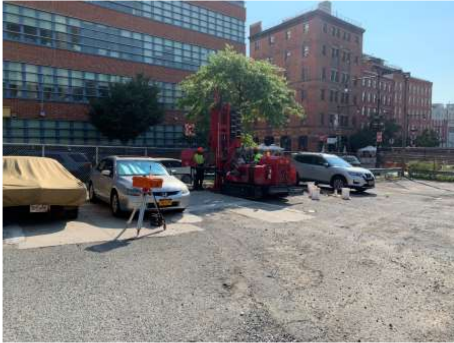
Photo 3: AARCO drilling boring SB34 (facing east)
