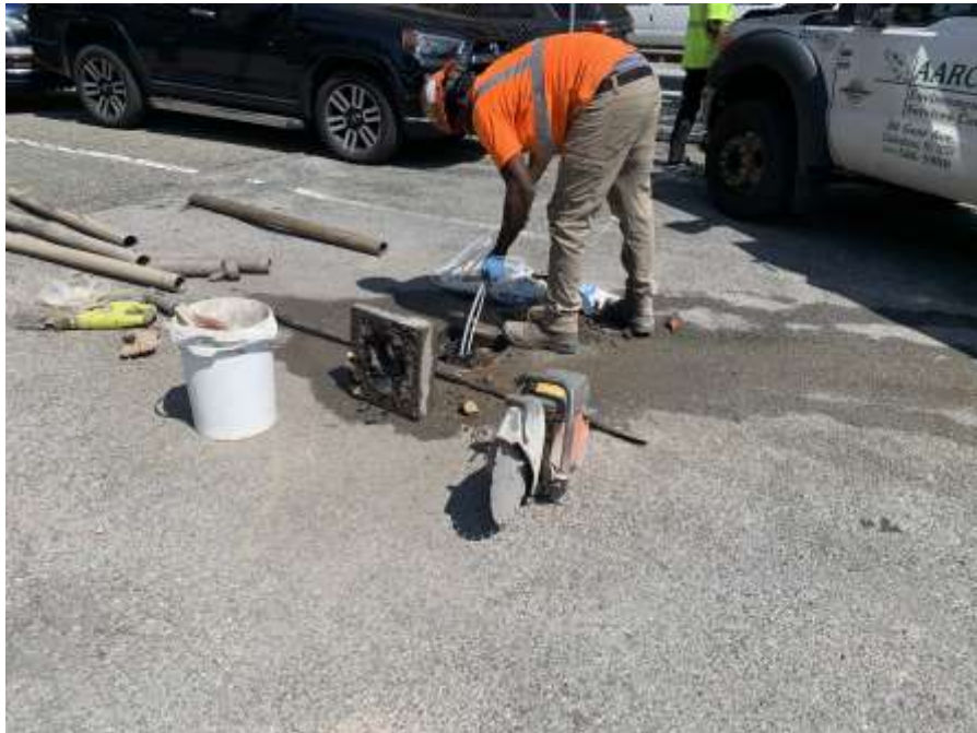
Photo 4: AARCO developing monitoring well MW30 (facing north)
