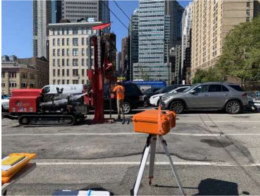
Photo 3: AARCO drilling boring SB4W3 (facing southwest)
