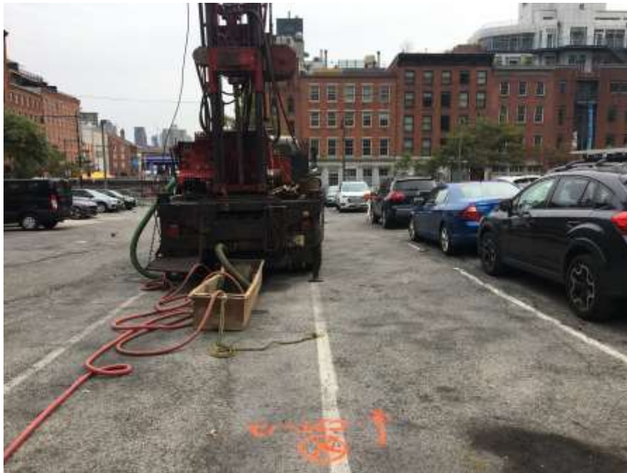
Photo 2: View of Warren George, Inc. predrilling CPT location CPT-12 (facing east).
