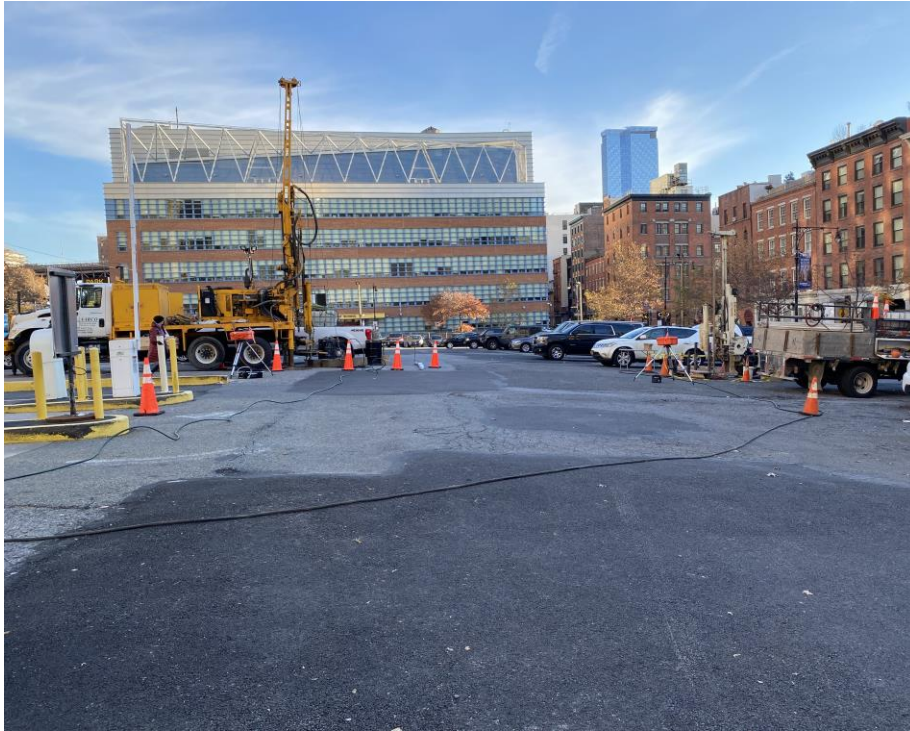
Photo 1: View of AARCO drilling LB-2 and LB-9 (facing northwest).
