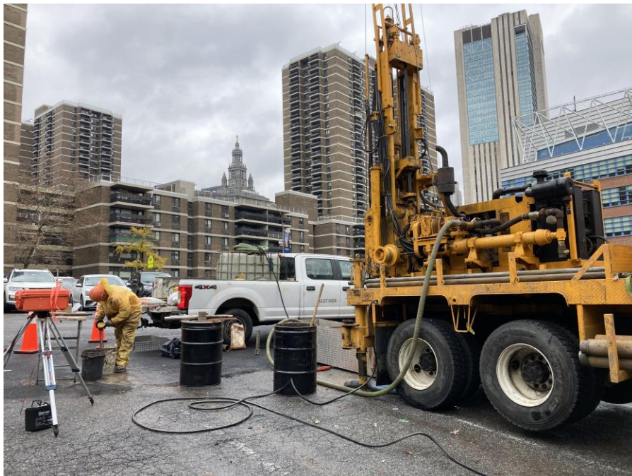
Photo 2: View of AARCO drilling at LB-8 (facing northeast).
