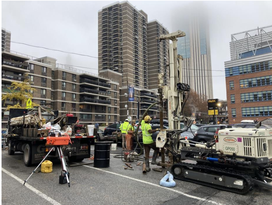
Photo 1: View of AARCO drilling at LB-3 (facing northeast).
