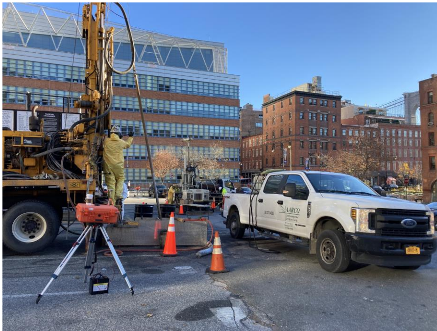
Photo 1: View of AARCO drilling at LB-7 and LB-13 (facing east).
