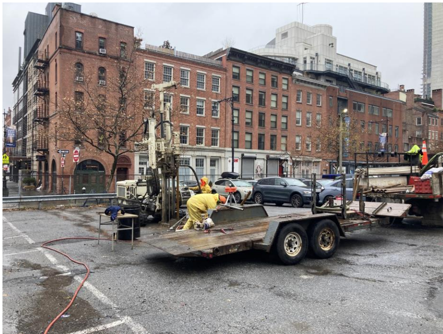
Photo 2: View of AARCO drilling at LB-6 (facing southwest).
