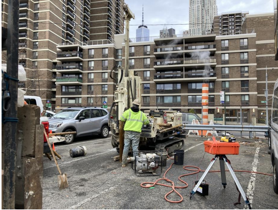
Photo 1: View of AARCO drilling at LB-5 (facing north).
