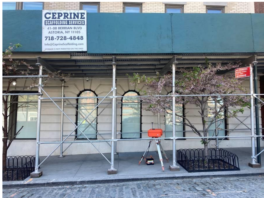
Photo 2: View of perimeter CAMP station PM-2, relocated to the eastern sidewalk of Beekman Street (facing west)
