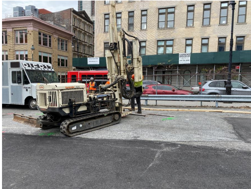
Photo 1: View of AARCO advancing a delineation soil boring in the southwestern portion of the site (facing west).
