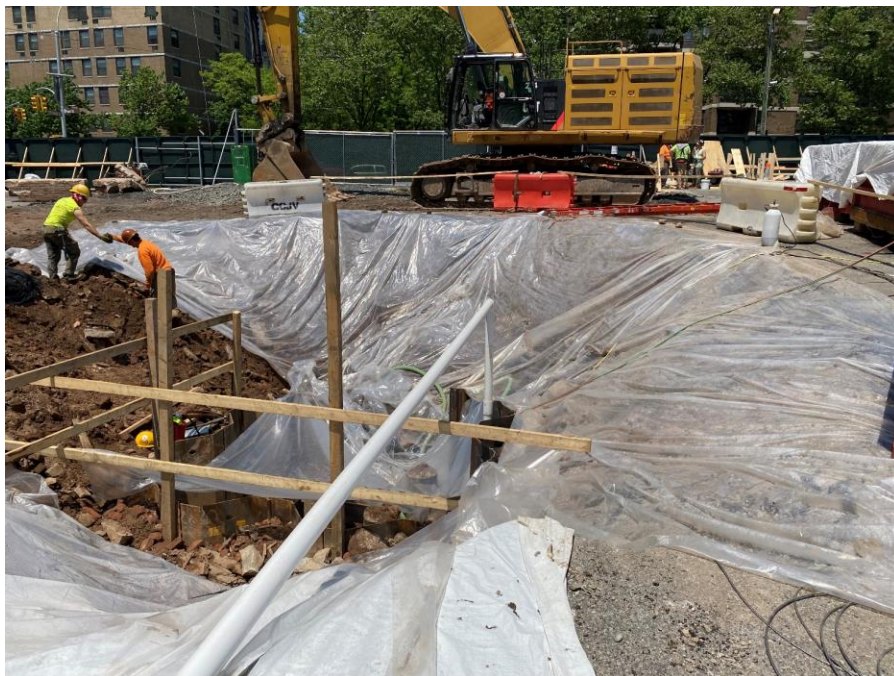
Photo 2: View of CCJV covering exposed soil/fill in the southwestern portion of the site (facing north).
