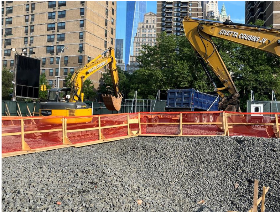
Photo 1: View of CCJV loading an excavator for demobilization off-site (facing north)
