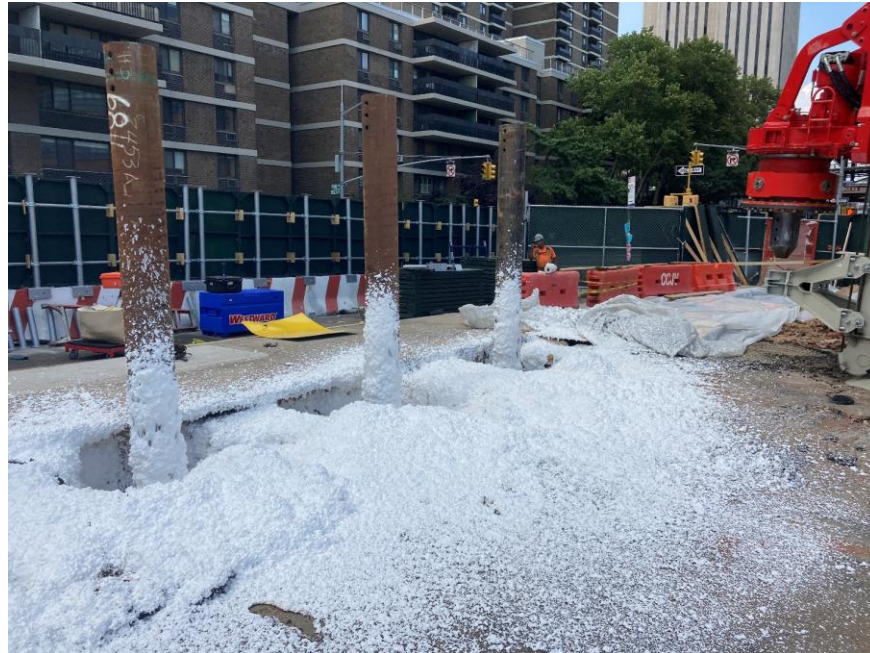
Photo 1: Atmos® AC-645 dust/vapor suppressing foam applied to areas of exposed soil/fill in the northern part of the site (facing northeast)
