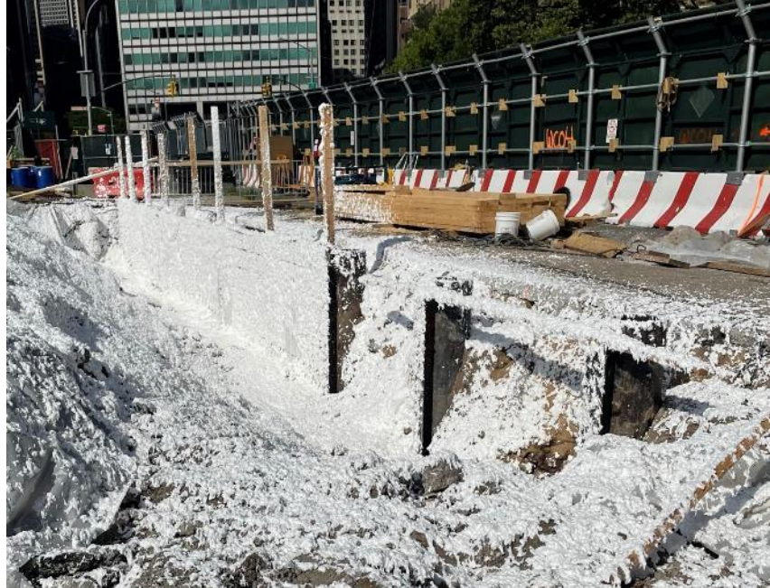
Photo 1: Atmos® AC-645 dust/vapor suppressing foam re-applied to exposed soil/fill along the northern boundary of the site (facing northwest).
