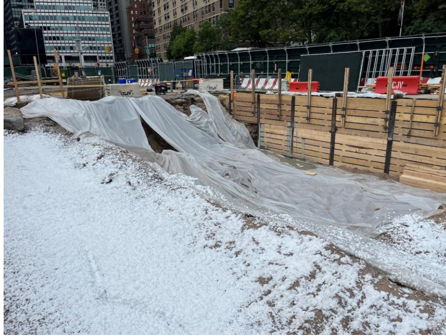
Photo 1: Atmos® AC-645 dust/vapor suppressing foam and/or polyethylene sheeting applied to exposed soil/fill in the north-central part of the site (facing northwest)
