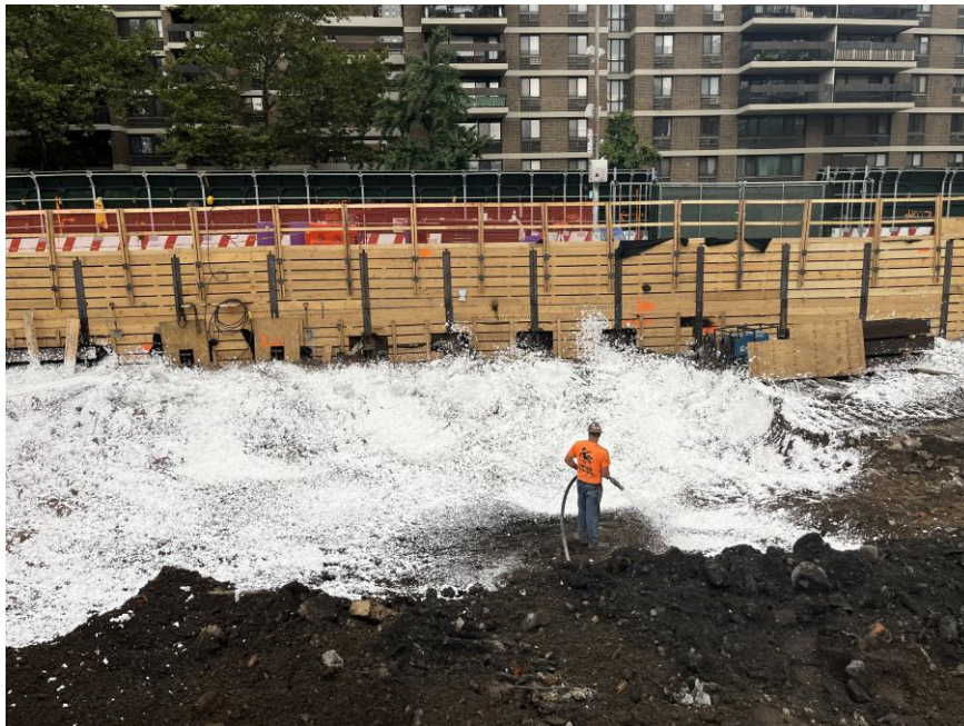
Photo 2: CCJV covering exposed soil/fill with Atmos® AC-645 dust/vapor suppressing foam (facing north)
