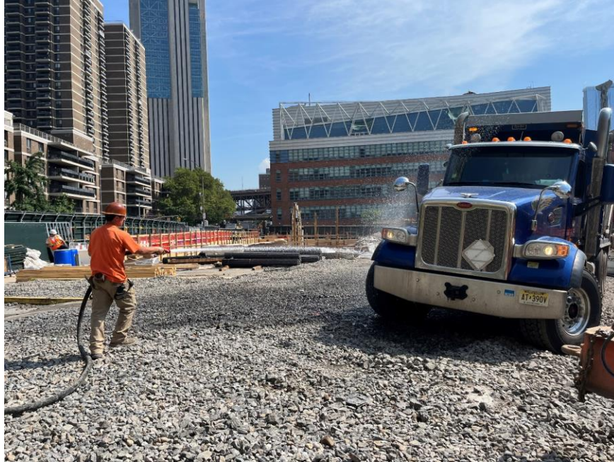
Photo 1: CCJV washing a dump truck prior to exiting the site (facing east)
