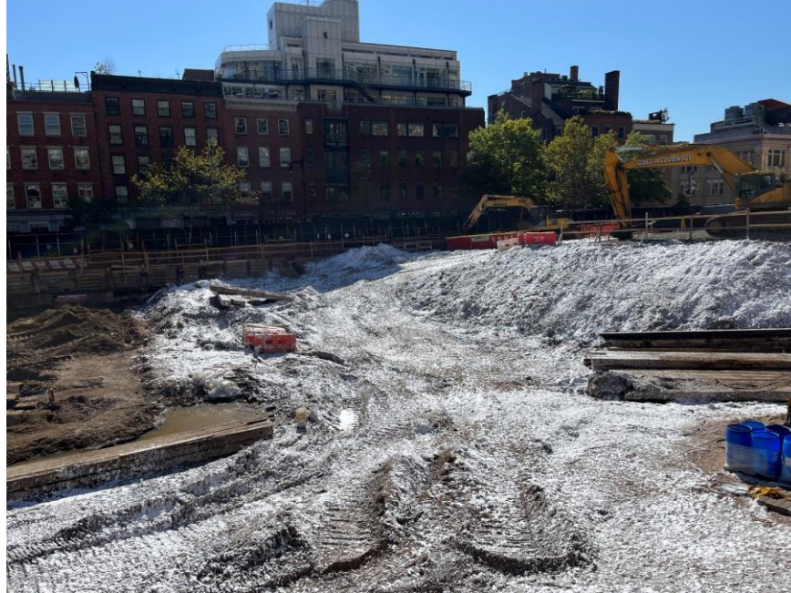
Photo 1: Atmos® AC-645 dust/vapor suppressing foam applied to exposed soil/fill for the temporary overnight cover (facing southwest)
