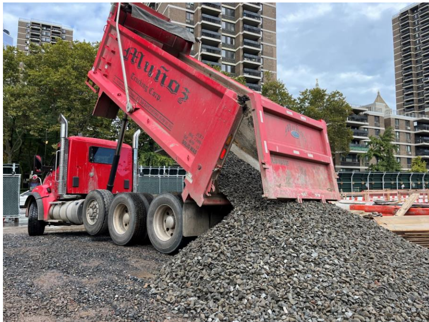
Photo 2: CCJV importing 1.5-inch clean bluestone for tracking pad maintenance (facing northeast)
