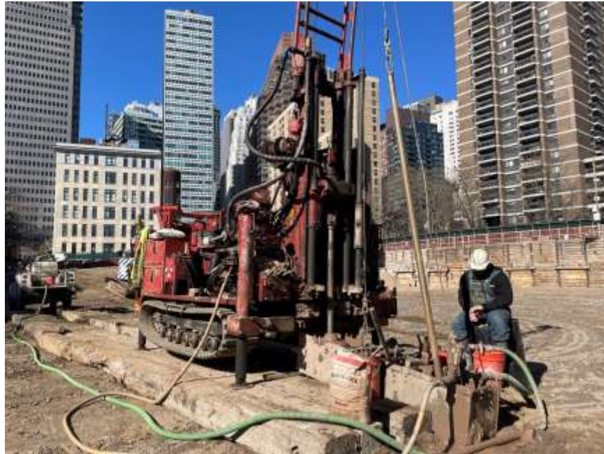
Photo 1: Craig advancing a geotechnical boring in the southeastern part of the site (facing northwest)
