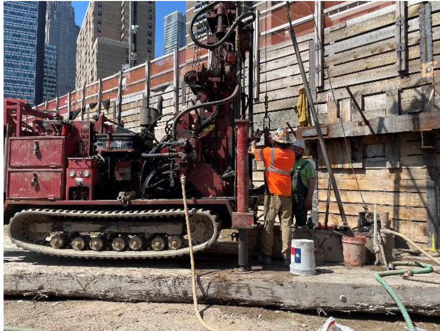
Photo 1: Craig advancing a geotechnical boring in the northern part of the site (facing northwest)
