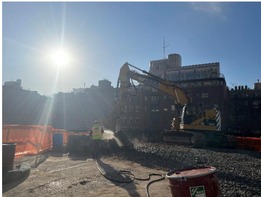
Photo 2: ECD spraying water across the site to mitigate dust generation (facing southeast)
