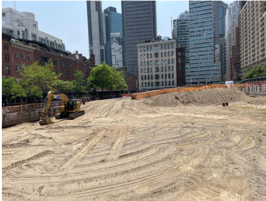
Photo 1: General view of the site (facing west)
