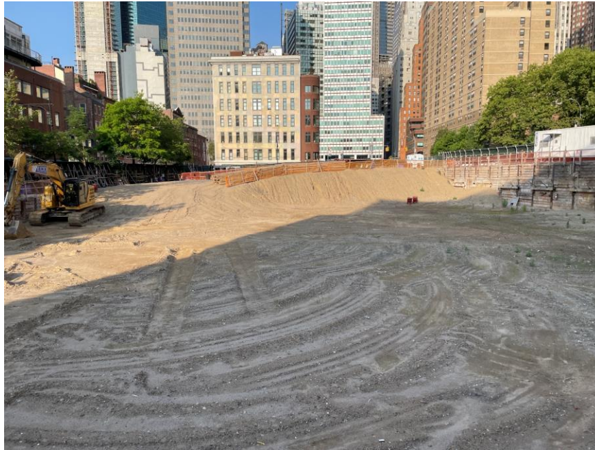
Photo 1: General view of the site (facing west)
